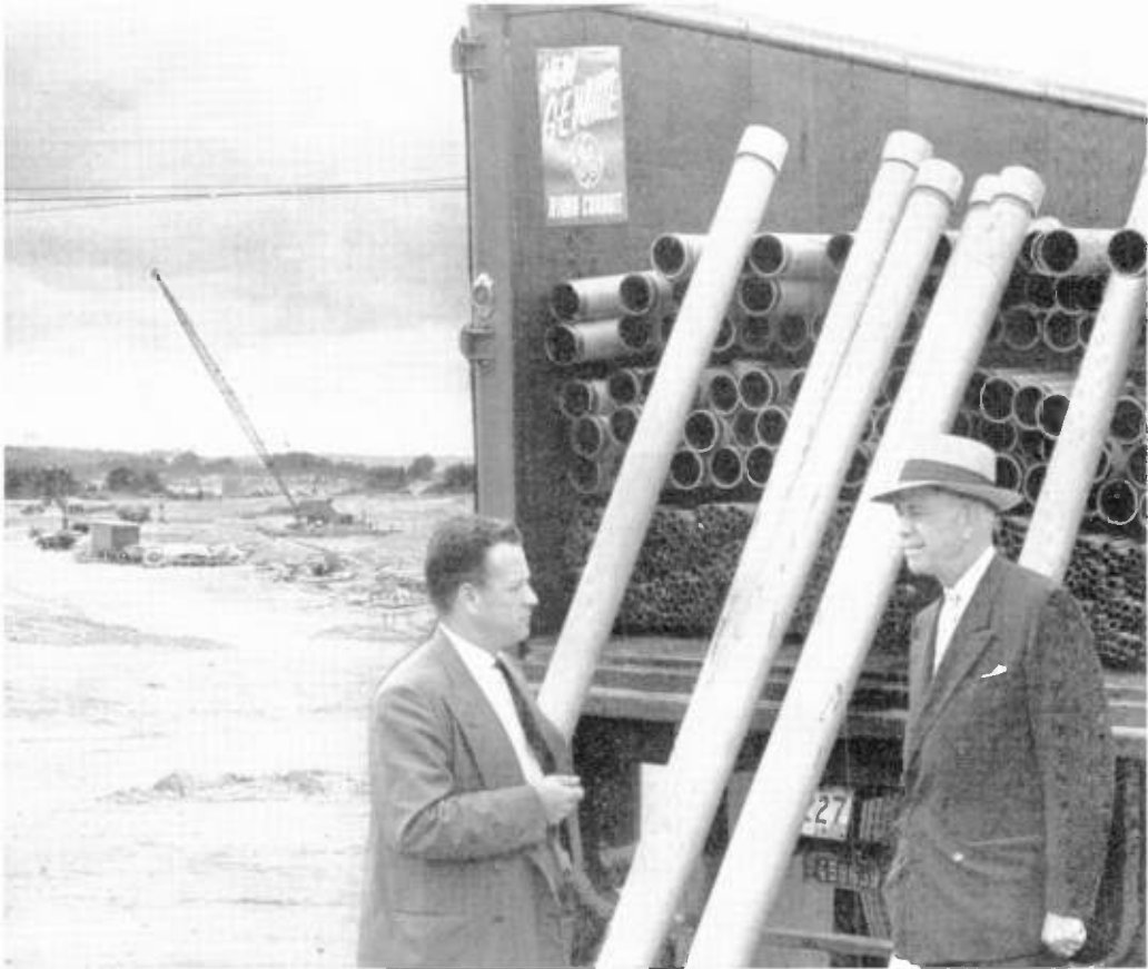
DOWNES OF SIKORSKY, MURRAY OF G.E. AND FIRST LOAD OF CONDUIT
