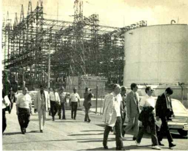
MSTGPD employees inspect their products on location at the South Coast Power facility in Ponce, Puerto Rico.
