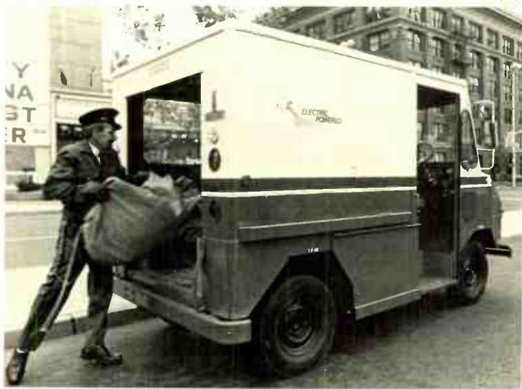
The Battronic electric Minivan is successfully covering a 90-stop-per-day mail route in Spokane, Washington. The GE powered and controlled vehicle uses less than 1¢ worth of recharging electricity per mile.
