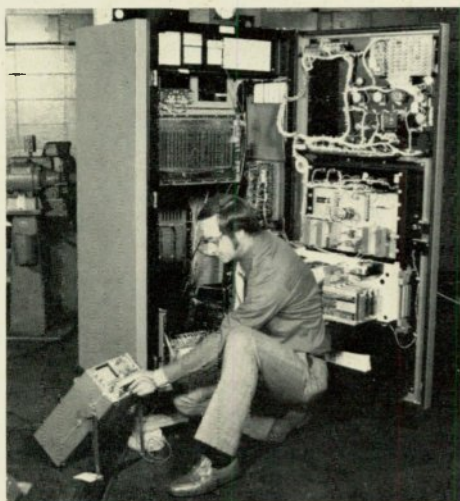
I&SE project manager (top) applies numerous technical skills to handle utility's electrical and electronic maintenance program. GE computer numerical control (above) is maintained by I&SE machine tool technicians.
