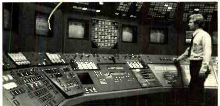
The first U.S. nuclear operator control system to use cathode-ray tubes as the primary data-display method—the GE Advanced Con-
