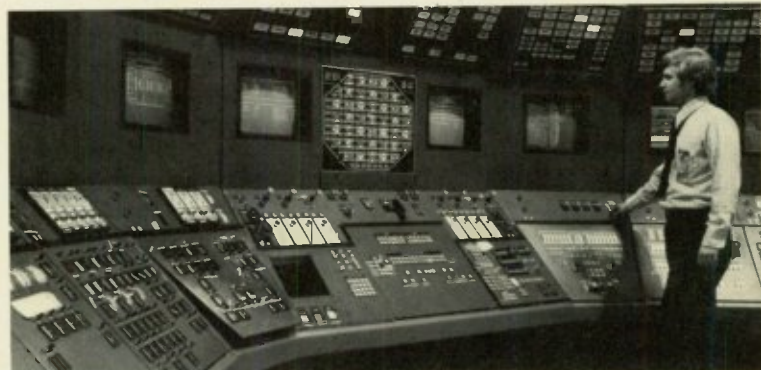
The first U.S. nuclear operator control system to use cathode-ray tubes as the primary data-display method—the GE Advanced Con-
