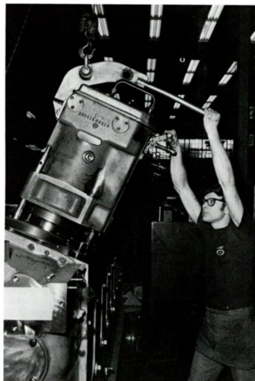
Some 5000 General Electric diesel engines are now in operation. In Erie's main assembly area, grinder Randy Strickenberger grinds an engine's main connecting rod, while assembler Rick Pheasant lowers unitized cylinder into place.
