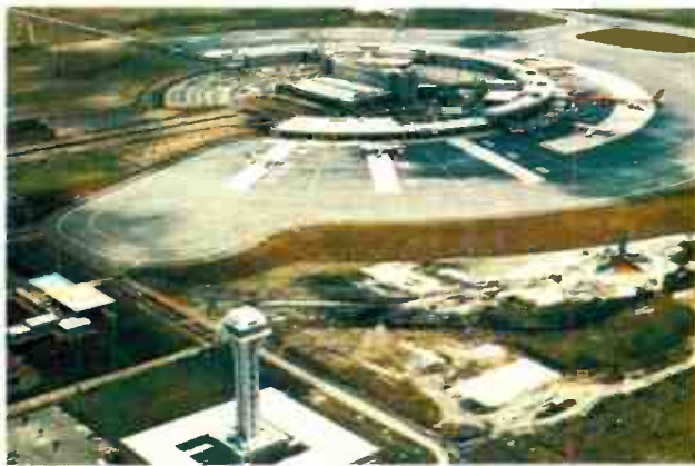
At Nairobi's airport, GE construction affiliate, Sadelmi, installed electrical/mechanical systems that operate control tower, runway lights and various air terminal services.
