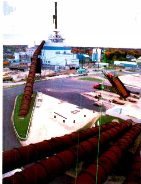
Cogeneration: In Maine, forest products unfit for paper are used to drive a GE steam turbine-generator.
