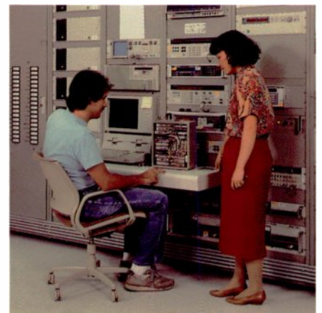
Minh Nguyen, project/design engineer (standing), and Dave Curulla, electrical repair & test, Seattle
