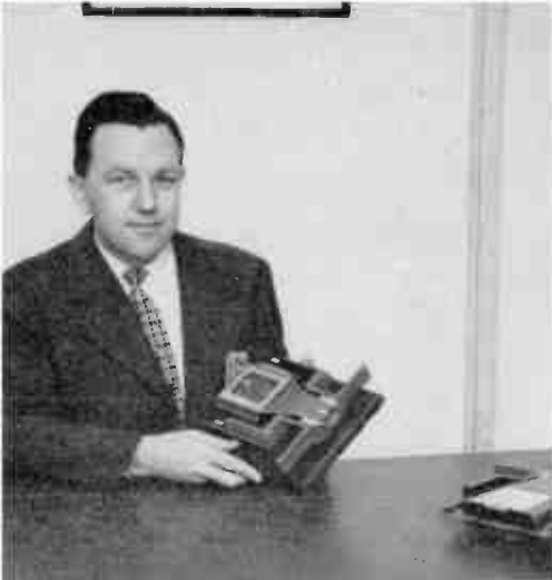
OBERLY —with electromagnetic sodium pump
