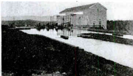
Fig. 5. Penstock Gates and Switch House
