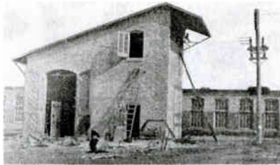
Fig. 6. Bessemer City Transformer Substation Built to Accommodate Multigap Lightning Arresters
