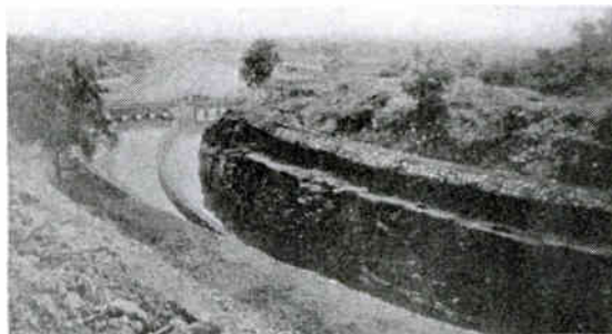
Fig. 4. Channels Through Rock Cutting
