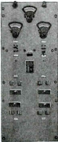
Fig. 11. Exciter Panel
