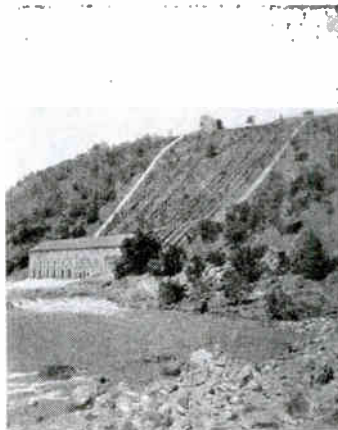
Fig. 6. General View of Development at Power House
