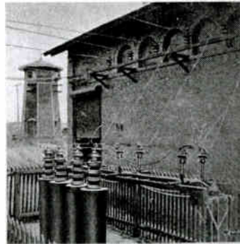
Fig. 7. Highland Park Substation, Charlotte, N. C., Showing Old Lightning Arrester Tower on left, O.E. Aluminum Cell Lightning Arrester and Horn Gaps in Foreground
