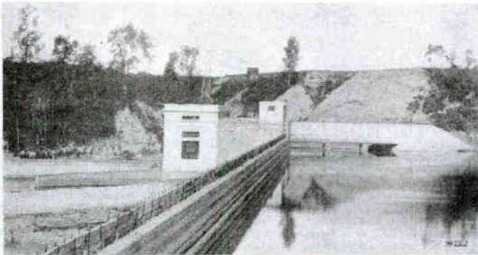
View looking down stream, showing dam equipped with flash boards and intake to forebay
