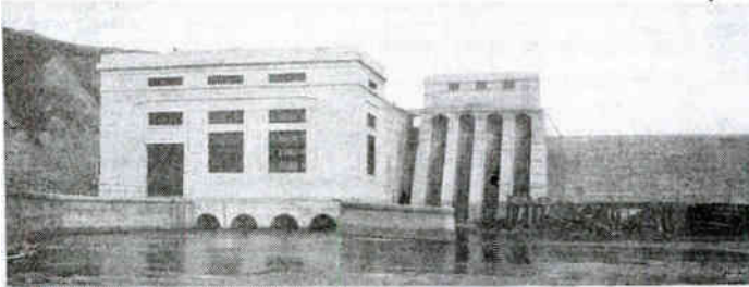
View looking up stream showing finished power house and sluice gate masonry
