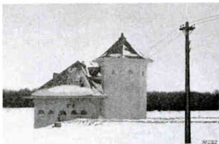
View of Tracy Brook Power House and Beginning of Direct Current Transmission Line
