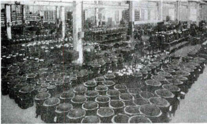
Fig. 11. Group of Small Transformers Completed and Ready for Test
