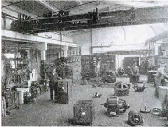
Transformer and Regulator Repairing and Testing. South Bay
