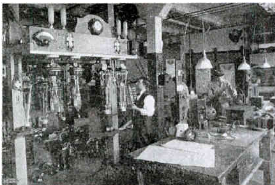
Arc Lamp and Fan Motor Repairing and Testing
