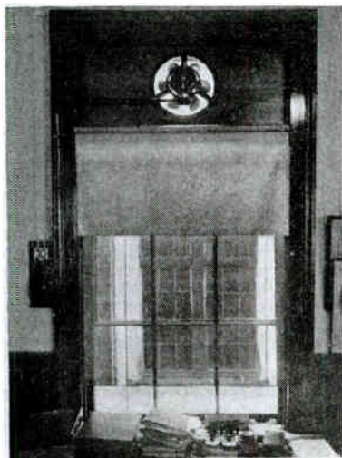
Installation of 12-Inch Alternating Current Ventilating Outfit
