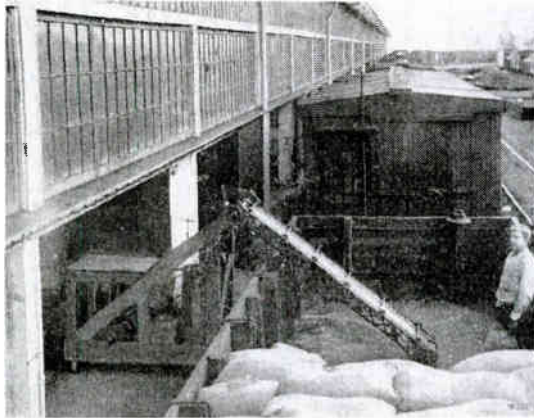
Fig. 4. Brown Portable Elevator for Unloading Gondola Cars
