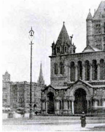
Fig. 4. Vertical Carbon Flame Arc Lamp, Copley Square, Boston
