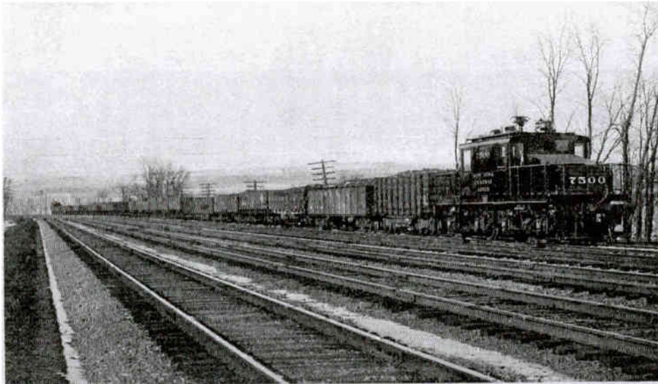
Detroit River Tunnel Electric Locomotive Hauling 1400 Ton Freight Train
