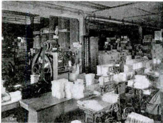
Fig. 2. General View of Fourth Floor
