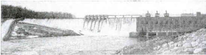
Dam, Power House and Grinder Station on the Penobscot River. Great Northern Paper Co., Dolby, Me.
