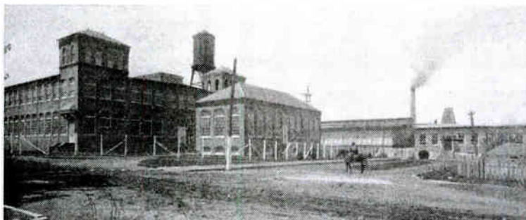
Fig. 6. Office and Substation, Proximity Mill
