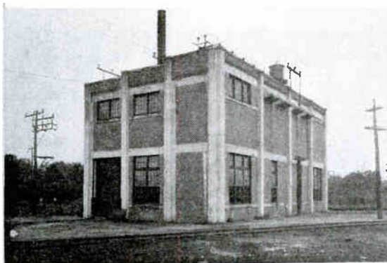
Fig. 9. Naval Academy Substation
