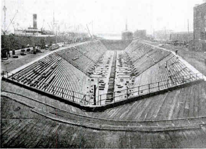
Fig. 1. Graving Type Dry Dock, Pumped Dry
