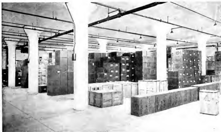
Fig. 3. Day View in a Warehouse Which Has an Excellent Illumination System. The rooms are divided into bays by columns on centers 20 by 20 ft. Each bay is provided with two outlets. Sixty-watt tungsten filament gas-filled Mazda lamps in deep bowl intensive aluminum finish reflectors are placed close to the 13 ft. ceiling. All wiring is in metal conduit and rows of lights are controlled by snap switches, which are located in the boxes shown on the columns in the foreground.
