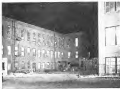
Fig. 66. Factory Yard Floodlighted for Protection
