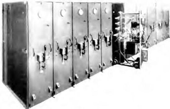
Fig. 51. Removable Truck Safety First Switchboard.
