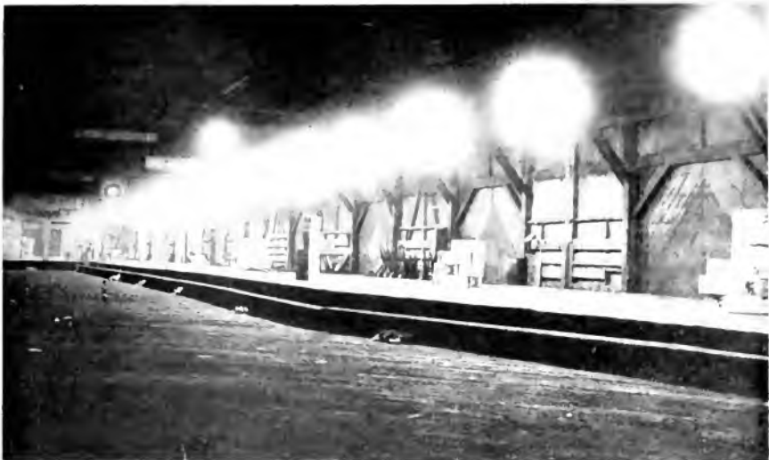
Fig. 5. Night View of the Delivery Platform of a Large Railroad Pier. This is illuminated by 200 watt, bowl-shaped tungsten filament gas-filled Mazda C lamps with dome-shaped enameled steel reflectors, hung well out of reach. Certainly trucking and freight handling can be carried on with expedience under such illumination.
