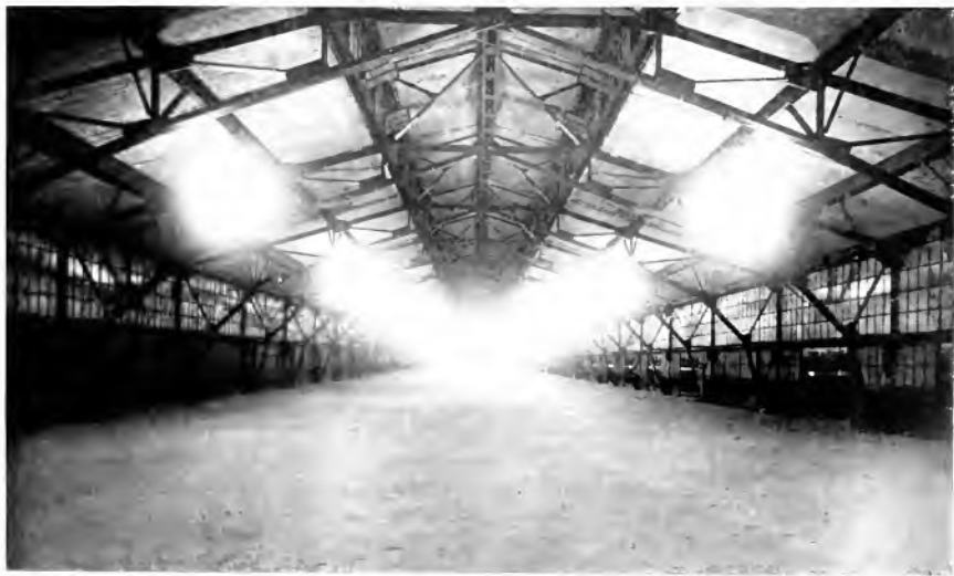
Fig. 6. Night View of the Passenger Section of the Chicago Municipal Pier. This is 2340 feet long. A total of 236,400 watt tungsten filament gas-filled Mazda C lamps in opalescent enclosing globes are hung 25 ft. high. These are on centers 40 by 35 ft. The freight section is located on the floor below. This is of equal dimension but with a somewhat lower ceiling. Similar equipment and spacing are installed.
