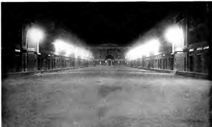
Fig. 8. On Account of the Density of Trucking and Traffic in the Neighborhood of a Pier, it is Desirable to Have Good Illumination for all Adjoining Areears. This night view, taken down the center of the Commonwealth Fish Pier, Boston, shows the effects of using 750-watt tungsten filament gas-filled Mazda C lamps in street lighting fixtures of the diffusing type. The lighting units are supported on brackets extending from the face of the building
