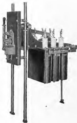
Fig. 42. Triple pole Type FK 32 A Oil Circuit Breaker
