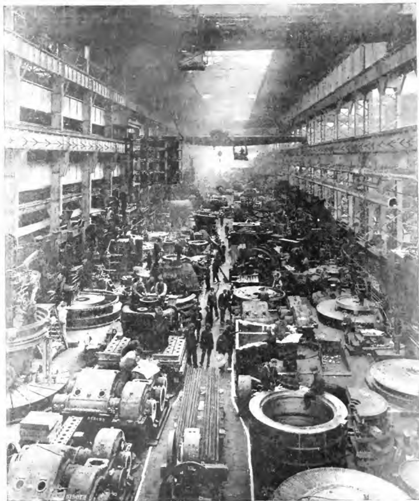
Assembly of Large Steam Turbine Generators, Schenectady Works, General Electric Company This view shows one bay of building No. 60 in which single-unit steam turbine generators ranging from 2500 to 50,000 kilowatts in capacity are assembled and tested
