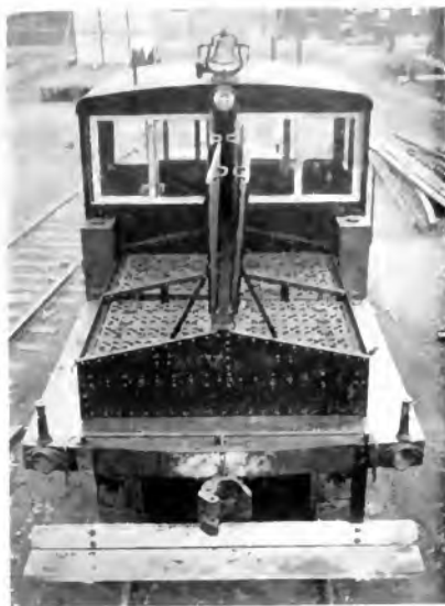
Fig. 17. Arrangement of Storage Batteries on 20-ton Locomotive
