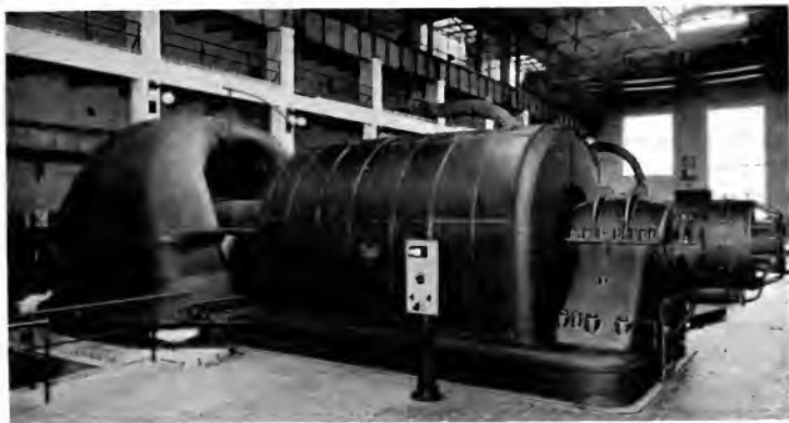
Fig. 1. 45,000-kw., 50,000 kv-a. Curtis Steam Turbo generator
