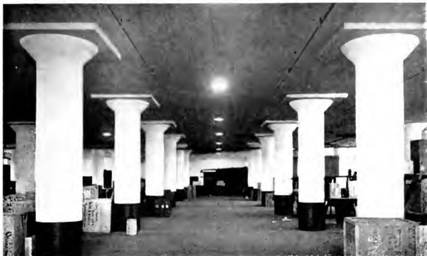
Fig. 2 Splendidly Illuminated Warehouse of Modern Construction. One 200 watt tungsten filament gas-filled Mazda C lamp in enameled dome reflector is placed close to the 15 ft. ceiling in each 20 ft. bay.
