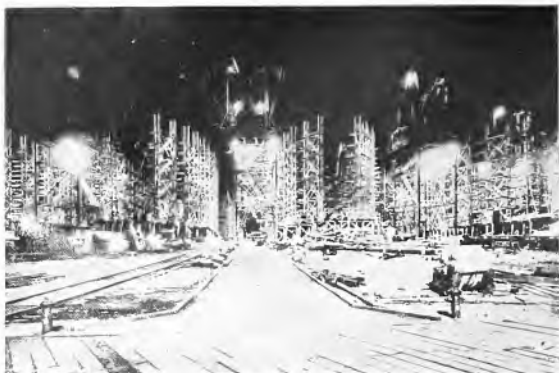
Fig. 68. Illumination of Hog Island Shipbuilding Yard by Floodlighting Projectors
