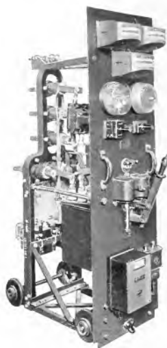
Fig. 53. Removable Truck Panel, Triple pole, Single-throw, 500 Amps., 2300 Volts
