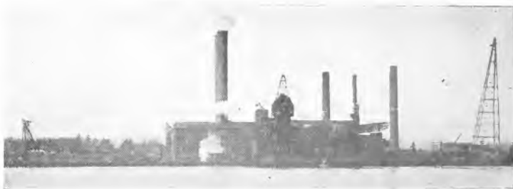
Fig. 23. General View of Power Station and Coal Handling Equipment of the Baltimore Consolidated Gas, Electric Light & Power Co.
