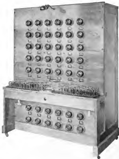
Fig. 6. Front of Improved Calculating Table Built for a Large Power Company
