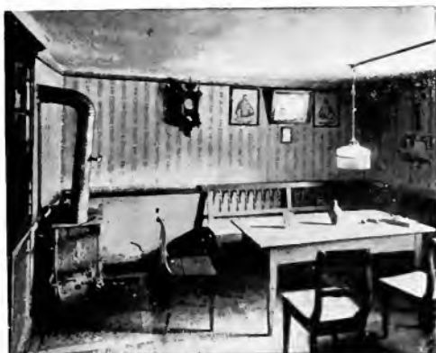
Fig. 2-b. Another example of electric lighting in a peasant's home. Whether good or bad lighting is sold depends almost entirely upon the one who sells the fixtures. Neither of the fixtures in Figs. 2-a and 2-b screens the lamp from view. The one in Fig. 2-a is no better from a glare standpoint than a bare lamp, and it could have been made much better at no greater cost.
