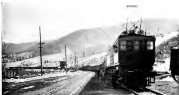
Chicago, Milwaukee & St. Paul 3000 volt Direct-current Electrification. Freight train, 1450 tons, west bound at Donald Summit of the Rocky Mountain Divide
