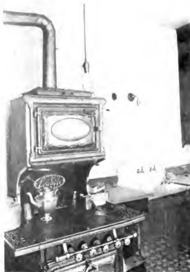
Fig. 15. Two outlets have been provided in this kitchen and if these were properly used good lighting would result. The cord above the stove should be considerably shortened, and both lamps should be fitted with good reflectors of opal glass, prismatic glass, or enameled steel.
