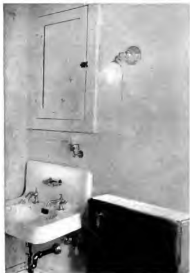
Fig. 11-a. Sometimes a marked improvement in lighting can be accomplished very simply. This illustration is typical of such an instance; the fixture as shown creates an objectionable glare. Compare with Fig. 11 b
