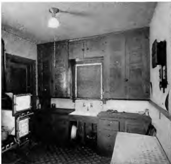
Fig. 8. The kitchen is the workroom of the home, and the lighting should be planned primarily for utility. The installation shown is above the average, but a person working at the sink or drainboards is handicapped by his own shadow. Since this photograph was taken, a supplementary lamp and reflector have been installed just beneath the middle cupboard
