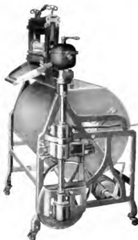
Fig. 4. Another cylinder type of motor-driven washing machine
