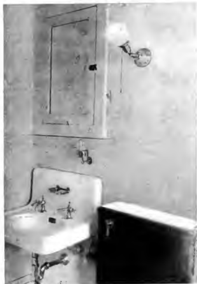
Fig. 11 b. The lighting fixture of Fig. 11-a is here shown turned upward and the frosted shade replaced by a prismatic reflector which reduces the glare and throws the major part of the light to the ceiling which in turn diffuses it completely
