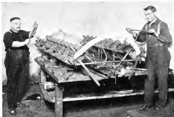
Fig. 14. Moulding the Turbine-generator Stator Coils in a steam mould before applying the external insulation
