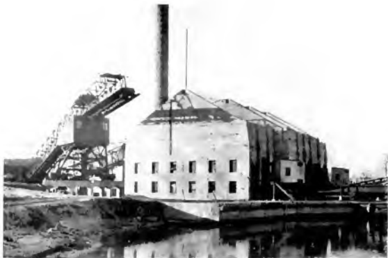
Fig. 21. Radial Incline Conveyor and Balancing Bin B & O Coal Loading Pier, Curtis Bay, Md.
