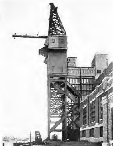
Fig. 17. Coal Tower Essex Station, Public Service Electric Company, Newark, N. J., 1½-Ton Bucket. Bucket Speed 1230 ft. per Minute
