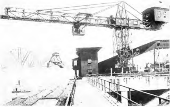
Fig. 14. Hammer Head Tower Coal Hoist at LaBelle Iron Works, Follansbee, W. Va.
