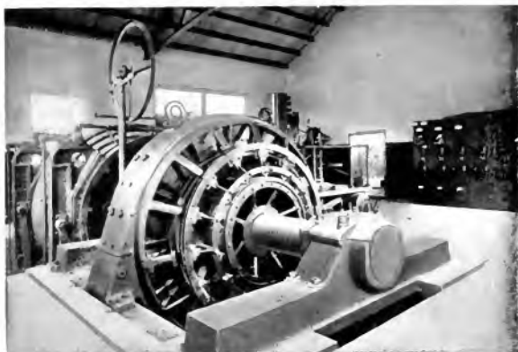
Fig. 14. 1400-h.p., 90-r.p.m., D.c. Motor Driving Cylindro conical Drum Hoist at Consolidation Coal Co., Fairmont, W. Va., Flywheel Motor-generator set installed in adjoining room
