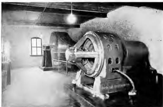
Fig. 2. 250-h.p. Induction Motor Belted to Mine Fan
