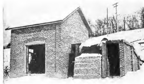
Fig. 5. Fan House Containing 100-h.p. Motor (Fig. 4) and 100,000-cu. ft. Fan.
