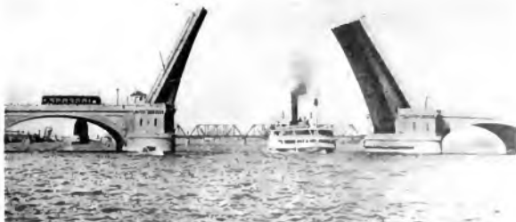
Fig. 8. Scherzer Double Leaf Bascule Bridge in Open Position
