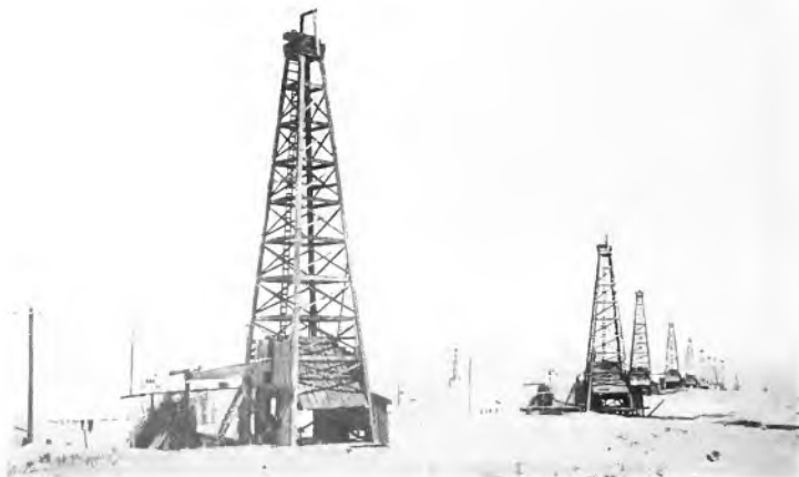
Fig. 20. This Group of Wells in the California Midway Field Has Been Electrically Operated for Several Years by the Fuel Oil Dept. of the Southern Pacific R.R.
