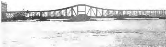
Fig. 2. Swing Span Bridge in Closed Position
