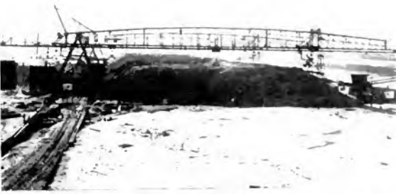
Fig. 4. Three Rope Operated Coal Bridges at Berwind Fuel Company's Dock Superior, Wis.
