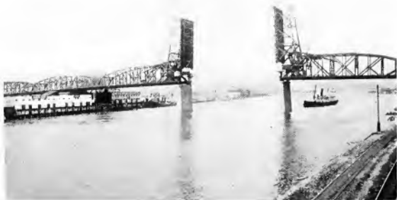
Fig. 13. Rall Double Leaf Bascule Bridge in Open Position
