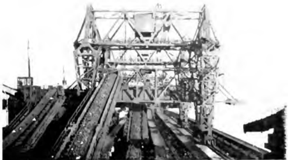
Fig. 24. One of the Four Transverse Bridges Showing Location and Operation of Main Conveyor Belts, B. & O. Coal Loading Pier, Curtis Bay, Md.
