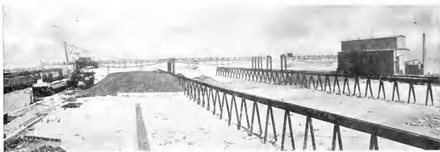
Fig. 5. Coal Bridge Equipments Installed at Pittsburgh Coal Dock & Wharf Co.'s Dock, No. 7, at Rice's Point
