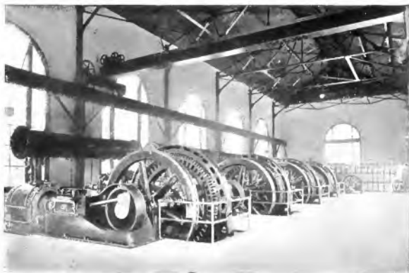
Fig. 3. Reciprocating Air Compressors Driven by Synchronous Motors
