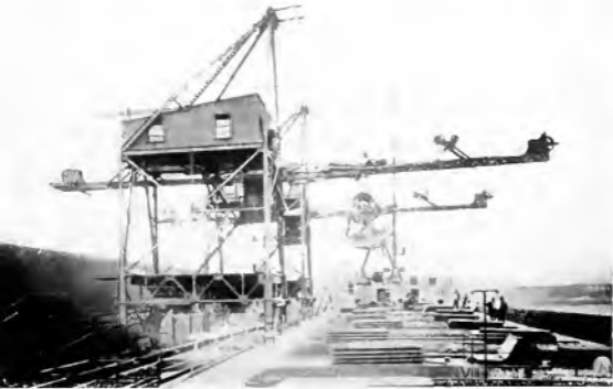
Fig. 16. Towers for Hoisting Limestone at the D. M. & N. Docks, West Duluth, Minn.
