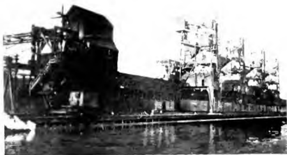
Fig. 3. The First Electrically driven Coal Unloading Dock Built in 1901 for Northwestern Fuel Company, Superior, Wis.
