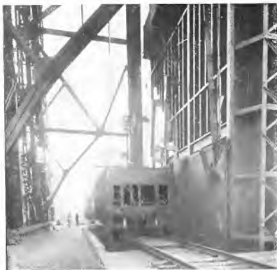
Fig. 11. Car Dumper Showing Cradle in Lowest Position with Car in Place Ready for Hoisting
