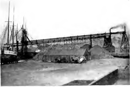
Fig. 2. Three Bridge Tramways Built for the New York, Lake Erie & Western Railroad Company, Cleveland, Ohio, in 1883
