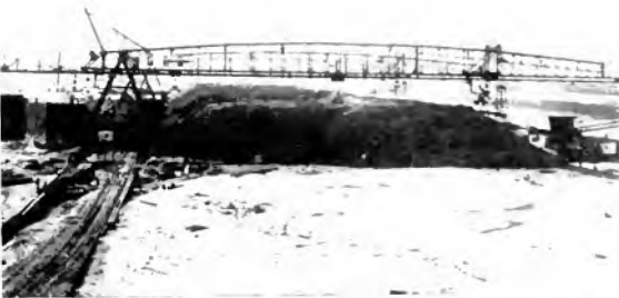
Fig. 4. Three Rope Operated Coal Bridges at Berwind Fuel Company's Dock Superior, Wis.
