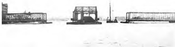
Fig. 3. Swing Span Bridge in Open Position
