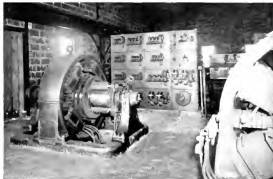
Fig. 10. 325-kw. Synchronous Converter Used to Control 1400-h.p. 21-in. Structural Mill Motor
