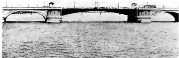
Fig. 7. Scherzer Double Leaf Bascule Bridge in Closed Position
