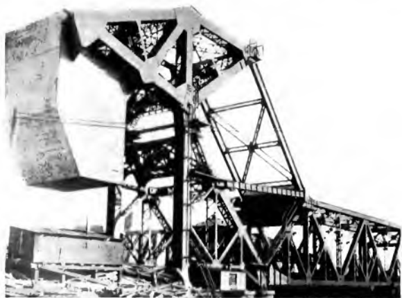
Fig. 9. Strauss Single Leaf Bascule Bridge in Closed Position
