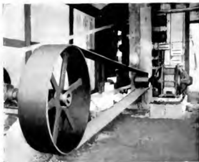
Fig. 14. Fifty-hp. Oil Well Drilling Motor Operating Standard Cable-tools at Well No. 3, Midway Pacific Oil Co., Fellows, Calif.
