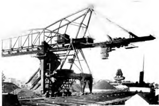
Fig. 7. Pier End of C. Reiss Coal Company's Coal Bridge at Manitowoc, Wis., Showing Electrically-driven Screening Plant
