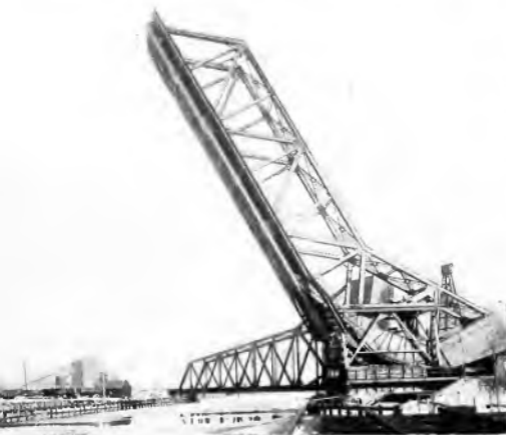
Two Single Leaf Scherzer Bascule Bridges. One Open and the Other Closed
