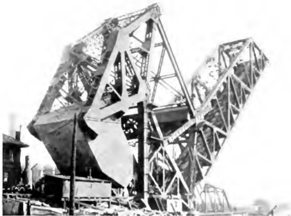
Fig. 10. Strauss Single Leaf Bascule Bridge in Open Position
