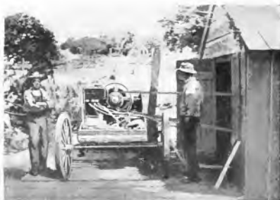
Fig. 9 Twenty-h p. Portable Motor Equipment for Pulling Oil Wells at the Badger Oil Co., Hosston, La.
