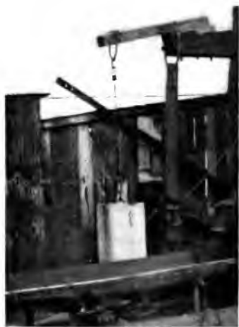
Fig. 13. This Concrete Counterbalance Was First Used by the Cosden Oil & Gas Co. at Shamrock, Okla., and is Considered the Most Effective Design Now in Use
