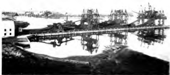
Fig. 22. General View of B. & O. Coal Loading Pier, Curtis Bay, Md.
