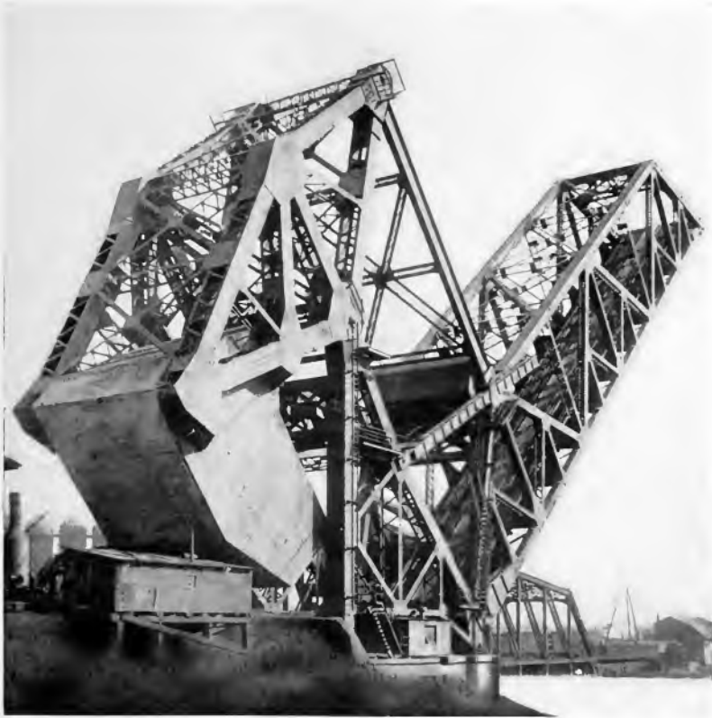
STRAUSS SINGLE LEAF BASCULE BRIDGE IN OPEN POSITION (See article, page 373)
