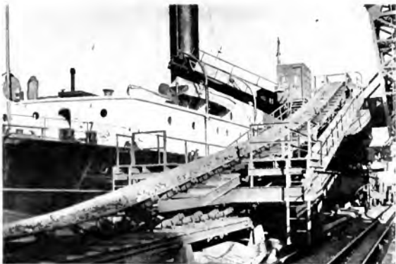
Fig. 23. Trimmer Conveyor Tower Showing Projecting Loading Boom and Conveyor Belt, B & O Coal Loading Pier, Curtis Bay, Md.
