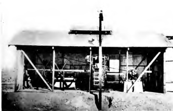
Fig. 4. A 30 15-h.p., Two-speed Oil Well Motor Showing General Arrangement Used by the Associated Oil Co., in the California Fields
