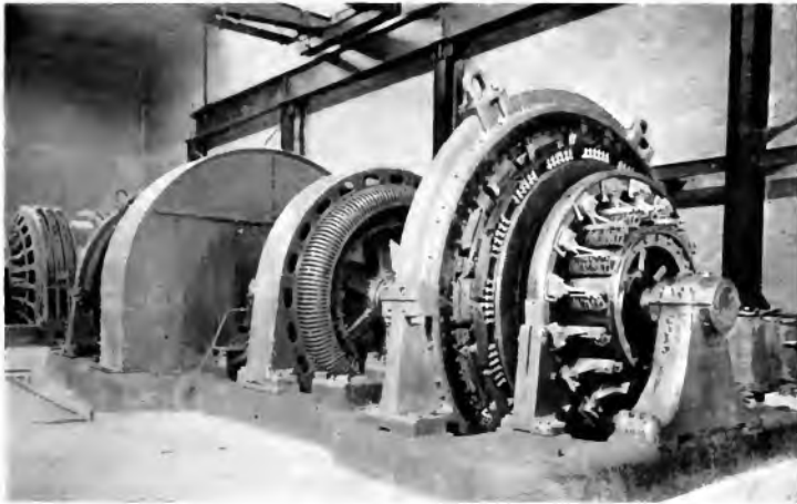
Fig. 20. Motor Room Showing 5000-h p., Reversing Mill Motor and 4000-kw., 3-Unit Flywheel Motor Generator Set for Driving Reversing Blooming Mill
