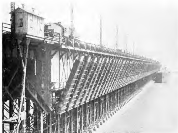
Fig. 19. Ore Dock No. 2, Duluth & Iron Range R. R., Two Harbors, Minn. The spouts are lifted by electric motors
