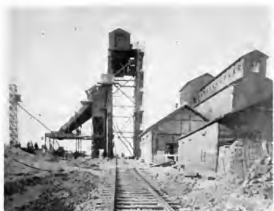
Fig. 25. General View of High Lift Car Dumper Installed at Semet Solvay Coke Plant, Indiana Harbor, Ind.
