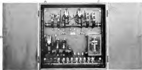
Fig. 9. Reversing Contactor Panel for Use on Plater Drive
