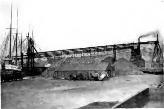
Fig. 2. Three Bridge Tramways Built for the New York, Lake Erie & Western Railroad Company, Cleveland, Ohio, in 1883
