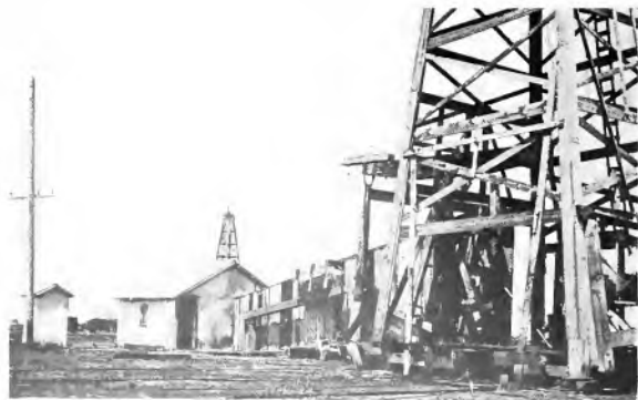
Fig. 12. The Type of Counterbalance on This Motor-driven Well of the Empire Gas & Fuel Co. in the El Derado, Field, Kansas, is Frequently Employed
