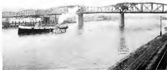
Fig. 14. Rall Double Leaf Bascule Bridge in Closed Position
