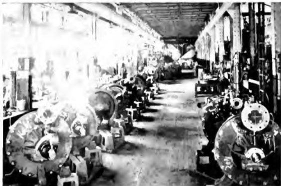
Fig. 9. Floor upon which are assembled the turbines described in this article
