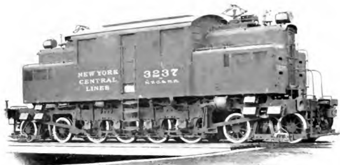
Fig. 1. 115-ton Gearless Bipolar Locomotive. Forty-seven of this original type of locomotive were furnished to the New York Central Railroad for hauling passenger trains out of the New York Central Terminal
