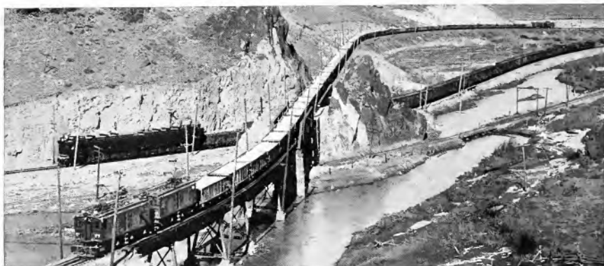
Fig. 4. Electric Trains on the Butte, Anaconda & Pacific Railway and on the Chicago, Milwaukee & St. Paul Railway Hauled by 2400-volt and 3000-volt Direct-current Locomotives
