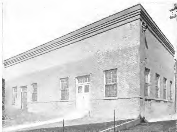
Fig. 7. New Main Substation, Cudahy Packing Co., Omaha, Neb.
