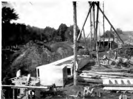
Fig. 3. Start of the Work Looking up the river towards Lock No. 6
