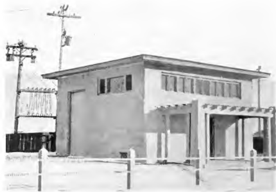
Fig. 1. An Attractive Housing for the Automatic Substation at Butte, Mont.
