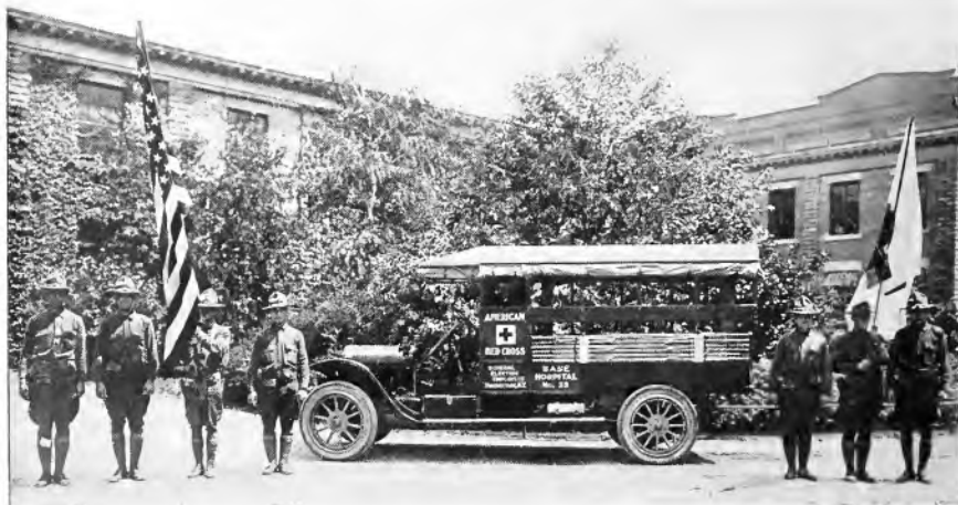
Fig. 2. Ambulance Presented to Base Hospital No. 33 by Schenectady Employees of General Electric Company
