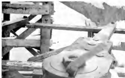
Fig. 6. One of the Sixteen Ratchet Wrenches which were Operated in Unison
