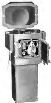
Fig. 4 Single-phase Automatic 2300-volt Pole-type Regulator
