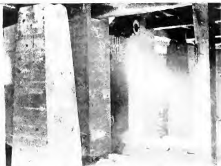
Fig. 3. Foundation of Turbo-generator, Bakery Power House, Is-Sur-Tille . Water level made a basement impossible and the generating unit had to be elevated
