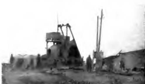
Fig. 18. Boche Concrete Mixing Plant, Slip-ring Motor Driven with Transformer Station. This was near Charey, on the Hindenburg Line, in the Toul Sector. The Germans had several of their plants on hills with extensive narrow-gauge railroads running down to the massive monolithic concrete dugouts on the Hindenburg Line
