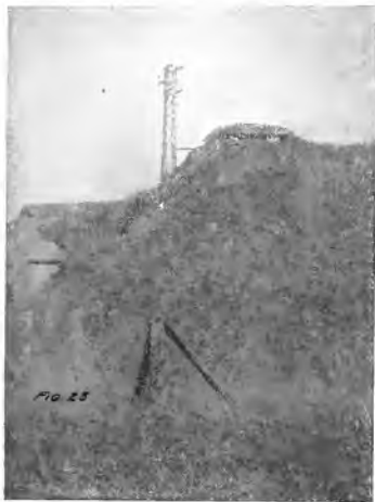
Fig. 23. Boche Observation Station in Former City Water Works. The Germans held this point until the armistice. They watched the French forts before Verdun from here. Note how little the ground is changed as seen from above by an airplane, by the addition of this post. The slot in front was faced with heavy plate glass and shielded from sunlight by a metal hood covered with earth.
