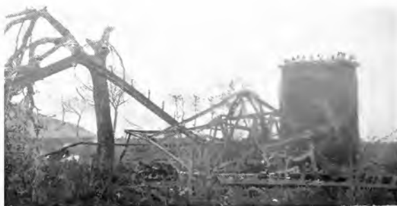
Fig. 30. Wreck of German 17000 3000-volt Transformer Substation Just Outside of Vignuelles, showing the condition in which the Boche abandoned it. One 17,000-volt line ran from here toward Montsec and another toward St. Mihel. Four 3000-volt lines went out of this station to about ten transformer stations of 10 and 15 kv-a. The oil switches and iron framework are completely destroyed
