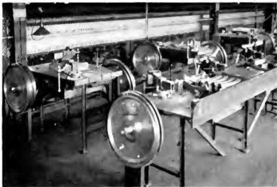
Fig. 9. Manufacture of Bucket Wheels and Intermediates.
