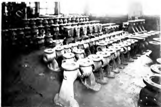
Fig. 15. Governor Valves. Short-arc type in front, long-arc in rear, and emergency valve in center
