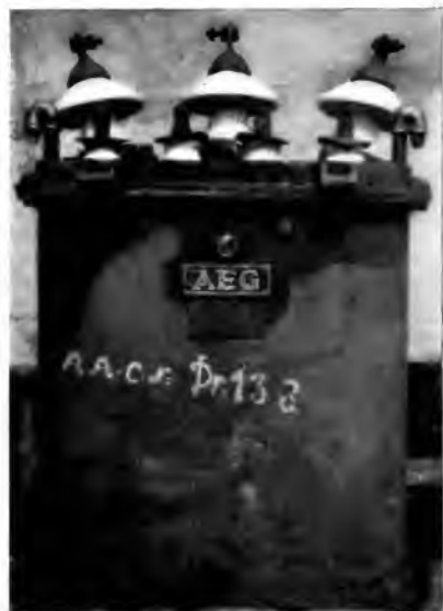
Fig. 14. Captured Boche Transformer. 7.5 kv.-a., Three-phase, 50 cycles, 3000-2700-218 volts, four-wire
