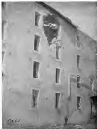
Fig. 20. Part of the East Face of the Old Mill at St. Mihiel, shown in Fig. 19. The Army 220-volt supply cables can be seen coming out of a window and running down the wall into the tailrace, in which they went under the railroad tracks.
