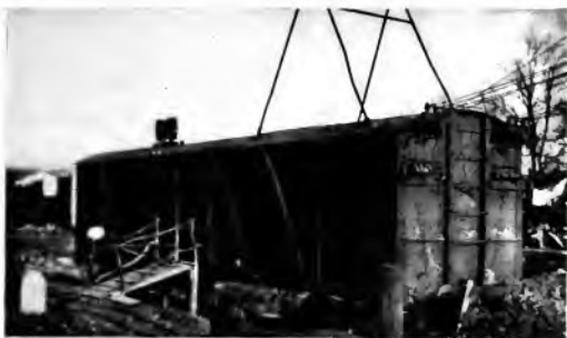
Fig. 22. 50-kw. Gasoline Engine Electric Plant in American Box Car in Freight Yard at St. Mihiel. This is the type of freight car in which hundreds of thousands of American soldiers rode back and forth across France and which was also used to supply them with rations, clothing, etc.
