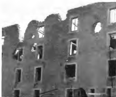
Fig. 19. Part of the Main Building of the Before-the-war Large Grist Mill and Electric Control Station on the Left (west) Bank of the Meuse River at St. Mihiel. The Army electrical plant was on the ground floor of this ruin and the control of speed was by a handwheel among the debris on the floor above. Most of the floors were gone as well as the roof and windows.
