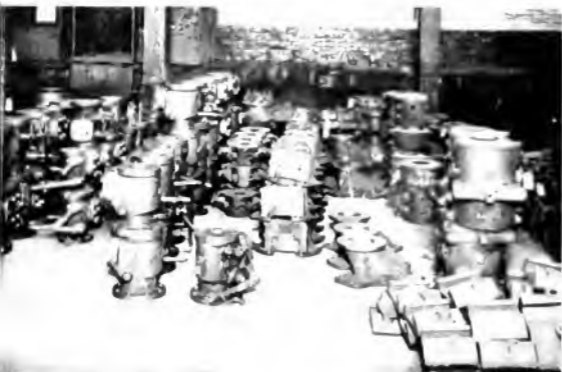
Fig. 18. Emergency Governor Valves
