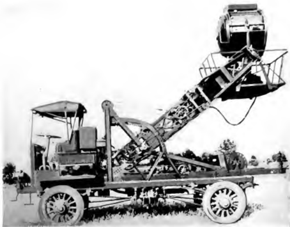
Fig. 3. 36-in. Carlisle & Finch Searchlight Mounted on Strauss Tower — Tower partly raised
