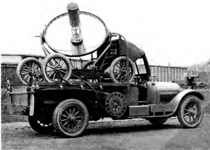
1918 Model, 60-inch Size, Mobile Searchlight Equipment
