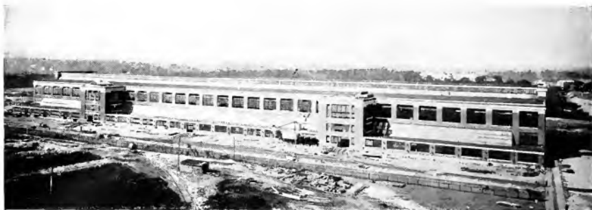
Exterior View of Building No. 5 at Eric
