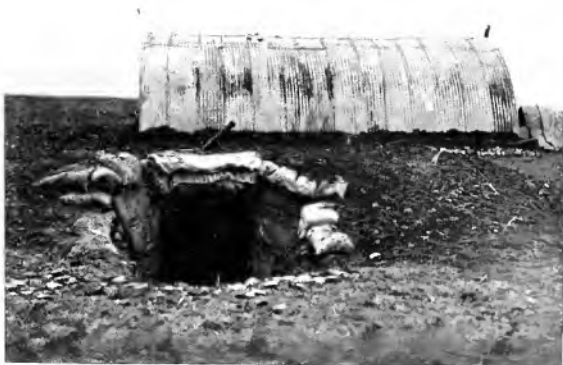
Fig. 4. Dugout for Searchlight Stationary Power Plant and Quarters
