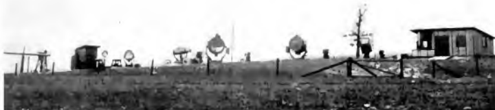
Fig. 2. General View of Searchlight Station. From left to right, there are shown: 1. 6 in. telephotometer tube, 2. lens of 15 in. telephotometer on pier, 3. sectored disc housing, 4. wireless telephone house, 5. 15 in. incandescent projector, 6. 30 in. incandescent projector, 7. 60 in. medium intensity open type projector, 8. 60-in. high intensity projector, 9. mast of wireless telephone, 10. 60 in. low intensity projector (in high intensity drum), 11. 60 in. high intensity projector, 12. test house.
