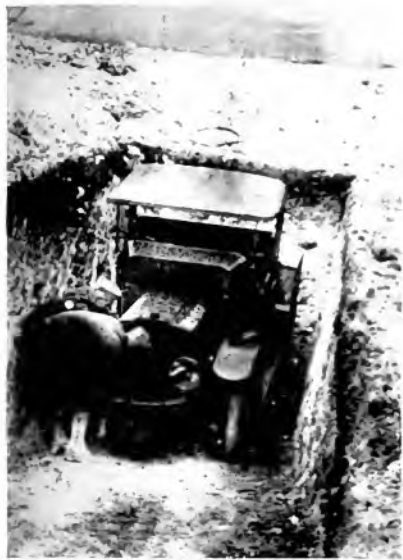
Fig. 7. Searchlight Power Plant Emplacement
