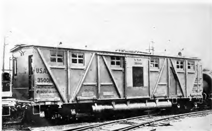
Fig. 6. 60-inch Seacoast Railway Tower Type Searchlight. Side View of Box Car (Power Unit) showing One of the 320-gallon Gasolene Tanks Suspended
