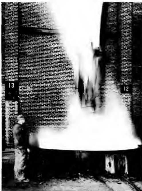
View showing gun being quenched after removal from electric furnace
