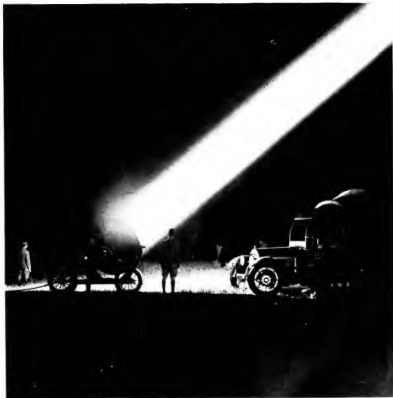
Night View of the New Open type 60 inch High-intensity Searchlight and Its 20-kw. Mobile Power Unit in Position to Ward Off an Airplane Raid
