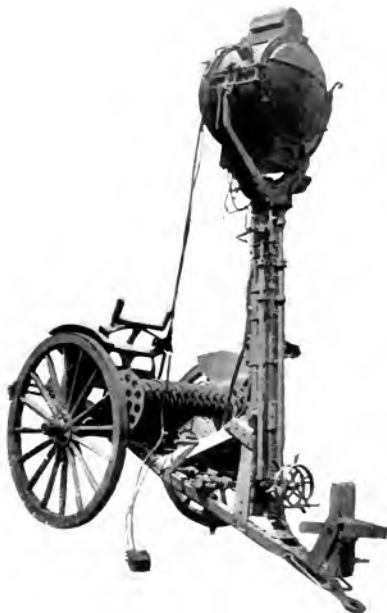
Fig. 1. 24-in. Sperry-Brill Caisson Tower Type Searchlight
