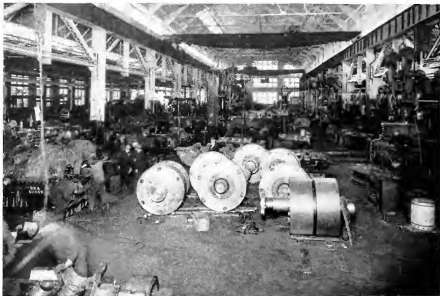
View of the interior of Building No. 49 at the Schenectady Plant. Before the war this was an iron foundry. To meet the war emergency for producing turbines and gears for ship propulsion, this building was enlarged and equipped with machine tools, etc.
