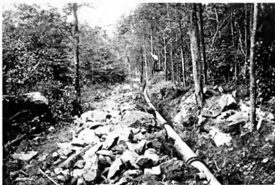
Fig. 16. Typical Natural Gas Main Line Construction Conditions
