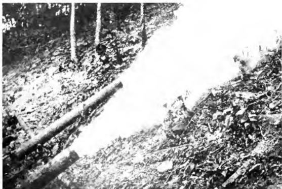
Fig. 13. Two 4-in. Pipes Wasting 5,000,000 Cu. Ft. of Natural Gas in Order to Get Oil
