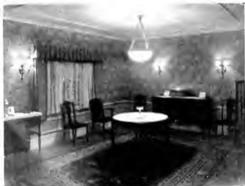
Fig. 8. View of the Dining Room with a Semi-indirect Unit Installed. This is supplemented by a number of attractive wall brackets. The cooking device and the electric fountain will be noted on the serving table and buffet respectively.
