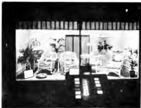
Fig. 11 - View of the Full Size Display Window with the High Intensity Uniform Lighting Turned On. Every detail of the display is clearly revealed. The control table for manipulating the intensity of the lighting automatically is visible in the inner hall foreground.
