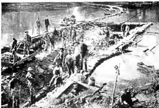
Fig. 15. Natural Gas Main Line River Crossing Under Construction
