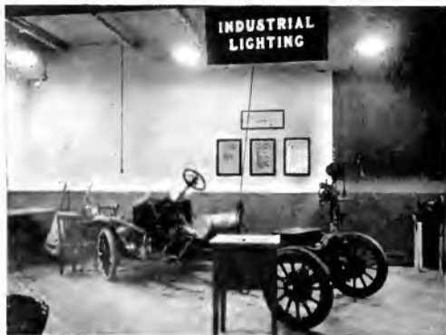
Fig. 3. View of the Industrial Exhibit with the "Good" Lighting System Turned On. This is designed to produce productive intensity. There is an absence of direct and reflected glare. Such shadows as are produced are soft and luminous. There is a high intensity of illumination on the work in both the horizontal and vertical planes.
