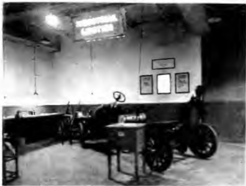
Fig. 3. View of the Industrial Exhibit with the "Fau" Lighting System. A slight intensity of general illumination is provided, supplemented by properly shielded local lamps. The distribution of light is not very even. There is considerable reflected glare and poor illumination in vertical surfaces.
