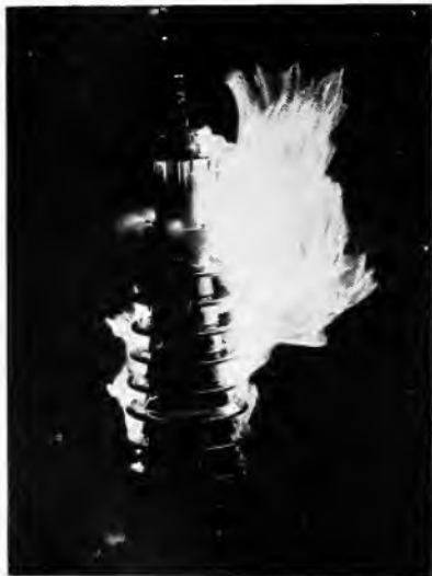
Fig. 6. Dry Flashover of Filled Type Flange Clamped Porcelain Bushing at 395,000 Volts
