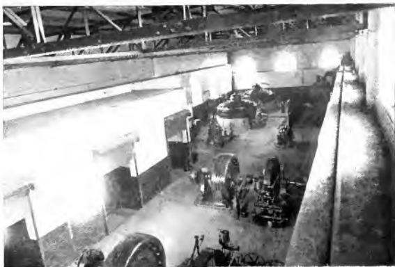
Fig. 3. Gardner's Falls Station; Greenfield Electric Light & Power Co.
