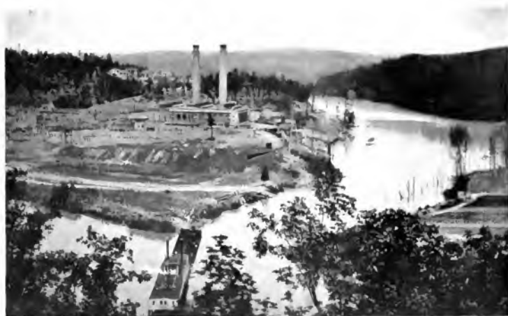
Fig. 1. General View of the Warrior Steam Plant. 110 kv and 44 kv. Switching Yard
