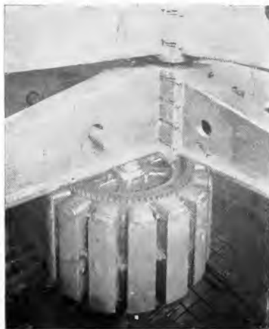
Fig. 5. Rotor of Waterwheel-driven Generator in Testing Pit
