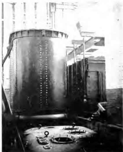
Fig. 6. Tanking Transformer Core with Special Lifting Device
