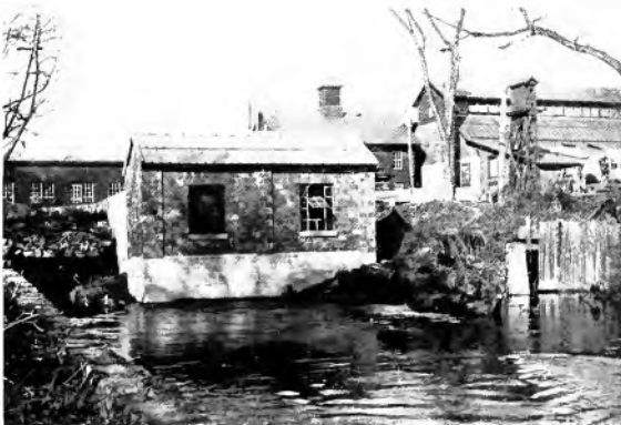
Fig. 6. The discharge of the draft tube is on the side away from the flume. The wires are shown which "collect" the power and feed it into the system.
