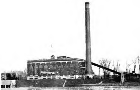
Fig. 13. General View of Hampden Station
