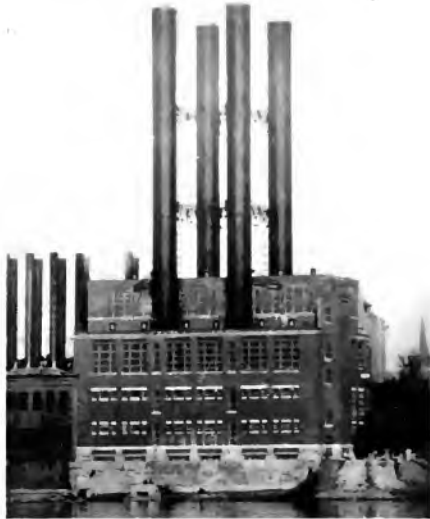
Fig. 8. State St. Station; United Electric Light Co.
