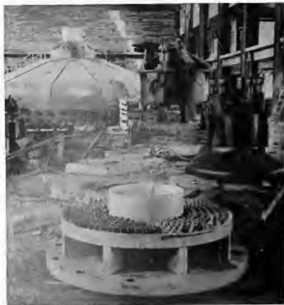
Fig. 1. Parts of Spring Thrust Bearing (in foreground) to Support Load of 550,000 lbs. on ATB-136-pole, 10,000-kv-a., 55.6-r.p.m., 6600-volt Generator, Cedars Rapids Power Station
