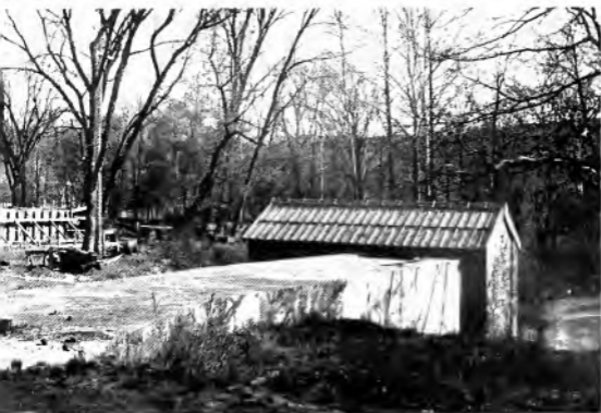
Fig. 5. The turbine is located in the flume, the end of which forms part of the wall of the power house. The turbine consists of two wheels discharging into a draft chest from which the draft tube goes down under the power house
