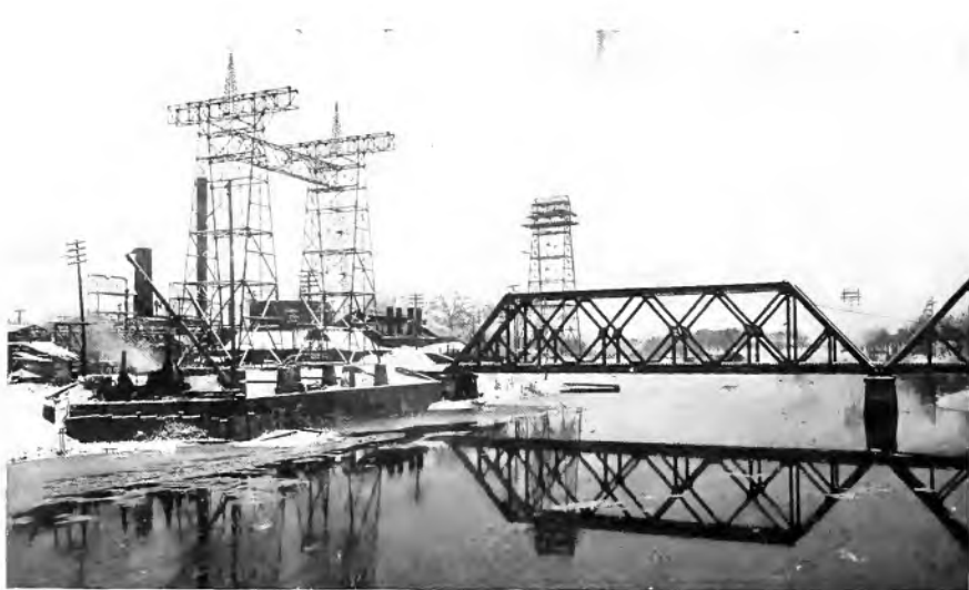
Fig. 19. 66,000-volt: Line Construction Through Westfield, Mass.; Hampden Station
