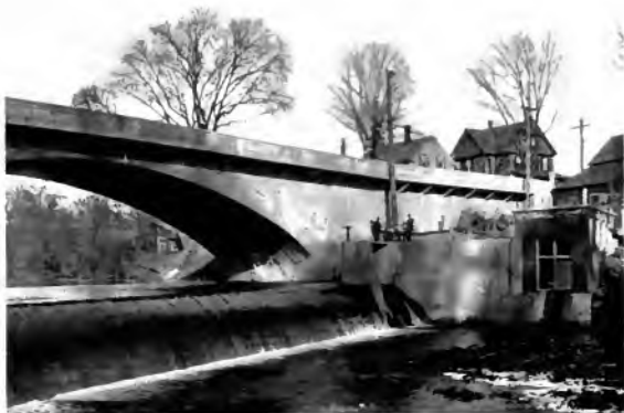
Fig. 2. Green River Plant of Greenfield Electric Light & Power Co. Photograph shows the dam and tiny Power Plant. The cable running up the side of the electric light pole connects this small generating station with the main system.
