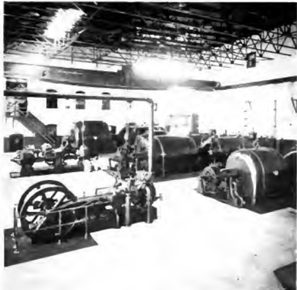
Fig. 9. State St. Station; United Electric Light Co., Turbine Room
