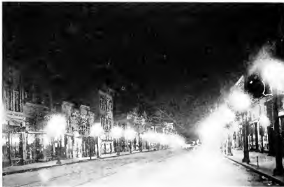
Fig. 12. Night View of the Illumination Produced by the Installation of the Single-lamp Units shown in Fig. 11
