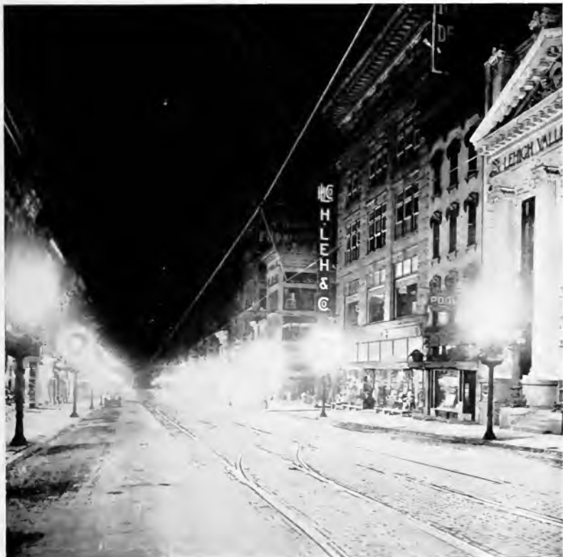
A MODERN ORNAMENTAL NOVALUX LIGHTING INSTALLATION, ALLENTOWN, PA
