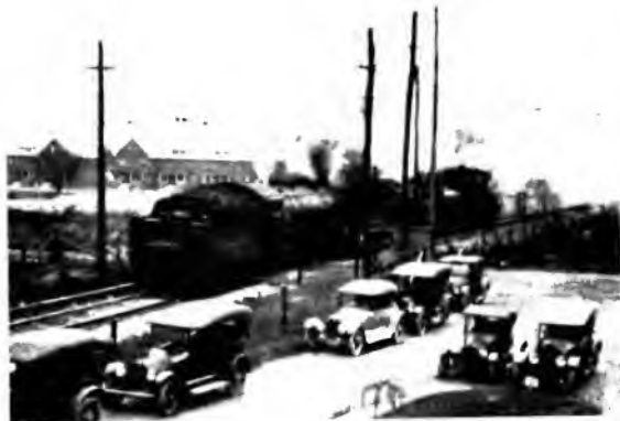
Electric Locomotive Connected for Regenerative Braking and Pushed by Two Steam Locomotives to Simulate the Effect of a Heavy Train Down grade. At times as much as 2000 kw. was returned to the trolley circuit.
