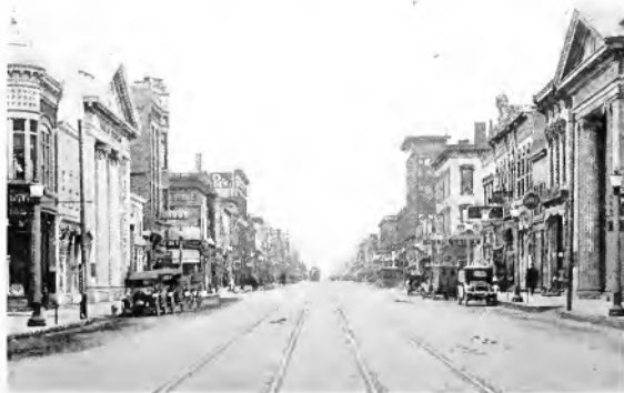
Fig. 11. Day View of Ornamental Street Lighting Installation with Form 9, Novalux Ornamental Units, Sheboygan, Wis.
