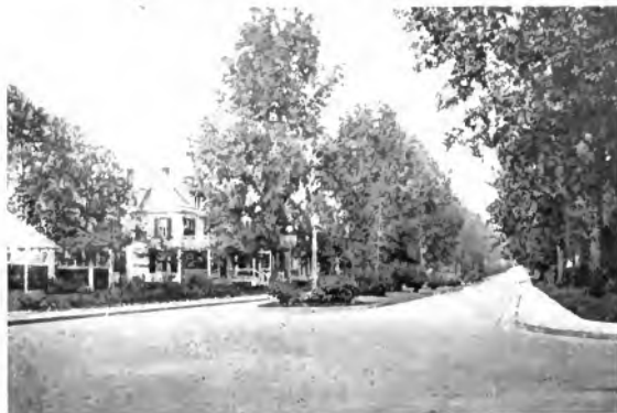
Fig. 14. Day View of Installation of 250 c-p. Mazda Series Lamps in Form 8 Noyax Ornamental Unit, with Stippled Glass Globes and Holophane Prismatic Dome Refractors, Parkwood Blvd., Schenectady, N. Y.
