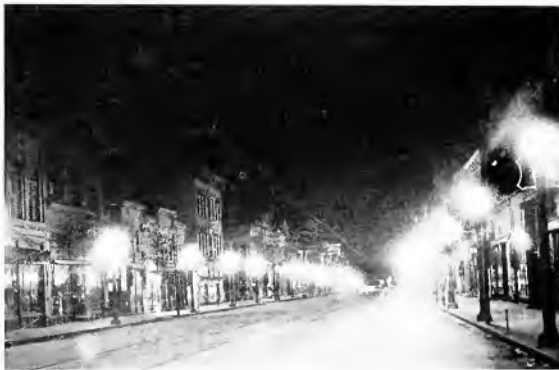
Fig. 12. Night View of the Illumination Produced by the Installation of the Single-lamp Units shown in Fig. 11
