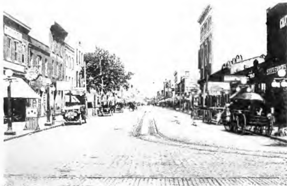
Fig. 9. Day View of Ornamental Street Lighting Installation with Cluster Units
