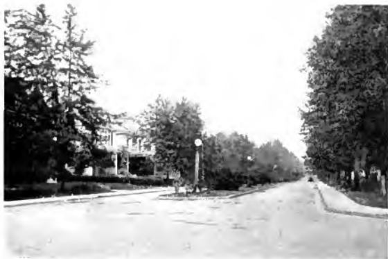
Fig. 13. Day View of Installation of 250 c-p. Mazda Series Lamps in Alabaster Glass Ball Globes, Glenwood Blvd., Schenectady, N. Y.
