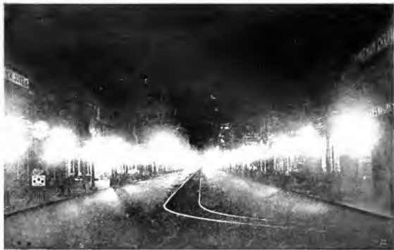
Fig. 10. Night View of the Illumination Produced by the Cluster Lamp Units shown in Fig. 9
