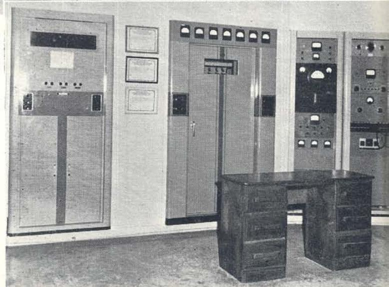
Radio Station KREL, Goose Creek, Texas, is one of the "Show Stations" of the southwest. The station is completely housed in an air-conditioned \$100,000 plant. The Gates BC1-E transmitter and all associated studio equipment, complete phasing units for its three tower directional pattern comprise the apparatus in use for the 1000 watts of transmission. The station is owned and managed by Virgil G. Evans. Mr. M. E. Dougharty is Chief Engineer.
