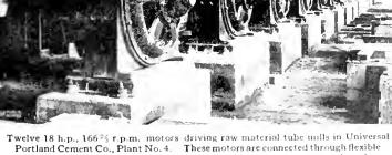
weive 18 h.p., 165<sup>-5</sup> r.p.m. motors driving raw material tube minis in Oniversal Portland Cement Co., Plant No. 4. These motors are connected through flexible couplings to the countershafts of the mills. This arrangement necessitated only one gear reduction. The concrete wall separating the motors from the mills secures an unusually clean motor room
