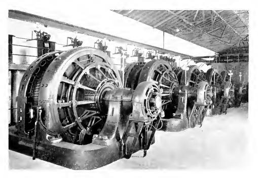
Substation Containing 1500 Kw. Synchronous Motor-Generator Sets
