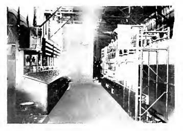
Fig. 4 Control Benchboard and Switchboard
