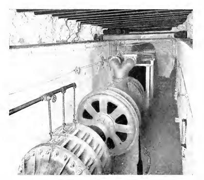
1000 H.P. 2300 Volt 720 R.P.M. Induction Motor Direct Connected to 5000 G.P.M. Six Stage Centrifugal Pump Operating Against 500 Ft. Head, Located at Hampton Water Shed Sump. D.L. & W.R.R. Co. Mining Dept.
