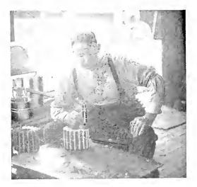
Fig. 3. Testing Gears and Pinions
