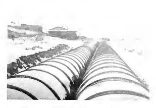
Fig. 7. Steel Pipes, 15 Ft. 6 In. in Diameter
