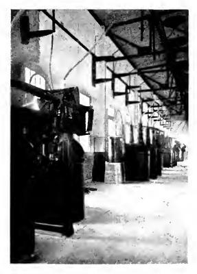
Fig. 19. Interior, Butte Subst ron, showing 100,000 Volt Line Switches
