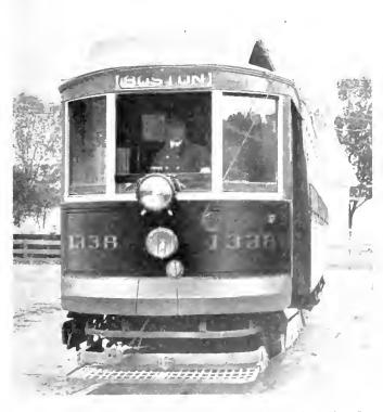
Fig. 3. Four-Ampere Luminous Arc Headlight Installed on Interurban Car
