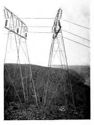
Fig. 14. Line Crossing Missouri River. One End of 3034 Ft. Span
