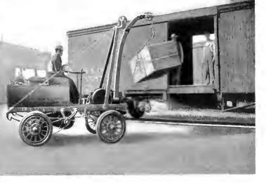
Battery Truck Crane Loading Freight Car
