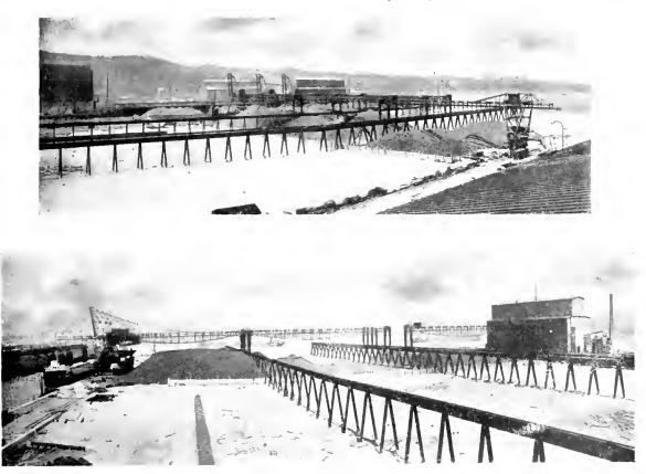
Figs. I and 2. Coal Bridge Equipment of the Pittsburg Coal Dock & Wharf Co., Rice's Point, Duluth, Minn. Three Bridges Equipped with Three 225 H.P. Hoist Motors and Magnetic Control, Six 112 H.P.
