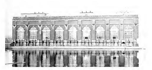
Fig. 4. North View of Power House Showing Racks and Head Gates
