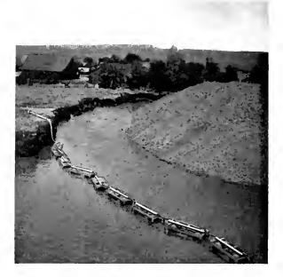
4000 Volt Armored Shore Cable Connecting High Tension with Transformers on Dredge
