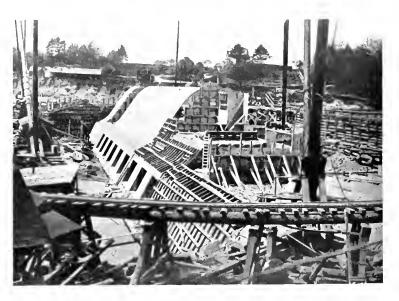
Fig. 2. Spillway of Dam in Course of Construction Showing Location of the 10 Floodgates
