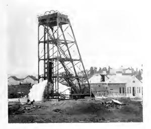
Exterior View of Hampton Water Hoist and Motor House, Showing Bucket Discharging, D. L. & W. R. R. Co, Mining Dept.
