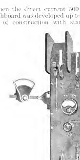
design has in the main been followed in making up other standard panels; office building switchboards being an exception to the rule. Even alternating current panel design follows the general scheme of the original railway panels, with modifications necessary on account of the use of oil switches.
