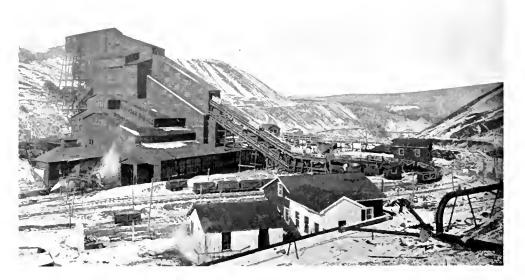
Breaker at Burnside Colliery, Near Shamokin, Pa., Showing Motor-Driven Car Haul Philadelphia & Reading Coal & Iron Co.
