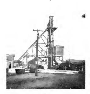
Fig. 23. Mountain View Hoist, operated by Compressed Air
