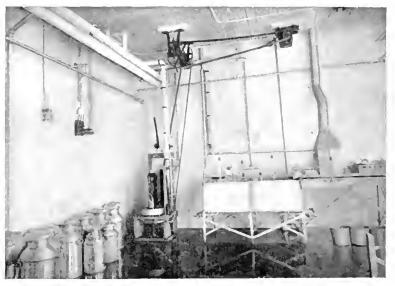
Fig. 3. 2 H P., 220 Volt Induction Motor Driving Can Washer in Creamery
