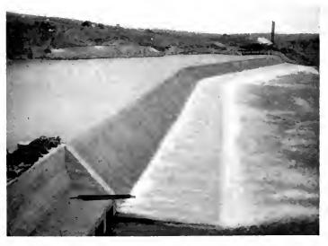
Fig 6. Rainbow Falls Dam; Sluice Gates in Foreground
