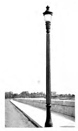
Fig. 5. Installation of Three 4-Ampere Parkway Ornamental Luminous Arc Lamps on Marblehead Causeway
