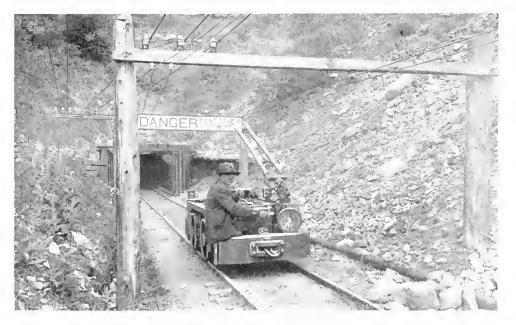
Fig. 8. Five Ton, 220 Volt Double Trolley Direct Current Locomotive at Barton Hill Tunnel
