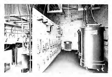
Fig. 9. Switchboard and Transformers for Wiscassett and Cabarrus Mills
