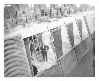
Fig. 4. Showing Construction Work on the Wooden Testing Flumes
