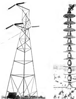
Fig. 2. 140,000 Volt Single-Circuit Strain Tower of the Eastern Michigan Power Company
