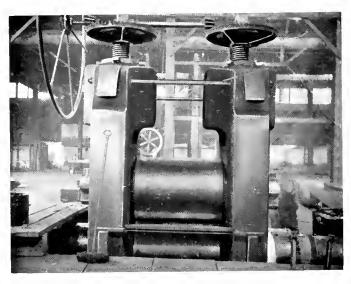
Fig. 14. One Stand of Rolls, 30 in. Sheet Mill
