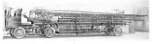
Fig. I Gasolene-Electric Aerial Truck. Tractor made by the Commercial Truck Company of America, Philadelphia
