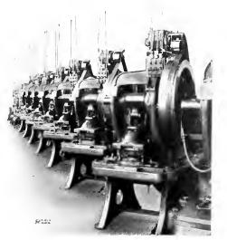
Fig. 9. Ferracute Punch Presses Individually Driven by Induction Motors
