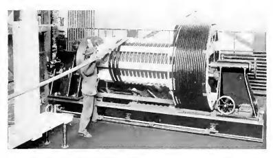
Fig. 2. Winding 400 Kv-a. Reactance with Two 1,250,000 cm. Cables in Parallel
