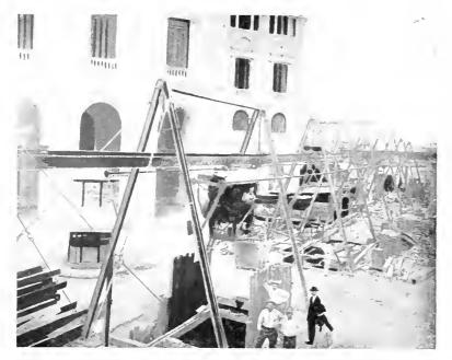
Fig. 9. Portable Monorail Hoist with 10 H.P., 500 Volt Motor. Cuban Engineering & Contracting Company, Havana, Cuba
