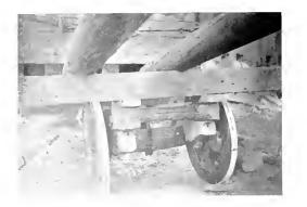
Fig. 7. Unloading Turbine Base-Showing Construction of Cartwheels and Axles
