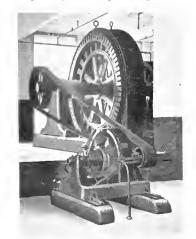
Fig. 1. 1250 Kw. Alternator, Wiscassett Mill
