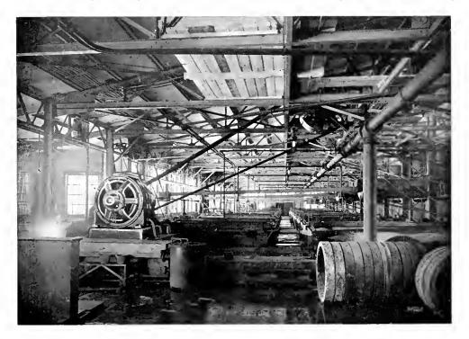
250 H.P., 2300 Volt Motor Driving Section of Regrinding Mill
