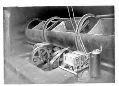
Fig. 12. 20 H.P., 220 Volt Enclosed Motor Operating Three-Car Tipple
