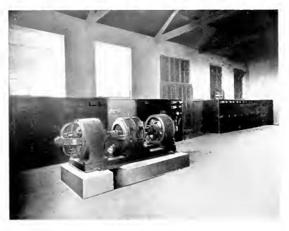
Fig. 3. 3-Unit Set for Excitation of Cogging Mill Motor and its Special Generator. Main Switchboard for Flywheel Set and Mill Motor on the Right
