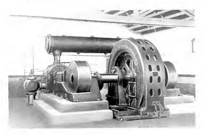
Fig. 14. 400 H.P., 6600 Volt, 136 R.P.M. Induction Motor Direct Connected to 2500 Cu. Ft. Compressor in Cheever Substation
