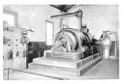
Fig. 4. 750 Kw., 3300 Volt, 1500 R.P.M Mixed Pressure Turbo-Generator, in Central Power Station, Mineville, N. Y.
