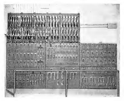
Fig. 5. Switchboard and Banks of Stage-lighting Dimmers at the Hartman Theater, Columbus, Ohio
