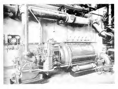
Fig. 21 Turbine-Driven Centrifugal Compressor for Bessemer Converter
