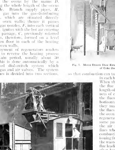
Fig. 6. Locomotive and Car on Discharge Side of Ovens. Partial Quenching Takes Place Here
