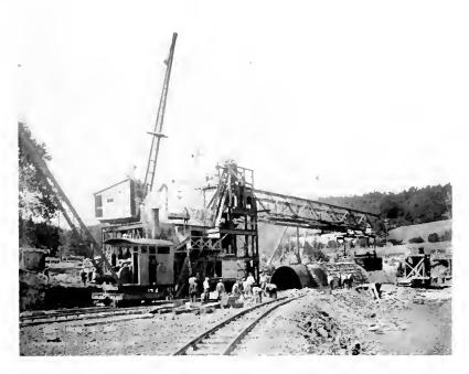
Fig. 2. Travelling Concrete Plant, the Principal Apparatus of which is Operated by Electric Motors
