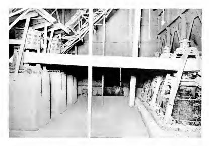
75 H.P., 400 R.P.M, 60 Cycle, Vertical Induction Motors Driving Giant Griffin Mills Knickerbocker Portland Cement Company, Hudson, N. Y.
