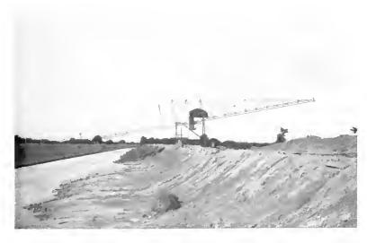
Fig 7. Cantilever Crane Operating Drag Bucket made by Brown Hoisting Machinery Co. 225 H.P., 400 Volt Induction Motor. The United Engineering & Contracting Company, Barge Canal Contract No. 40, Lockport, N. Y.
