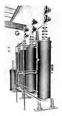
Fig. 10. One of the 70,000-Vclt Electrolytic Lightning Arrester Sets in High Tension Room
