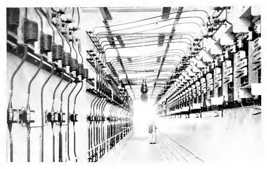
Fig. 8. Interior of Substation showing Lightning Arresters
