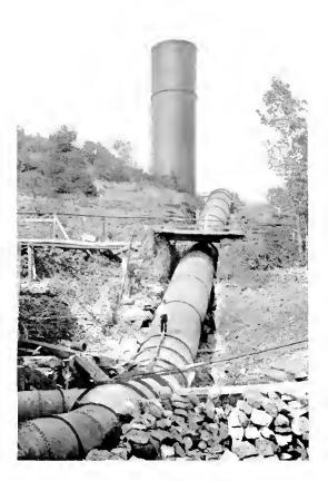
Fig. 5. Section of Penstock Between Stand Pipe and Power Station
