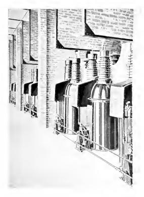
Fig. 9. Arrangement of 70,000-Volt 150 Ampere Oil-Switches
