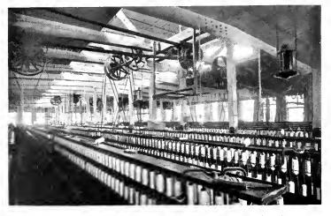
Fig. 4. Group of Spinning Frames in Cabarrus Mill, Driven by Motor Located Overhead
