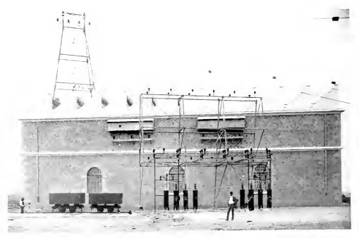
Fig. 7. Back of Substation showing High Voltage Line Entrance
