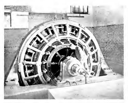
Fig. 1. 1200 H.P. Direct-Current Motor for Driving 28 In. Cogging Mill
