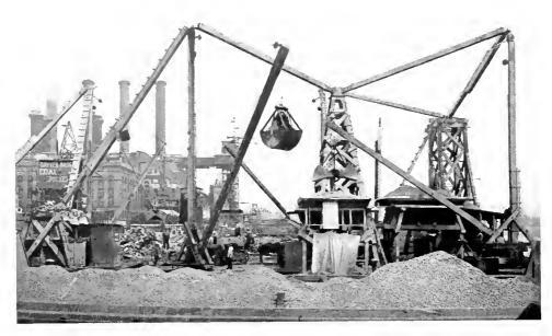
Fig. 5. Electric Derricks, East 35th Street Dock. The United Engineering & Contracting Co.
