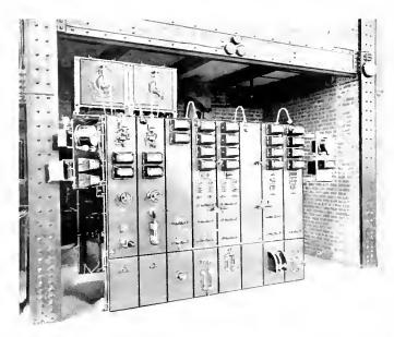
Fig. 11. Front Panels of Main Power Station Switchboard
