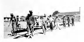
Fig. 11. Carrying One of the Completed Roof Trusses to Site of Station
