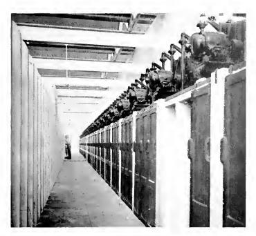
Fig. 9. Interior of Substation showing 6600 Volt Oil Switches
