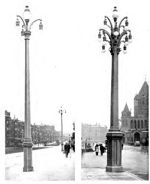
Fig. 2. One of the Poles Used for the Spectacular Illumination of Huntington Avenue, Carrying Four Colored Flame Arcs, the Upper One Pale Green, the Lower Three Light Rose Pink
