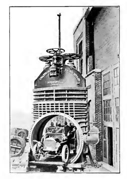
Fig. 1. Motor Operated Valve of the Ontario Power Company
