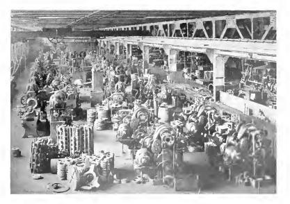
Fig. 10. Various Machine Tools with Individual Motor Drive
