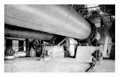
75 H.P., 720 R.P.M., 60 Cycle, 440 Volt, Slip Ring Induction Motors Driving Rotary Kilns. Knickerbocker Portland Cement Company, Hudson, N. Y.
