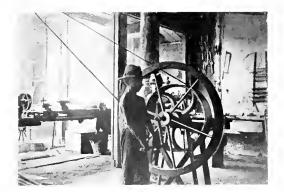
Fig. 10. A Chinese Machine Shop—Two Boys Driving an Engine Lathe
