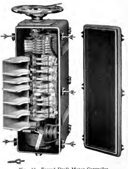
Fig. 12. Forced Draft Motor Controller
