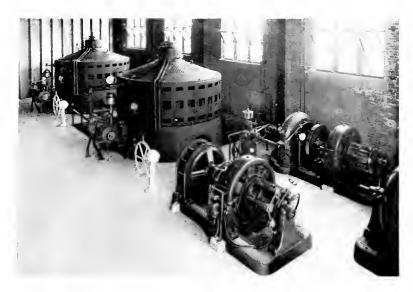
Fig. 6. Arrangement of 2800 Kv-a., 25-Cycle, 2300-Volt Water-Wheel-Driven Alternators and Exciters
