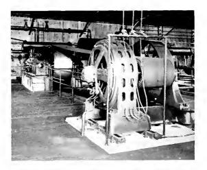
Fig. 4. Air Compressors Driven by 500 H.P. Induction Motor
