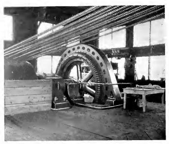
Fig. 13. Induction Motor Driving 30 in. Four-Stand Sheet Mill
