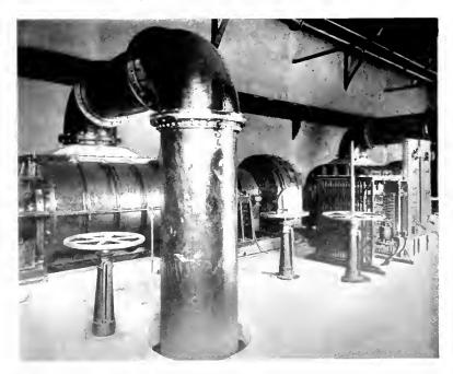
Fig. 8. Gas Exhausters Operated by 250 H.P. Motors
