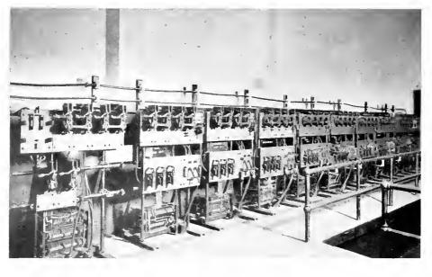
Series Contactor Panels Controlling Induction Motors in Steel Mill Service
