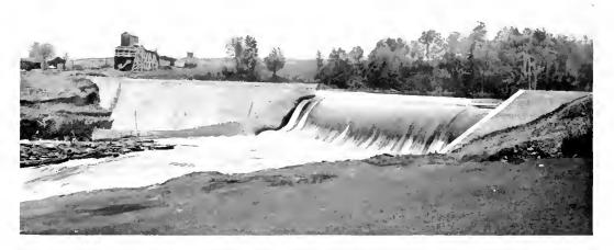
Fig. 3. View From Down Stream Showing Spillway and Impounding Section of Dam
