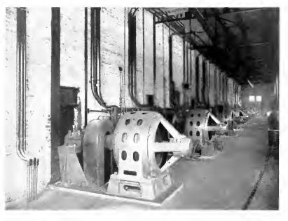
Fig. 2. 250 H.P. Squirrel-Cage Motors Driving Hammer Mills
