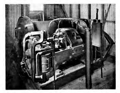
Fig. 6. 90 H.P., 550-230 Volt D.C. Motor Geared to Lidgerwood Mnfg. Company Mine Hoist. Smith, Hauser, Locher & Co. Catskill Aqueduct Contract 66, New York City
