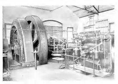
Fig. 3. 750 Kw., 3300 Volt, 94 R.P.M Alternator driven by 1000 H P. Engine, Central Power Station, Mineville, N.Y.
