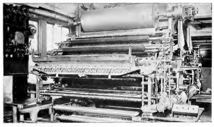
Fig. 8. Hoe Rotary Magazine Press Driven by 15 H.P. Direct Current Motor with Full Automatic Single Motor Controller
