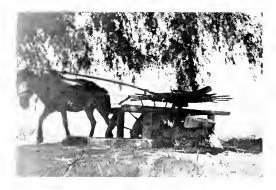
Fig. 13. A Primitive Form of Bevel Gear Driven Waterwheel for Irrigation Purposes
