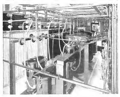
Fig. 12. Three 50 Kv-a., 6600/460 Volt Transformers for Power: Three 10 Kv-a. 6600/130 Volt Transformers for Lights
