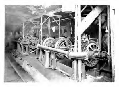
Fig. 3. Induction Motor-Driven Pumps
