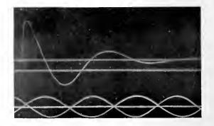
Fig. 3. Line Oscillating as a Whole. Upper curve, current at generator end of line; lower curve, 60-cycle timing wave.
