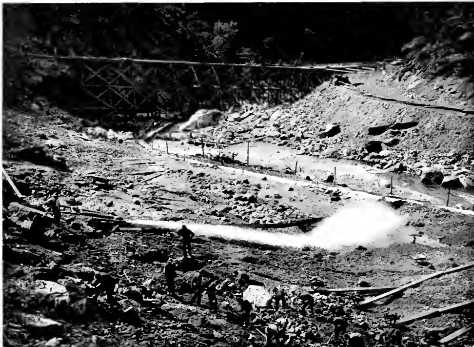
Fig. 4. Excavating for Power House No. 2. A Large Portion of this Work was done by Means of a High Pressure Stream of Water, as shown
