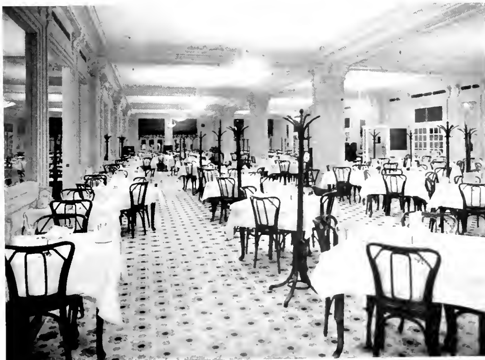
Fig. 4. An Excellent Method of Lighting a Dining Room, Semi-indirect Units being Employed
