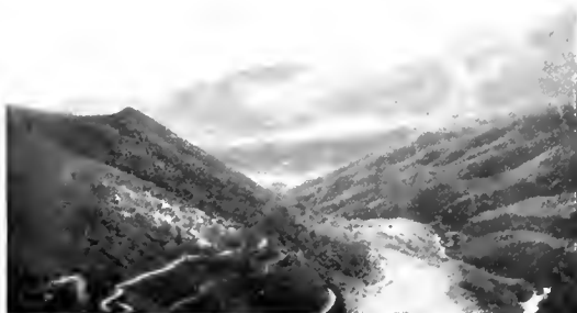
Fig. 10. The Peak of the Hill with the Winding Cart Road on the left-hand side shows the site of the 200-ton stamp mill, shops etc., of the Rosario Mines before construction work began
