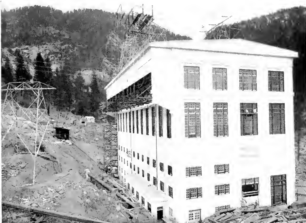
Fig. 8. Power House No. 1 showing Line Entrance and Lightning Arrester Horn Gaps on Roof of Building
