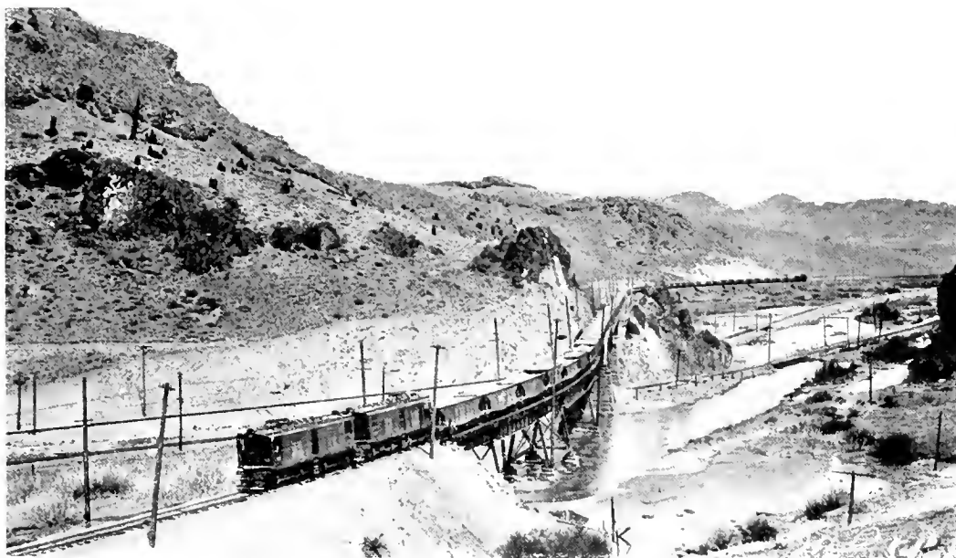
160-Ton Electric Locomotive Hauling 4550-Ton Ore Train, Butte, Anaconda and Pacific Railway
