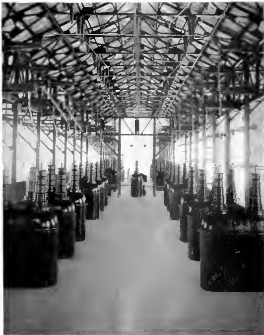
Fig. 14. High Tension Switch Room
