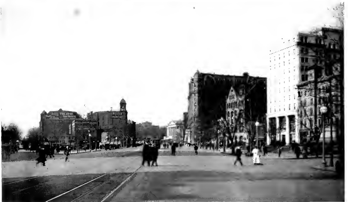
Fig. 12. Two Views of Pennsylvania Avenue Taken Toward the Treasury Building showing the Appearance of the Lighting Units as Installed
