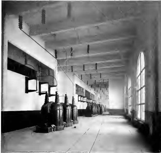
Fig. 18. Completed Section of West High Tension Room, Fourth Floor
