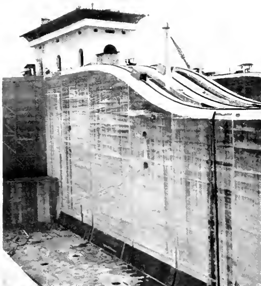
Fig. 4. Control House for Center Wall. Upper Locks at Gatun. Towing track incline between upper and intermediate locks. July 22, 1913
