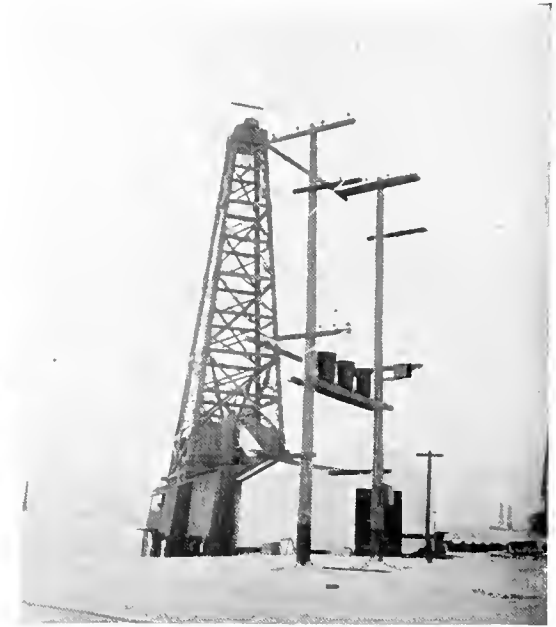
Fig. 14. Well No. 3 of the Midway Pacific Oil Co., Fellows, Cal., drilled entirely by electric power. Depth 1900 feet. The transformer installation is typical of the oil fields
