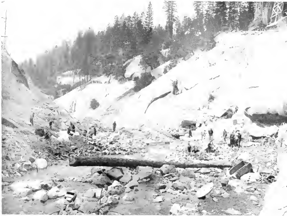
Fig. 1. Excavating for Dam No. 4. Looking Down Stream
