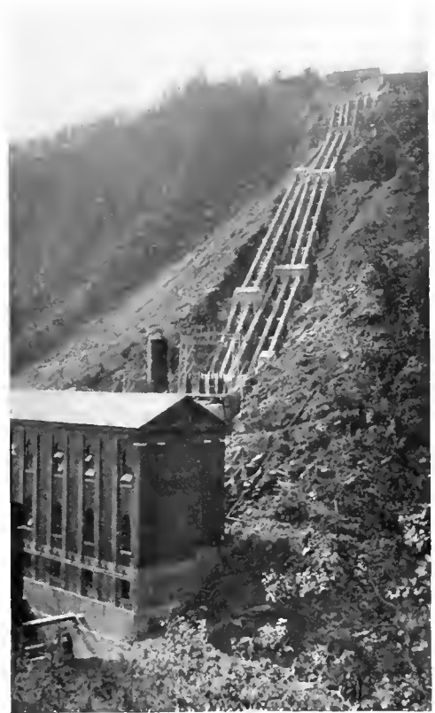
Fig. 5. Forebay and Penstocks
