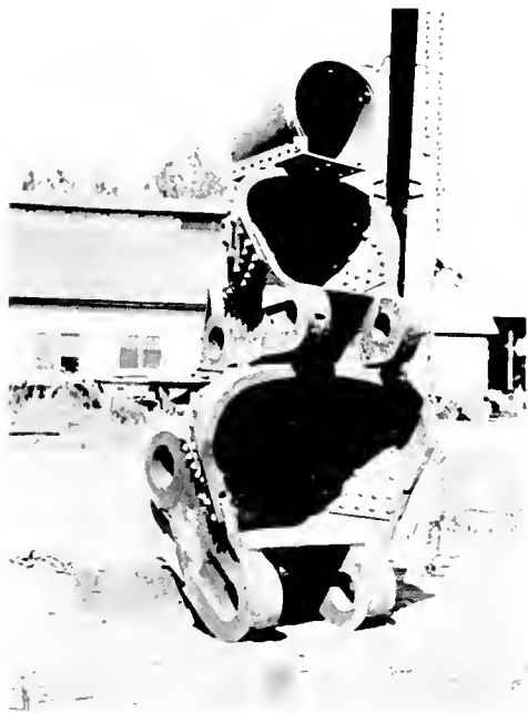
Fig. 1. A Comparison of: Bucket of First Dredge on Yuba River 7 Cubic Foot Bucket of Early Dredges 15 Cubic Foot Bucket of Yuba No. 13
