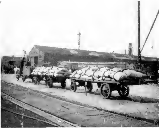
Battery Truck Crane Towing Fifty Bags of Coffee from Wharf Building to Warehouse. The rope slings are for hoisting the bags to upper floors
