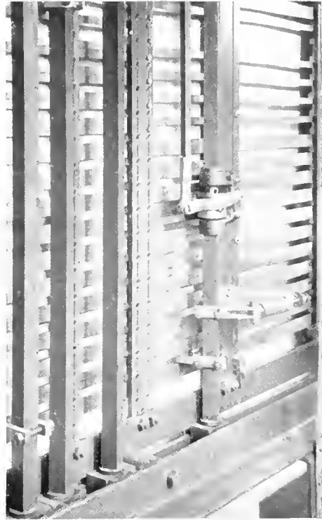
Fig. 13. Interlock Relieving Clutch and Auxiliary Spring for Intermediate Gates
