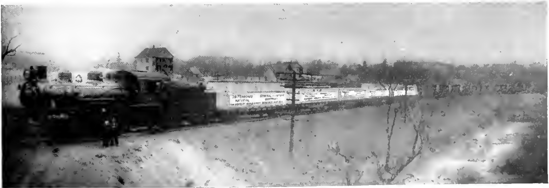
Fig. 14. Train Load of Switchboard Material for Tata Hydro Electric Power Company, Bombay, India
