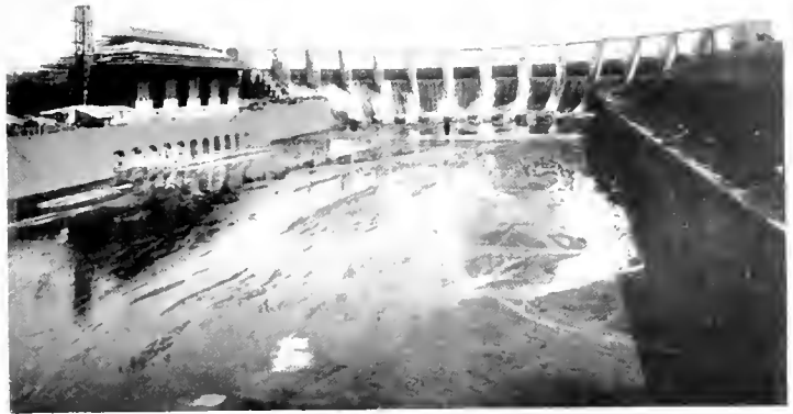
Fig. 3. Gatun Spillway Dam, looking South from Bridge, showing 14 Crest Gates. Ogee Dam and Baffle Piers. Hydro-Electric Station at Left
