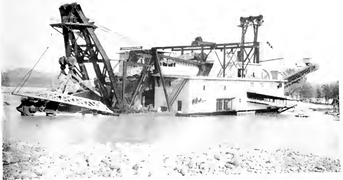
A View of the Yuba Gold Dredge showing the Digging Ladder Raised
