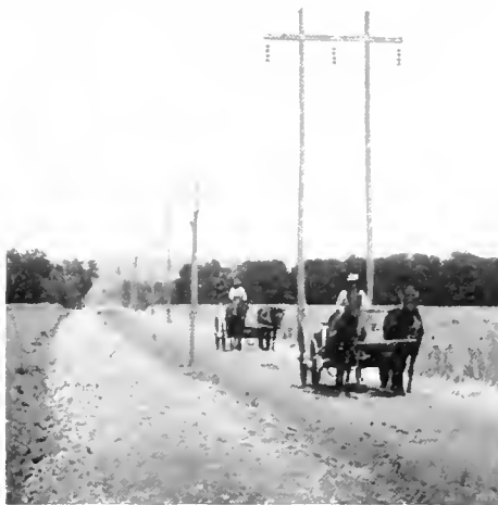
Fig. 30. 66,000 Volt Line to Alton, Looking Towards Illinois River Crossing
