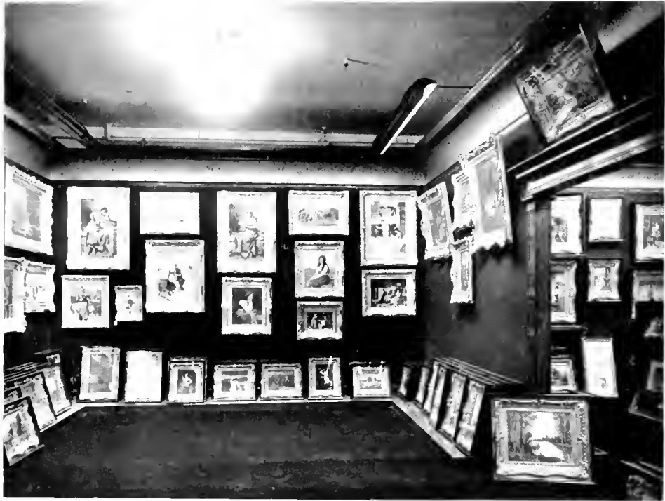
Fig. 1. A Good Method of Low-Intensity Direct Illumination, Especially Suited to Art-Gallery Lighting
