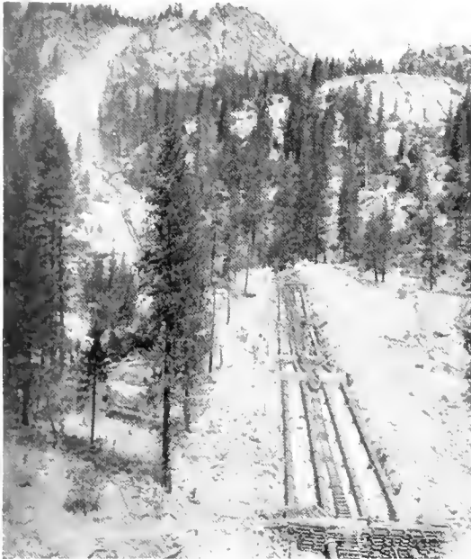
Fig. 5. Penstocks for Power House No. 1
