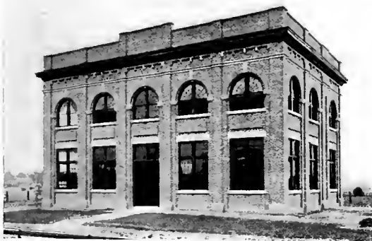
Fig. 2. Exterior View of Clark Mills Substation, Oneida Line
