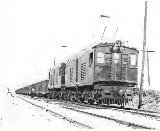
Fig. 8. 2400 Volt Locomotive Hauling Ore Train, Butte, Anaconda and Pacific R. R.
