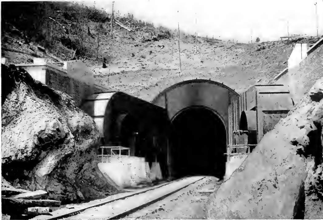
View Showing Position of Ventilating Equipment and Tunnel Portal
