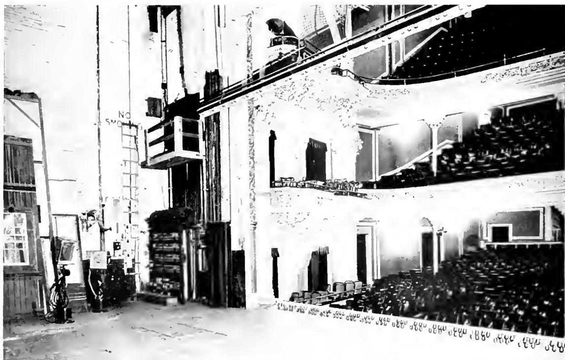
Fig. 2. Partial View of Stage and Auditorium Including Border-light, Double-row Footlight, Stage Switchboard, Boxlight Lens Lamp, Dimmer, Magazine Panel, Company Service Switch and Portable Strip-light
