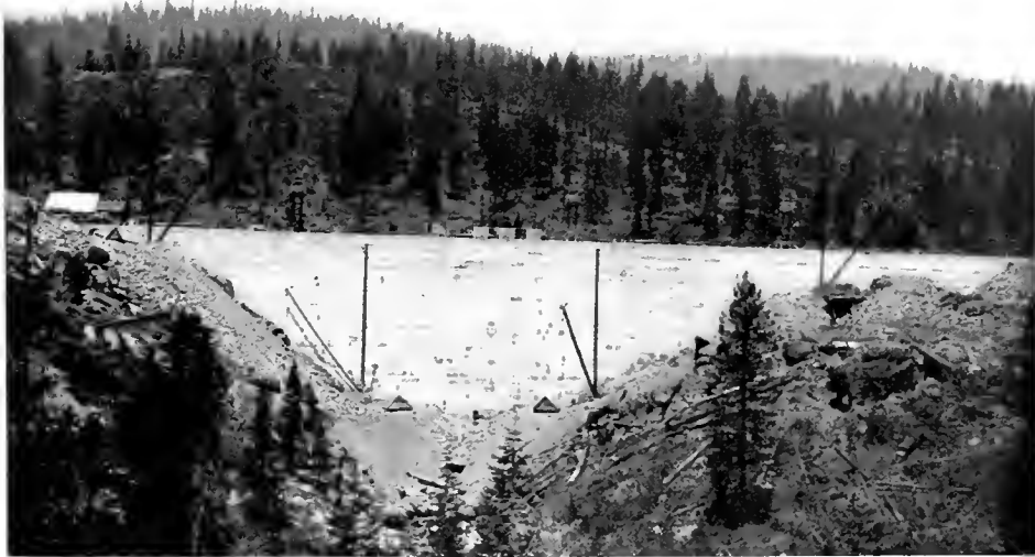
Fig. 3. Dam No. 1 Completed
