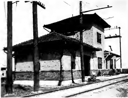
Standard Substation and Waiting Station
