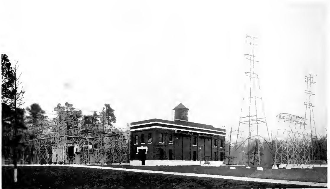
A 110,000 Volt Outdoor Substation. Georgia Railway & Power Company
