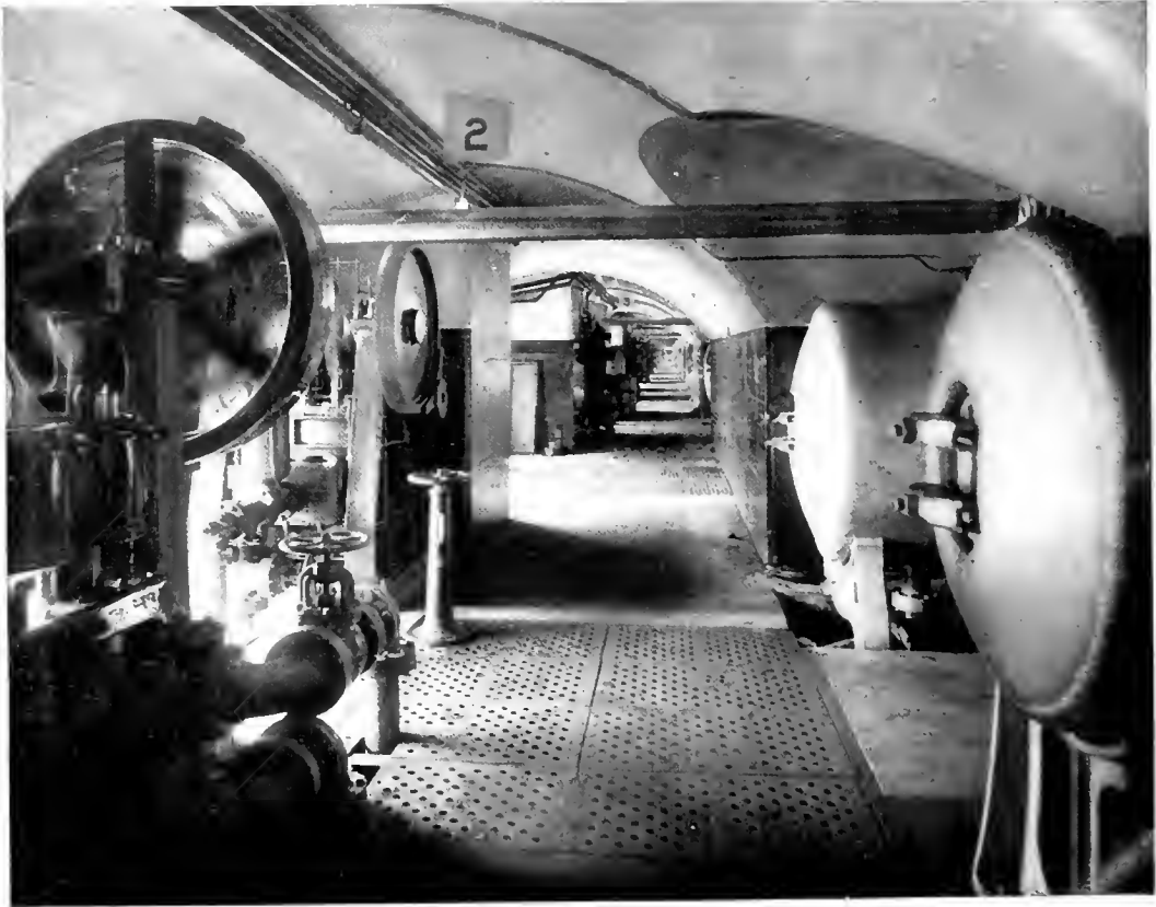
Fig. 10. Looking South Through Machinery Tunnel
