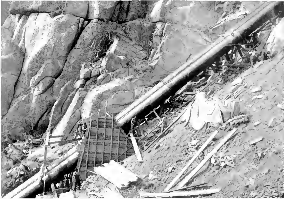
Fig. 7. Placing Forms for Anchors for Penstocks, Power House No. 1
