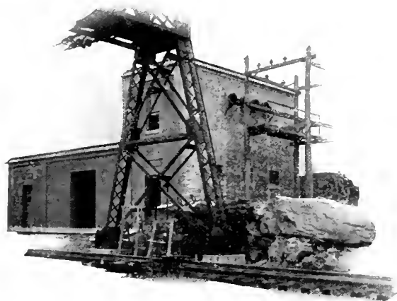
Fig. 16. Exterior of New York, Westchester & Boston Rwy. Signal Substation, Columbus Ave., Mt. Vernon, N. Y.
