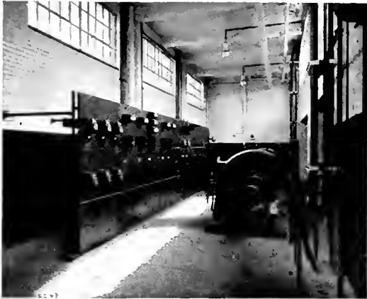
Fig. 16. Front View of the Synchronous Converter Switchboard. (Back View, Fig. 11)
