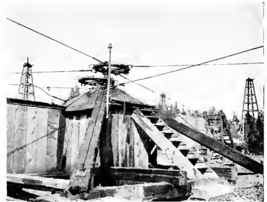
Fig. 8. Power-Head Driven by a 20 h.p. Motor in the Sherman Salt Lake Oil Fields, Los Angeles, Cal.
