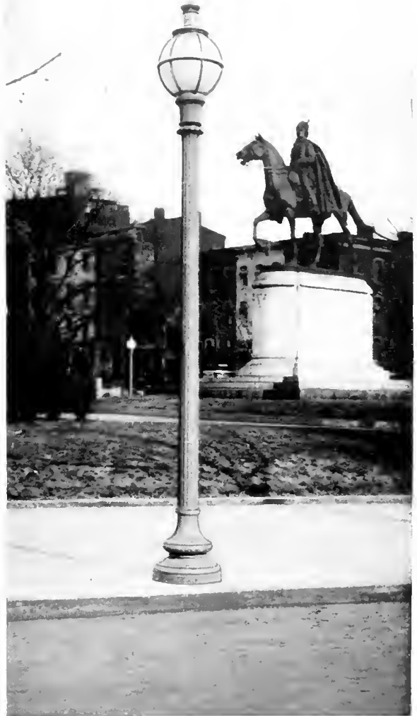
Fig. 13. A Near View of One of the Lighting Units
