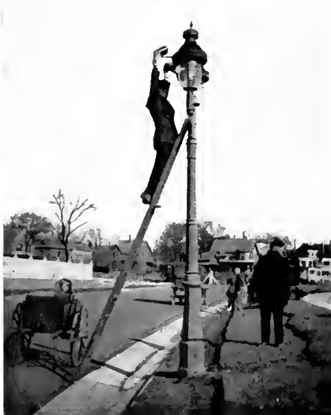
Fig. 1. The Method Used in Filling the Lamps of the Old Gasolene-Mantle Lighting System
