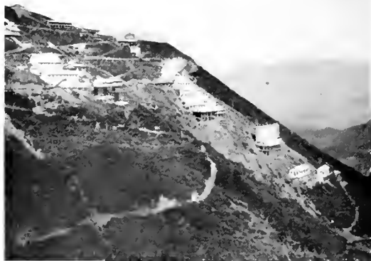
Fig. 11. A near view of the mill site when construction work was nearly completed
