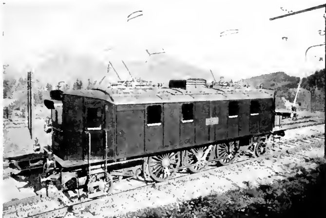
Fig. 10. Midi Railway, France. Experimental locomotive. Motors coupled with triangular rod
