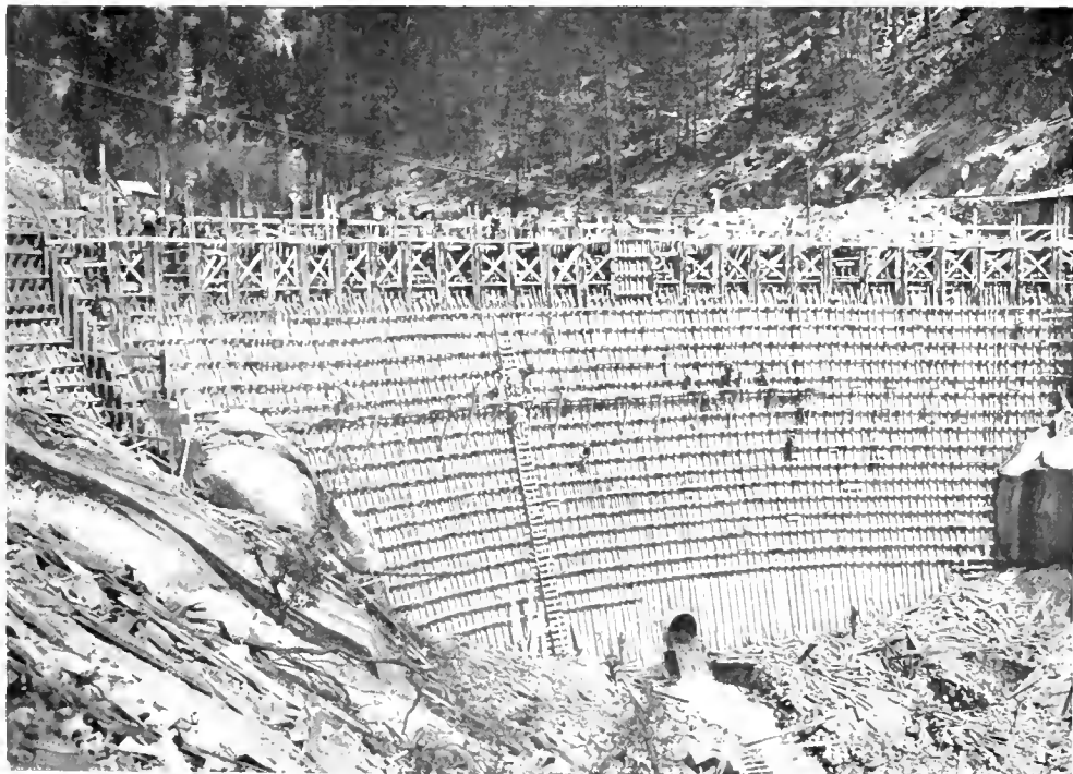
Fig. 2. Dam No. 4 in Process of Construction. Down Stream Side
