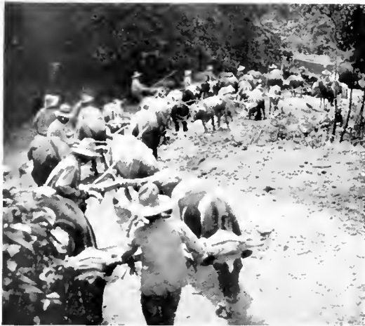
Fig. 2. Twenty-six Oxen Pulling a Wagon Loaded with a 6-ton Rotor of a 38-pole Low-speed Induction Motor. The number of oxen is increased to 40 on steeper grades. Note the disadvantage at which the oxen pull around the curve
