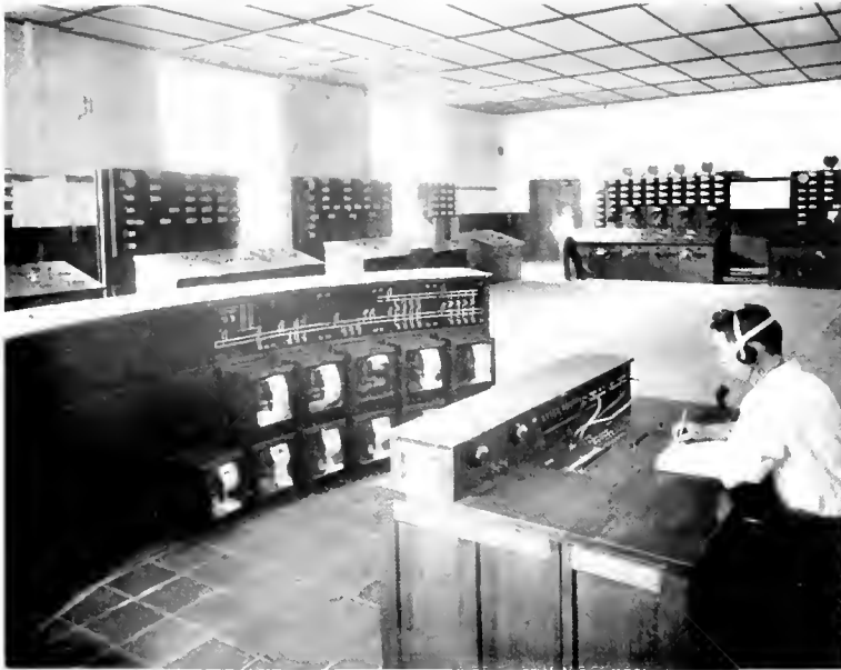
Fig. 22. Chief Operator's Room, showing Control Board and Switchboards
