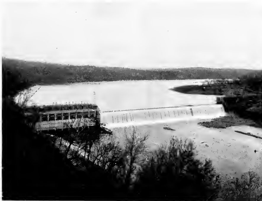
Fig. 1. General View of the Hydro-Electric Power House and Dam
