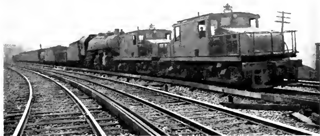
Fig. 7. Two 100-ton Freight and Passenger Locomotives, Type OE-1 and OE-2, each equipped with four GE-209 Motors hauling freight train
