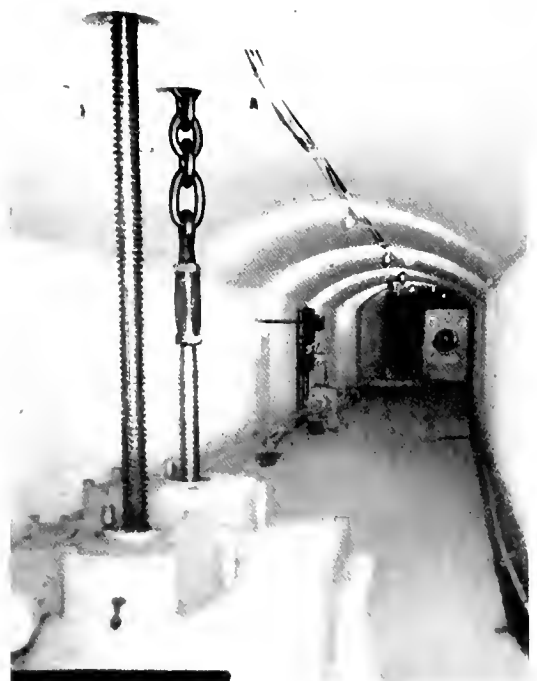
Fig. 9. The Gatun Spillway Machinery Tunnel
