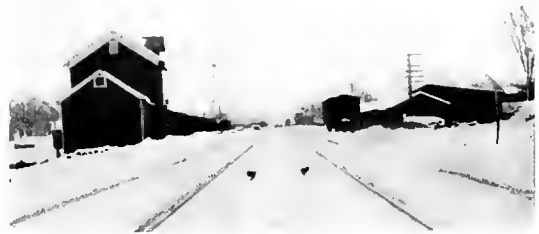
Fig. 8. View of Third Rail under Snow Conditions, Oneida Line
