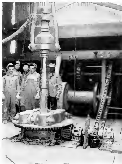
Fig. 10. Rotary Drilling Rig and Crew
