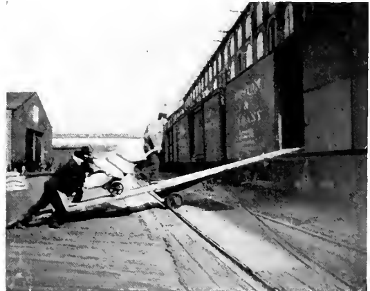
Loading a Freight Car by Hand under the Brooklyn Bridge
