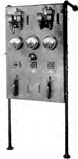
Fig. 2. Switchboard for Series Line Charging, New York Central & Hudson River Railroad
