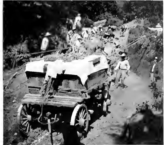
Fig. 3. Wagon loaded with a generator armature on way to the mines, block and tackle being used to assist in the ascent
