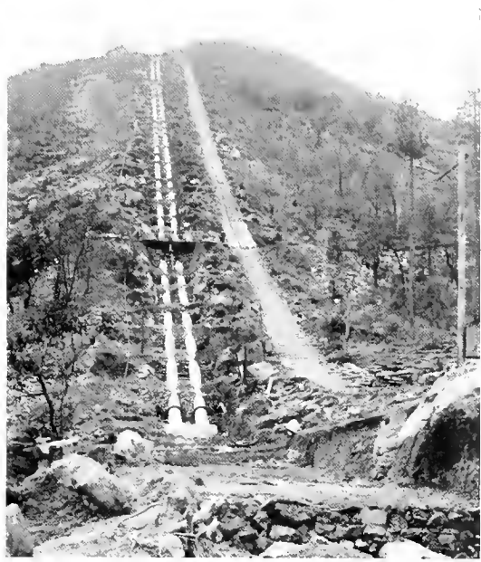
Fig. 6. Penstocks for Power House No. 2
