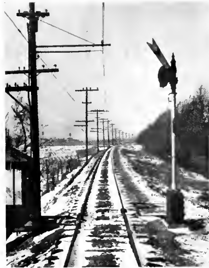
Distance Signal in "Proceed" Position. Also showing High Tension Overhead Construction, Trolley, Feeder, Telephone and Signal Wires
