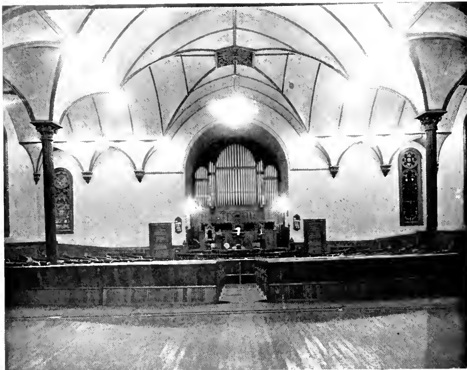
Fig. 3. An Example of Poor Lighting. The Lamps are in the Line of Vision and Produce a Uniform Brilliancy
