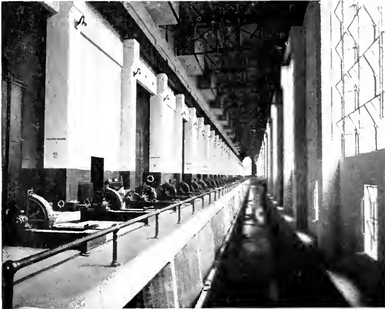
Fig. 7. Looking South Through Gate Room, Showing Gate Mechanisms in Place August 4, 1913
