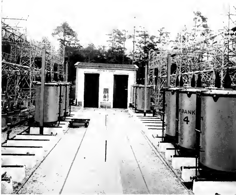
Fig. 13. Atlanta Substation. Repair House in Middle Distance
