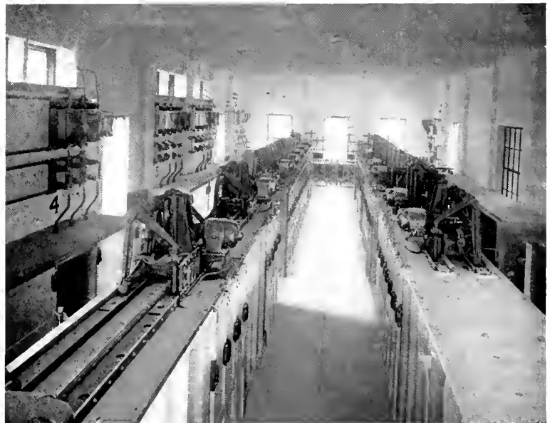
Fig. 14. Low Tension Oil Switch in Atlanta Substation
