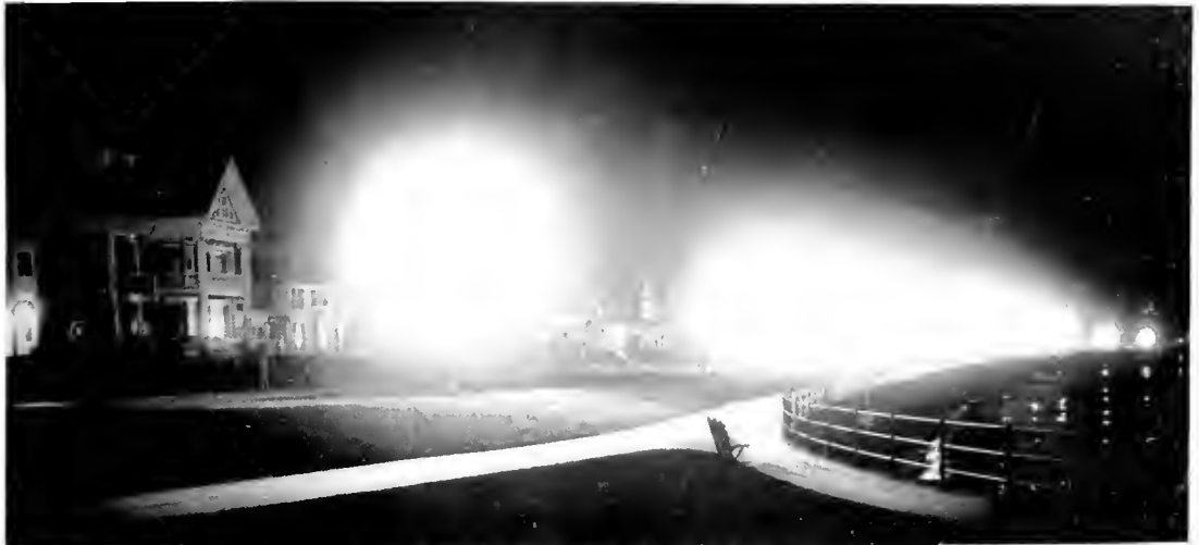
Fig. 4. A Night Photograph showing a Portion of the Boulevard as Lighted by the New Luminous-Arc System
