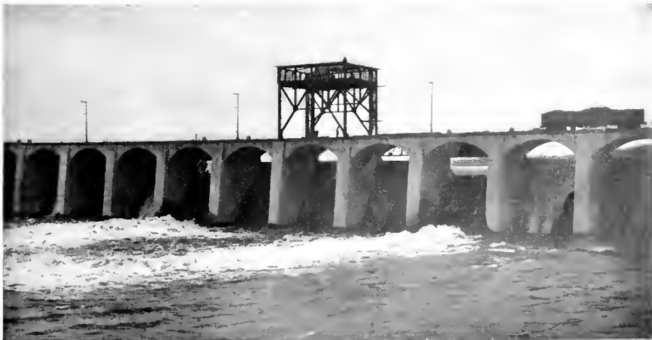
Fig. 4. Downstream Side of Dam
