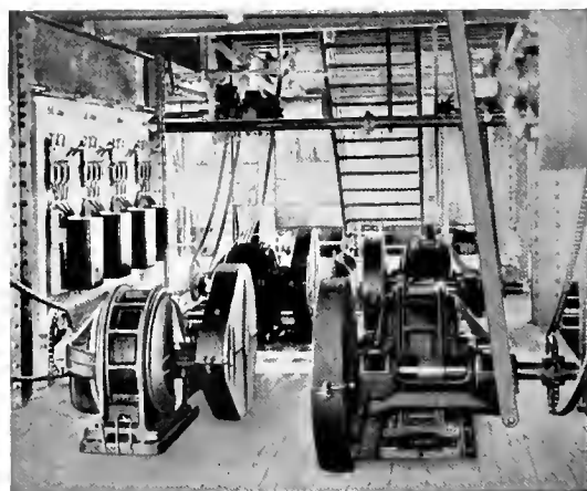
Fig. 3. Back-g geared Motors Driving Crystallizer Counter-shafts by a Chain Drive
