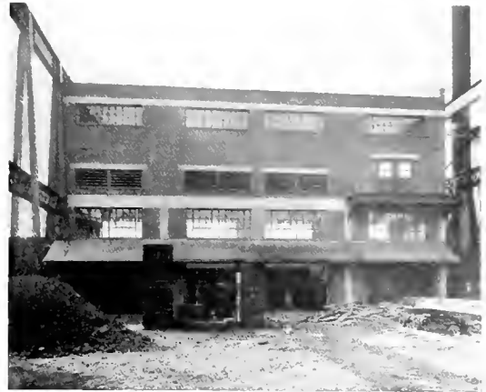
Fig. 3. Substation Building, Front View from Yard
