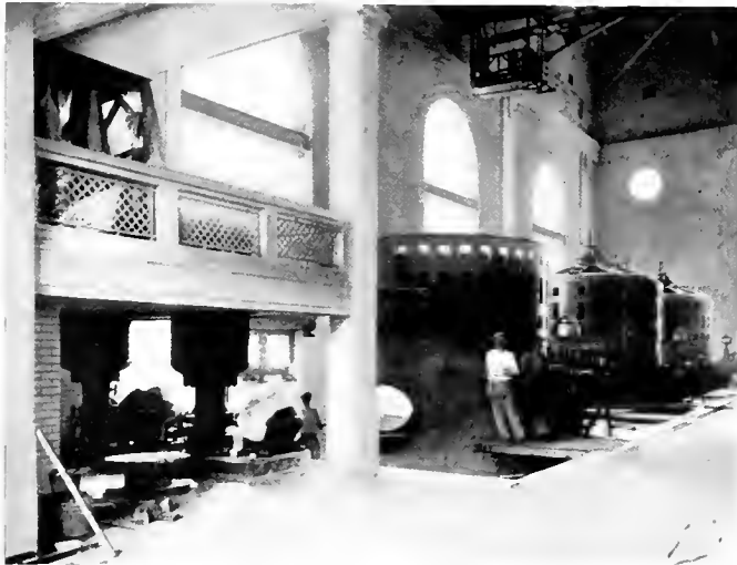
Fig. 3. Interior View of Gatun Hydro-Electric Station
