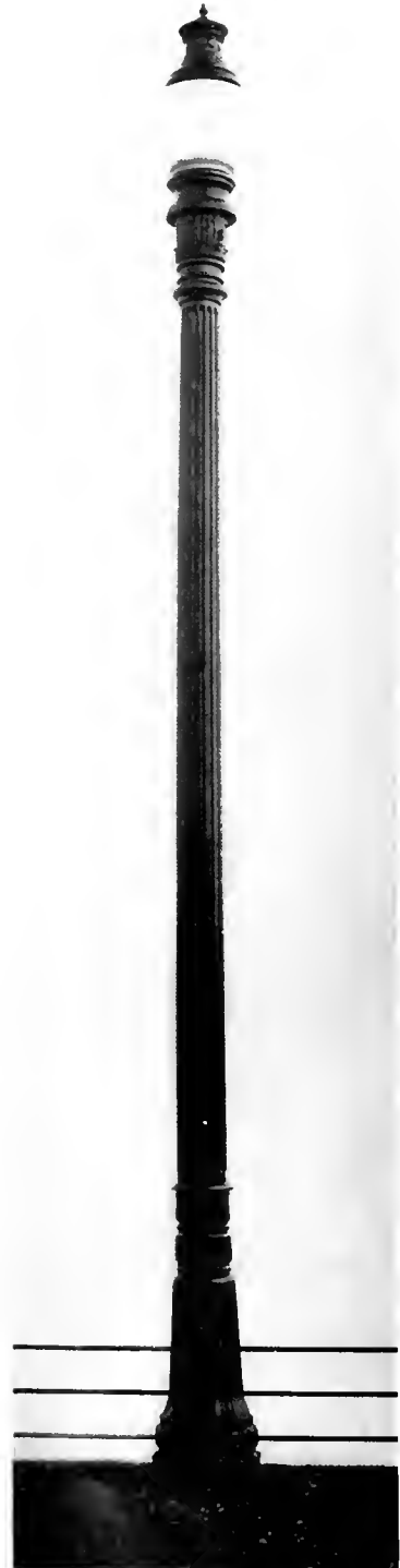
Fig. 6. A Complete Luminous-Arc Unit as Installed in the Boulevard Lighting System
