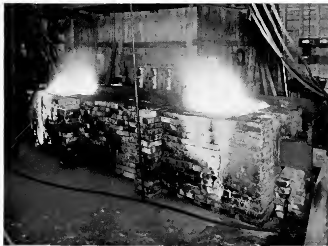
Fig. 5-B. Resistance Furnace in Operation, showing gases burning above contact area between electrodes and charge
