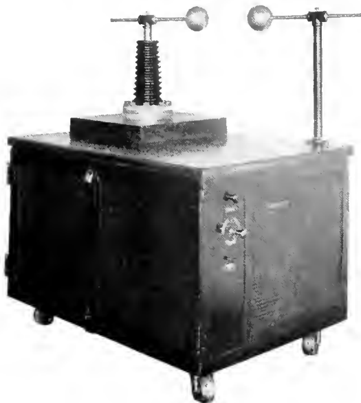
Oscillating Current Transformer
