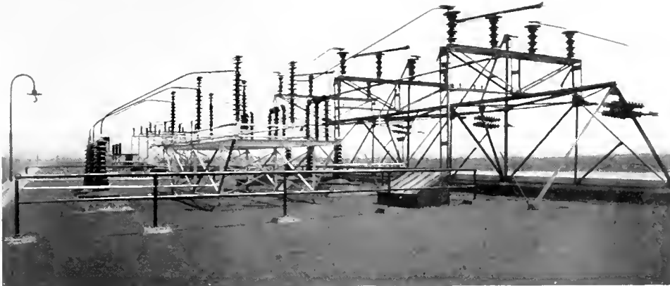
Fig. 26. Roof Structures for 110,000 Volt Line Entrance
