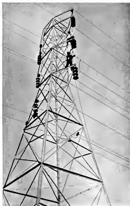
Fig. 1. Photograph of a Standard Line Tower of the Georgia Railway & Power Co., Showing the Power Wires and the Telephone Wires and Their Transposition
