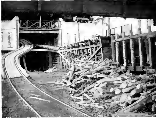
Fig. 6. Inclined Track at Ingenio San Manuel Sugar Co., Cuba, to take care of the wood fuel needed to help the bagasse in the process of evaporation, and for which the bagasse alone is insufficient
