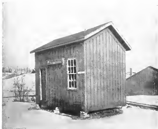
Fig. 3. Exterior of an Early Central Station Lighting Plant, Appleton, Wis. Capacity 250 Lights or Approximately 11 Kw Interior View shown in Fig. 2, Page 256
