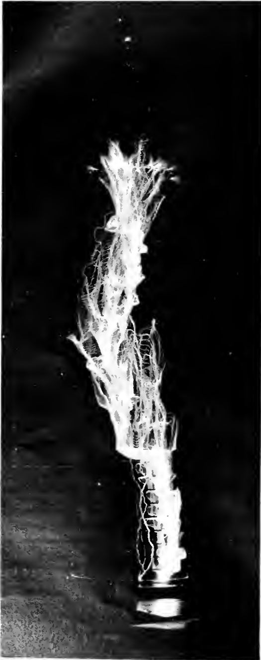
Fig 4 Photograph of a High Tension Lead Flash Over at 400,000 Volts
