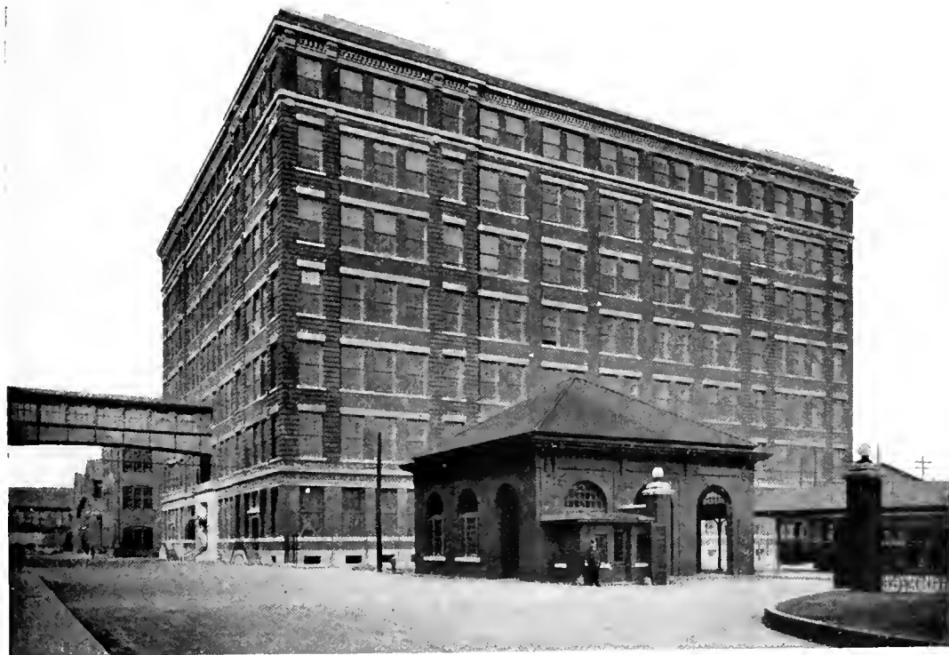
Fig. 1. Research Laboratory Building
