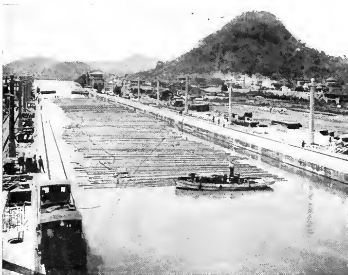
Fig. 8 Electric Locomotives Locking 85-ft. Piles through the Pedro-Miguel Locks
