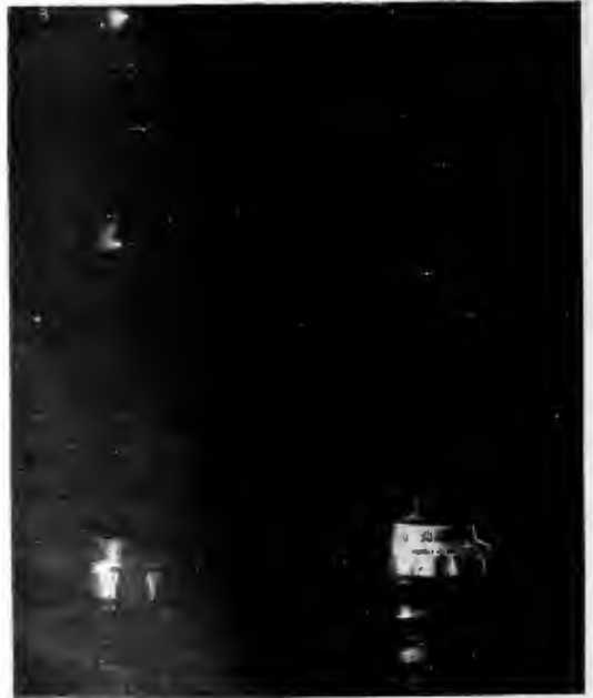
Fig. 1. Five Minute Negative Exposure of Two Oil-Filled Porcelain Leads in Multiple at 175,000 Volts. The Resistance in Series with Lead on Left, 260,000 Ohms in Series with Lead on Right
