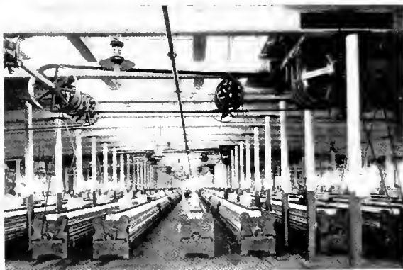
Fig. 11. Typical Group Drive in Ring Spinning Room
