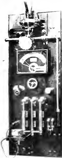
Fig. 14. Early Panel Switchboard—1892
