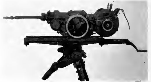
Fig. 2. Left-hand Side of Drill showing Belt and Tightener
