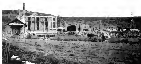
Fig. 7. A Substation and Outside Equipment of the Utah Power and Light Co.
