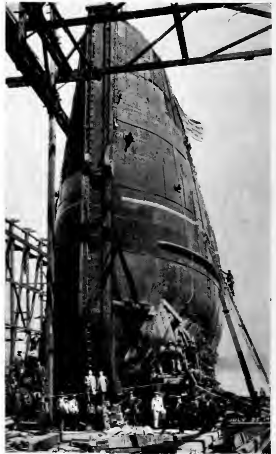
Fig. 1. An End View of the Caisson Taken but a Short Time Before it was Launched
