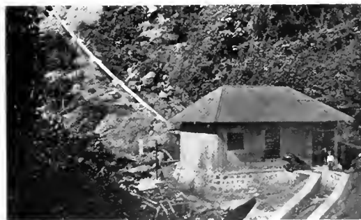
Fig. 2. Hydro-electric Power Plant at Finca Ona
