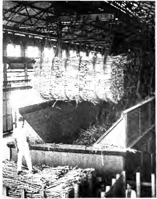
Fig. 60. 30-h.p. Induction Motor Driving Cane Hoist in Sugar Mill
