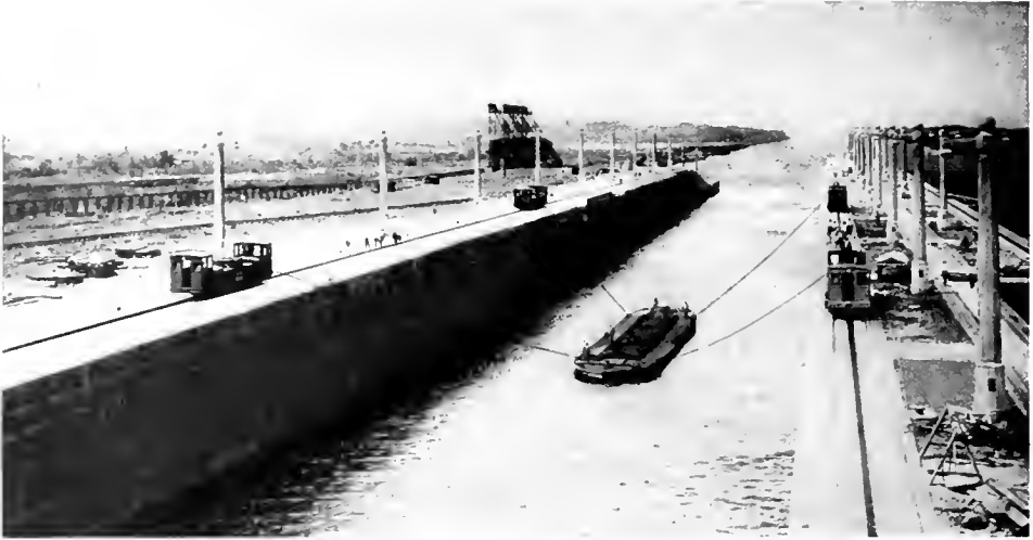
Fig. 10. The First Trial Run of the Towing Locomotives at the Gatun Locks. A barge was used in making this test
