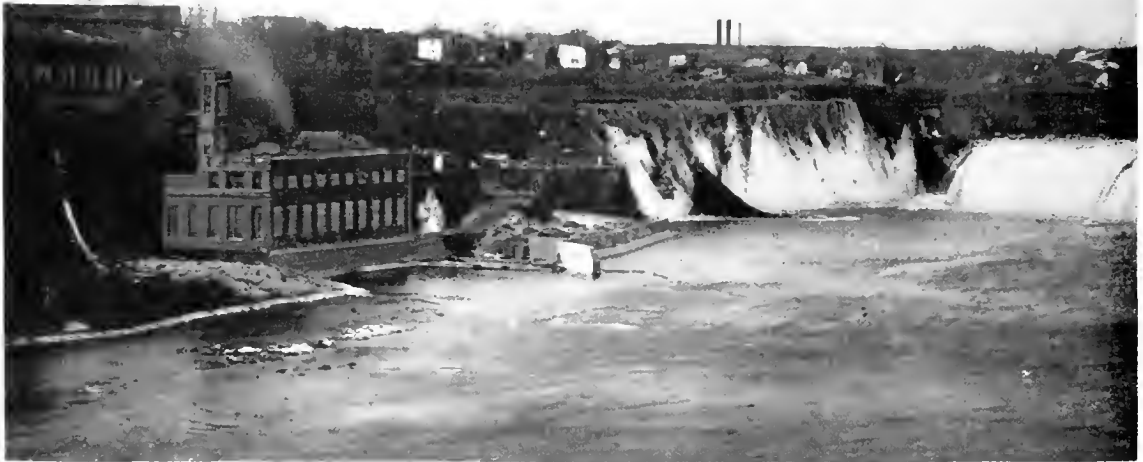
Fig. 3. View of Power House and Cohoes Falls
