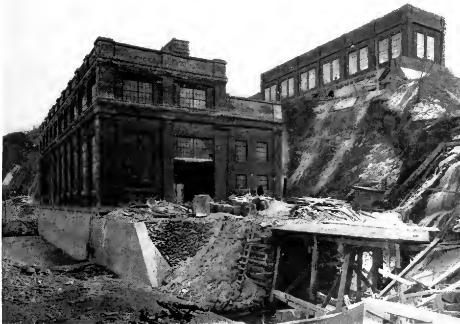
Fig. 4. Exterior View of Power House and Gate-house
