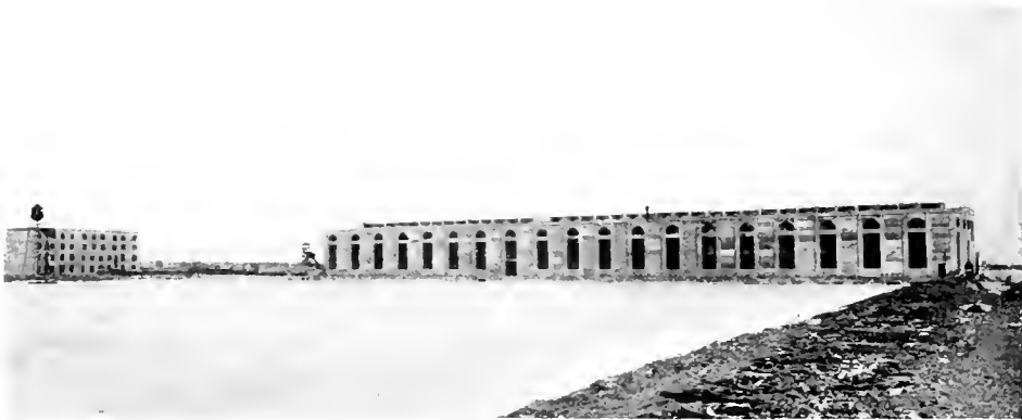
Fig. 4. Cedars Rapids Manufacturing & Power Company on the St. Lawrence River at Cedars Rapids, Canada. Exterior View of Power House with Transformer and Switch House on the Left
