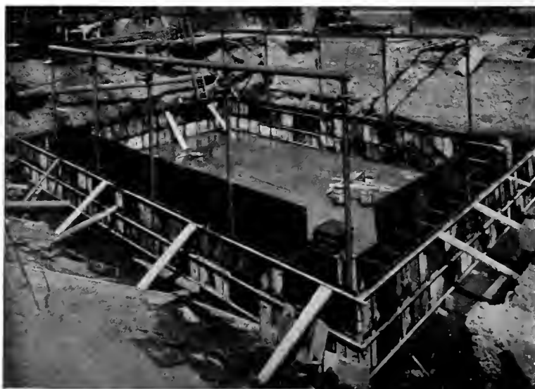
Fig. 1. Lower Forms for Impregnating Pit Walls set in place
