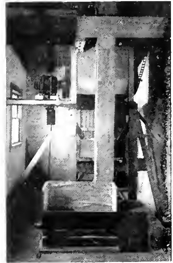
Fig. 4. 5-h.p., 60-cycle, 220-volt, Three phase, 1200-r.p.m. Motor Driving Flour Sifter
