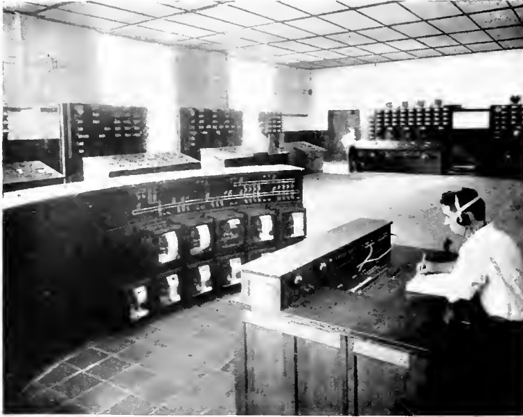
Fig. 4. Control Board and Switchboards of the Keokuk Hydro-Electric Power Station
