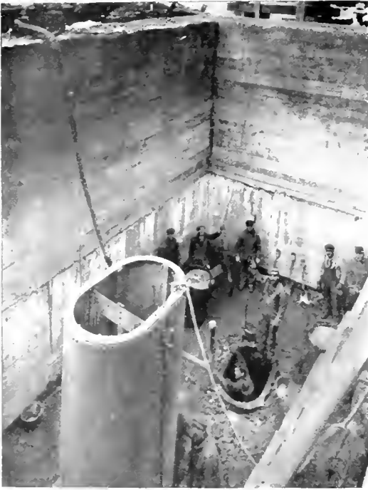
Fig. 3. View of the Tank in place within the Pit
