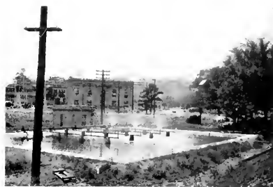
Fig. 14. A View of the Magella Substation and Cooling Pond
