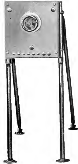
Fig. 1. Field Rheostat Panel
