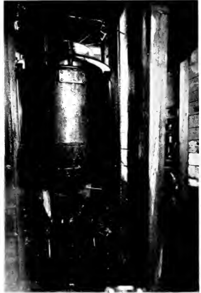
Fig. 6. This same pump in operation just opposite the Relay Pump Station at the 470-ft. level
