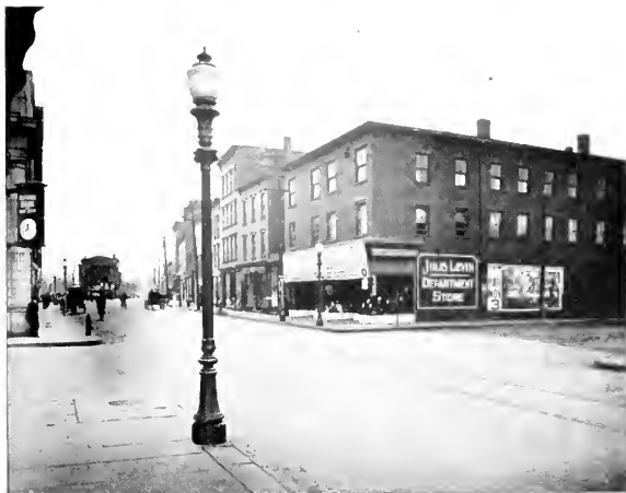
Fig. 2. Day View in Port Jervis, showing Novalux Units equipped with 600-c.p., 20-amp., Edison Mazda Series Lamps
