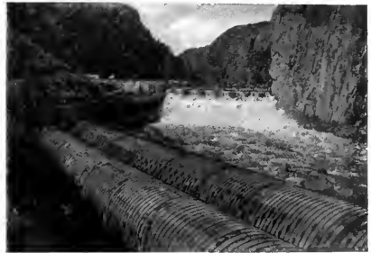
Madison River Dam, 34 ft. High and Stave Penstocks 12 ft. Diameter
