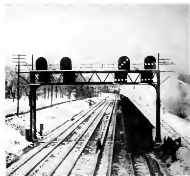
The electric signal over the right-hand track reads "Stop." This means that the westbound train here shown, near Rosemont, Pa., has just entered a "block" of 3500 feet in length. The signal will remain at "Stop" until the train enters the next block, when it will go to "Caution" with the diagonal, instead of vertical, row of lights lighted on the upper half. On the adjoining westbound track, shown in the picture, the signal reads "Proceed," which means that at least three blocks ahead are clear. This picture gives a good view of the overhead conductors which will be used when the electric trains are operated.
