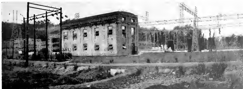
Fig. 16. A Panoramic View of the Magella Substation and Outdoor Equipment
