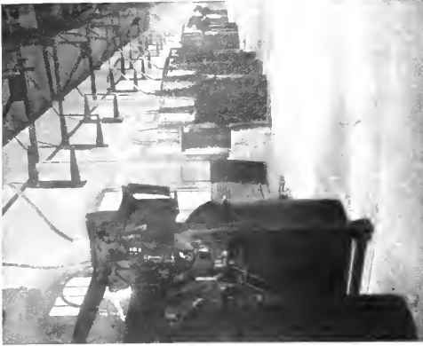
Fig. 15. Butte Substation Showing 100,000-volt Line Switches
