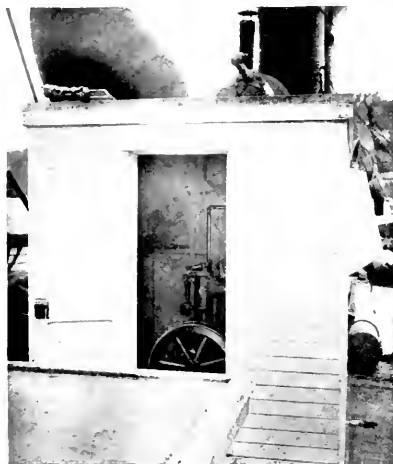
Fig. 5. Oceanic Steamship Company S. S. Sierra with 5-kw. Gasolene-electric Set as Auxiliary Wireless Power. Set Installed in Auxiliary Power House
