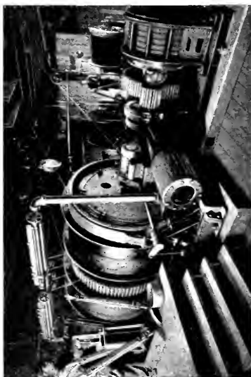
Fig. 12. The Hoist Room of the Penrose Shaft
