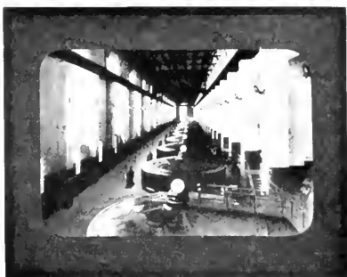
Lantern Slide—Lecture No. 14. Generators in Hydroelectric Plant at Keokuk, Ia.
