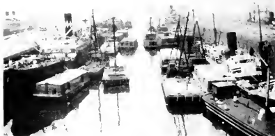
Fig. 10. Floating Cranes Alongside Ships. New York Harbor
