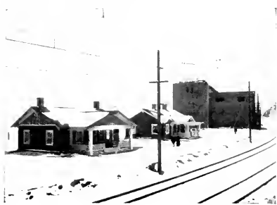
Fig. 6. Janney Substation showing Bungalows for Housing Substation Operators
