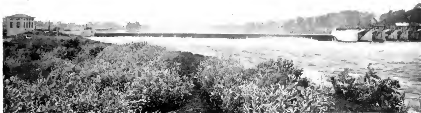
Fig. 5. Dam across Hudson River, Lock 1, Champlain Canal, Waterford, N. Y., showing Taintor Gates on the right and Power House on the left
