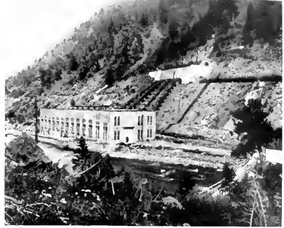
Madison No. 2 Power House and Regulating Reservoir 110 ft. Head, 10,000-kw. Capacity
