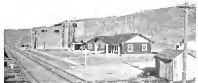
Fig. 17. Morel Substation on the Chicago, Milwaukee & St. Paul Railway
