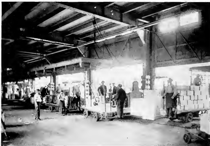
Fig. 19. Electric Freight Trucks Plying between Drays and Steamer's Deck
