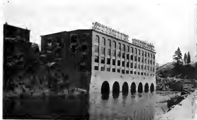
Thompson Falls Station, 30,000 kw. in Six Units
