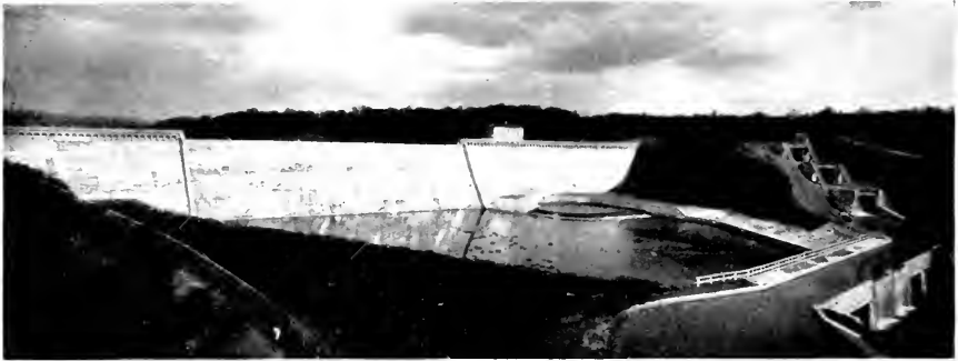
Fig. 44. View of Dam at Delta Reservoir showing Flight of Locks of the Relocated Black River Canal
