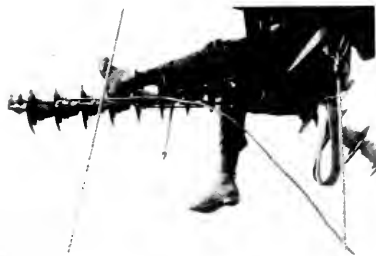
Fig. 12. View Showing the Use of a Turnbuckle to Apply a Strain
