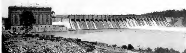
Fig. 2. Lock 12 Dam and Power House, the Principal Generating Station
