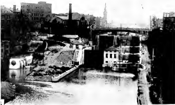
Fig. 39. Locks 34-35, Erie Canal, Lockport, N. Y. New Barge Canal locks on the left, old canal locks on the right, power house in the center
