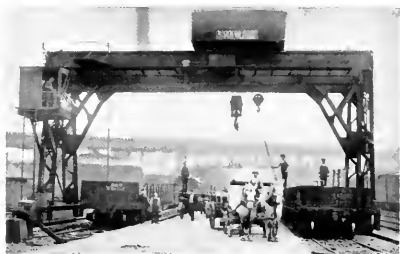
Fig. 11. Gantry Crane in Railroad Yard
