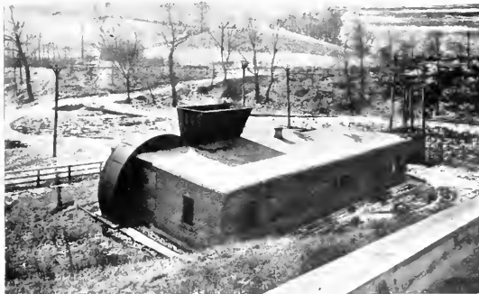
Fig. 29. Fan House of the Pittsburg Coal Company. Polyphase Regulating Sets are employed here for Regulating the Speed of the Mine Fans
