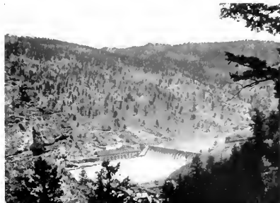
Hauser Lake Development, 60 ft. Head, 18,000-kw. Capacity
