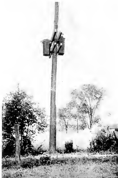
Fig. 15. Installation of a Stationary-coil Constant-current Transformer
