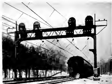
This eastbound train, near Ardmore, Pa., is just passing one of the new automatic electric block signals, which it has set at "Stop." On the adjoining eastbound track, the signal reads "Caution." It means that the 3500-foot block directly ahead is clear, but that there is a train on the next block. The direction to an engineer when the signal is set in the "Caution" position is "Proceed, prepare to stop at next signal."
