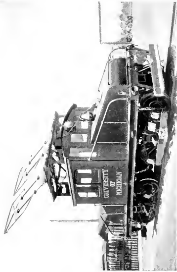
Fig. 12. A 28-ton 600-volt Locomotive Used by the University of Michigan
