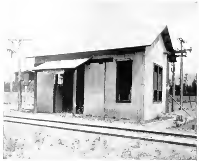
1200-volt Substation at Etiwanda
