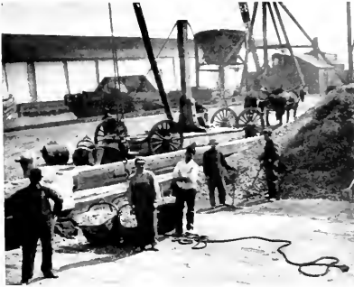
Fig. 1. "Two Horse Power" Tramp Crane Discharging Lighter to Wagons, South St., New York (present practice).
