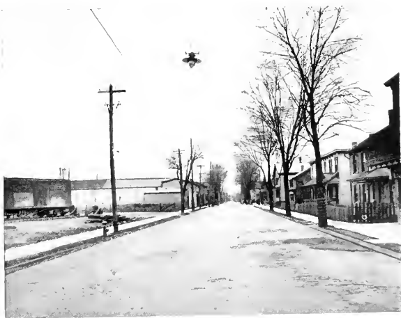
Fig. 3. Day View in Port Jervis, showing an Eye Suspension Unit with 20 In. Concentric Reflector, Prismatic Reflector, and 250-c.p. Edison Mazda Series Lamp
