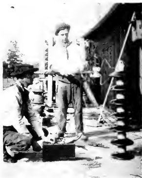
Fig. 10. The Method of Measuring Insulator Resistance with a Testing Fork and Megger
