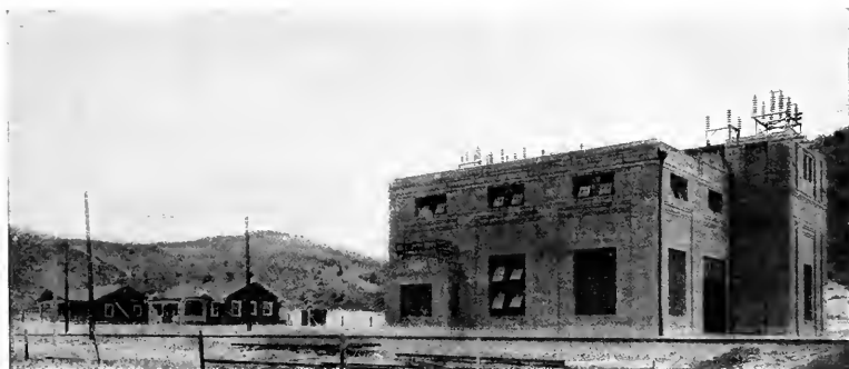
Fig. 1. Substation No. 4 at Eustis
