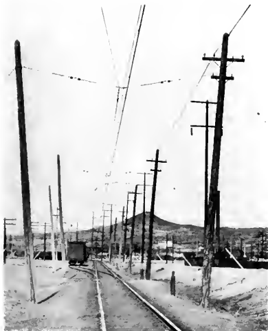
Fig. 4. Overhead Construction at Siding near Butte Yards
