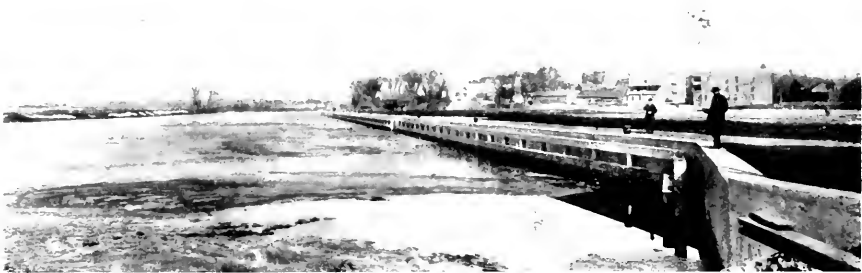
Fig. 45. Barge Canal Terminal, Schenectady, N. Y. Typical of terminals along the canal. At a later date warehouses and loading and unloading machinery will be installed
