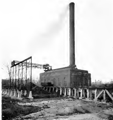
Fig. 3. The Gadsden Steam Turbine Generator Station
