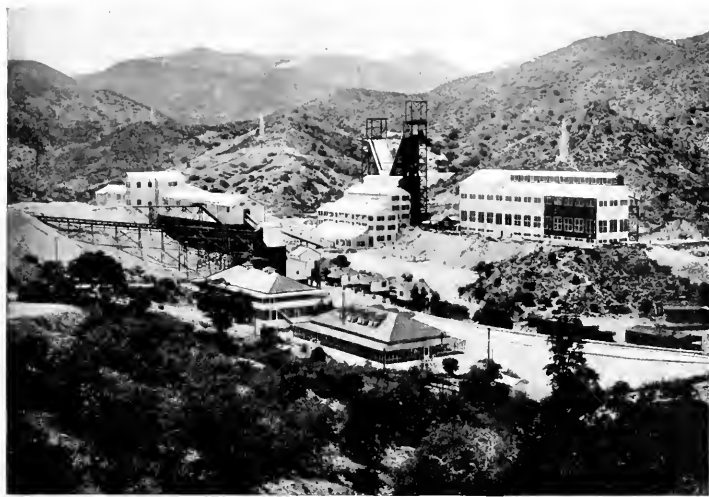
Fig. 4. Main Shafts, Compressor House, Coarse-Crushing Plant and Storage Bins, Inspiration Consolidated Copper Co., Miami, Ariz., During Construction Period
