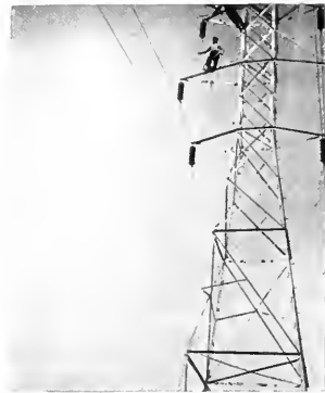
Fig. 11. The Method of Attaching a Hand Ground when Necessary for Testing Purposes
