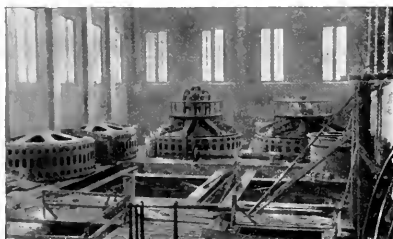
Fig. 5. View in Generator Room showing Installation of 3750 Kw. Units
