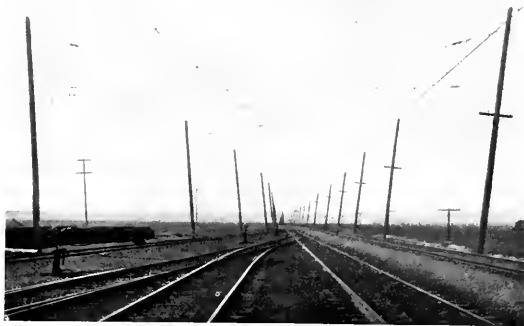
Fig. 5. Typical Overhead Work at the Entrance of Three Forks Yards
