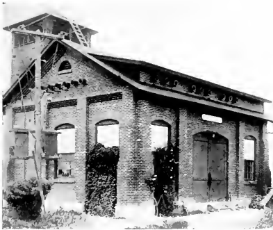
Substation at Vineland
