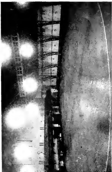
Fig. 1. Night view in the 8th Regiment Armory, N. G. N. Y., Lighted by eight 1000-watt Mazda C lamps in G. E. Novalux Form 1 Fixtures with Opalescent Enclosing Globes.
