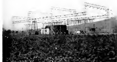
Fig. 4. A General View of the Anniston Substation and Switching Station
