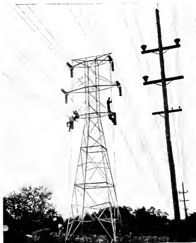
Fig. 9. The Type of Transmission Line Tower Used
