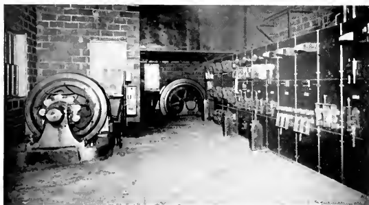
Fig. 3. 500-h.p. Adjustable Speed Induction Rolling Mill Motor with Scherbius System of Control. Union Rolling Mills, Cleveland, Ohio
