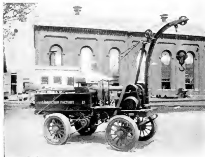
Fig. 5. Storage Battery Crane and Tractor. Hoisting Capacity 4000 lbs. Drawbar Pull 2500 lb.
