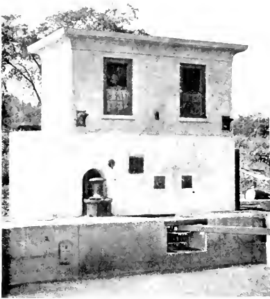
Fig. 32. Typical Concrete Operator's Cabin, Locks 8 to 15 inclusive, Erie Canal
