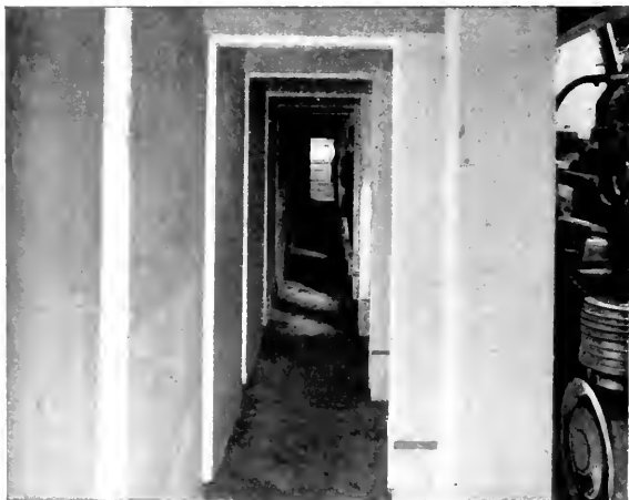
Fig. 5. Showing Passageway on Weighing Side
