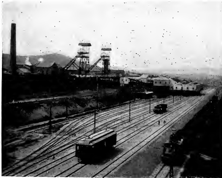
Fig. 3. Oyama Shaft and Screening Plant
