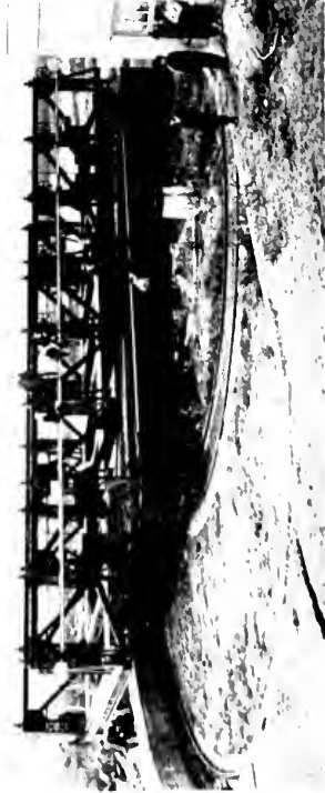
Fig. 9. Turning the Boat Carriage Around on the Turntable
