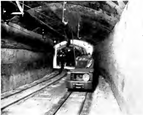
Fig. 16. 8-ton, 24-inch Gauge, 500-volt Locomotive and Train of Ore Cars
