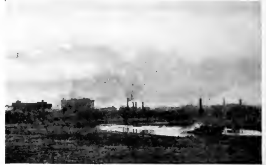
Looking Toward Schenectady Works from State Terminal. Arrow Shows Proposed Location of Slip and Great Crane
