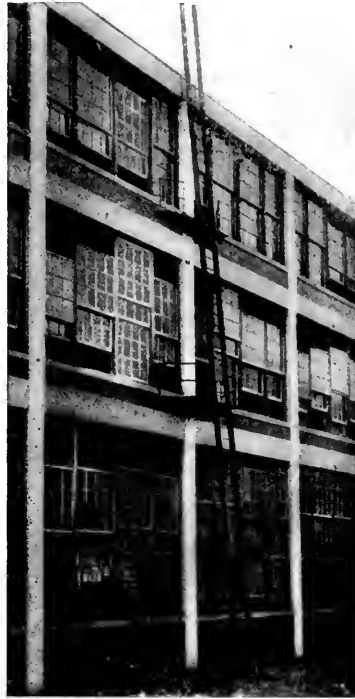
Permanent Fire Ladder Installation
