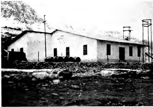
Fig. 4. Substation at Morococha, Peru, Elevation 15,000 ft., Mud Building
