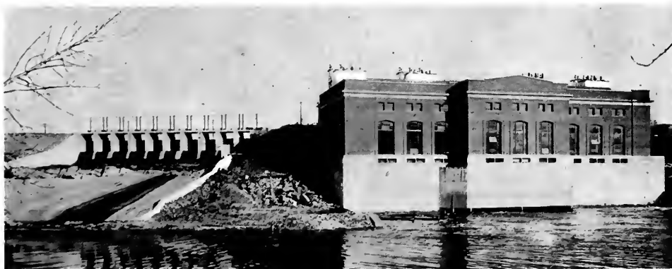
Fig. 3. View of the Power House and Spillway from the River Side
