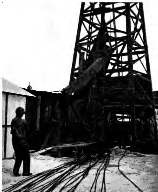
Fig. 2. Pulling rods with motor drive in the Midway field in California
