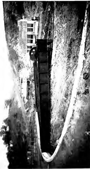
Fig. 7. Turntable, Spring Lake Marine Railway
