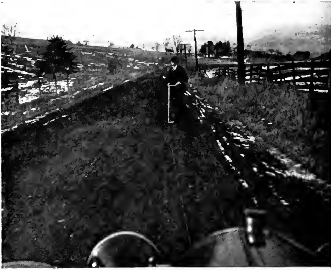
Fig. 2. Type B macadamized state road taken from driver's position
