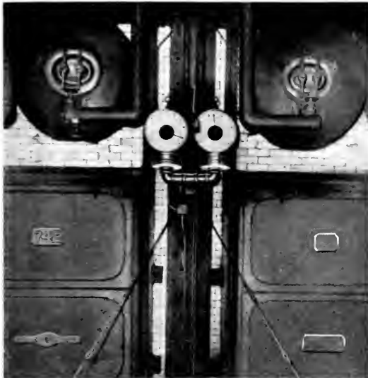
Fig. 3. Two Types of Indicating Steam Flowmeters measuring the steam output of boilers in the Port Morris Station of New York Central & Hudson River Railroad, New York City
