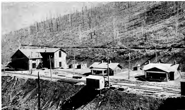
Fig. 4. East Portal Substation with Operators' Bungalows, C., M. & St. P. Station Contains Three 2000-kw. Synchronous Motor-generator Sets
