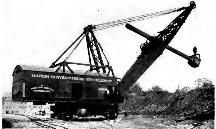
Fig. 19. 250-ton Electric Stripping Shovel in Coal Field at Smithfield, Ohio
