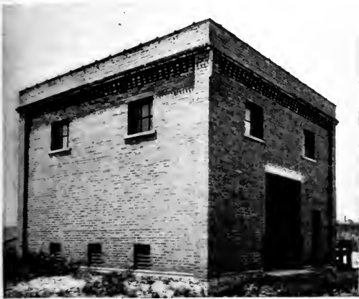
Fig. 5. Automatic Railway Substation (Brennan) Interurban Railway Company, Des Moines, Iowa
