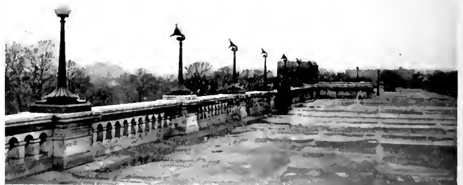
Fig. 3. Flood Lighting Projectors for Illuminating Main Portion of Capitol
