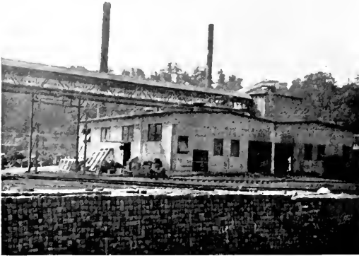
Destructor Plant, showing Overhead Conveyor from Carpenter Shop
