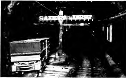
Fig. 22. "Safety-first" Sign to Impress upon the Miners the Importance of Observing Greatest Care in Operating all Equipment
