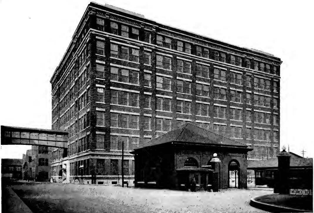
Laboratory and Office Building at Schenectady Works.
