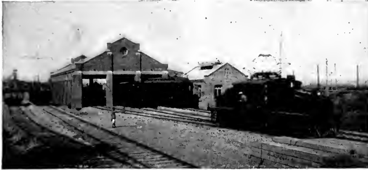
Fig. 2. Locomotive Shed, 45-ton Locomotive and 28-ton Motor Passenger Car
