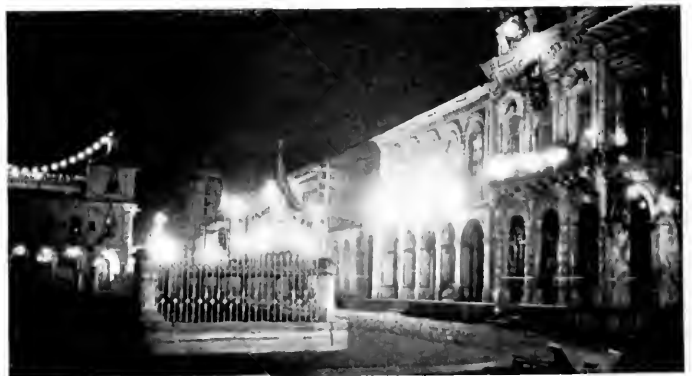
Fig. 14. Special Illumination of Public Buildings
