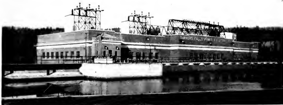
Fig. 2. View of Station from Canal Side
