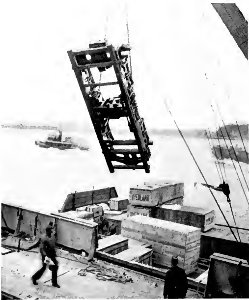
Loading Truck Frame on Steamship Celia
