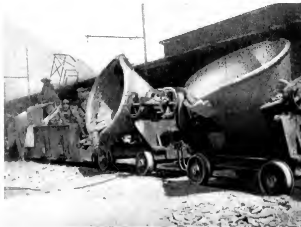
Fig. 6. Electric Locomotive Handling Slag, Casapalca, Peru
