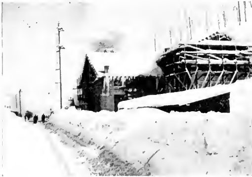
Fig. 1. Substation at East Portal showing Snow Conditions in the Bitter Root Mountains
