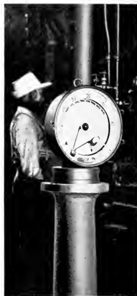
Fig. 2. Indicating Recording Integrating Flowmeter measuring maceration water in the Central Santa Rosa Sugar Mill, Santa Rosa, Cuba
