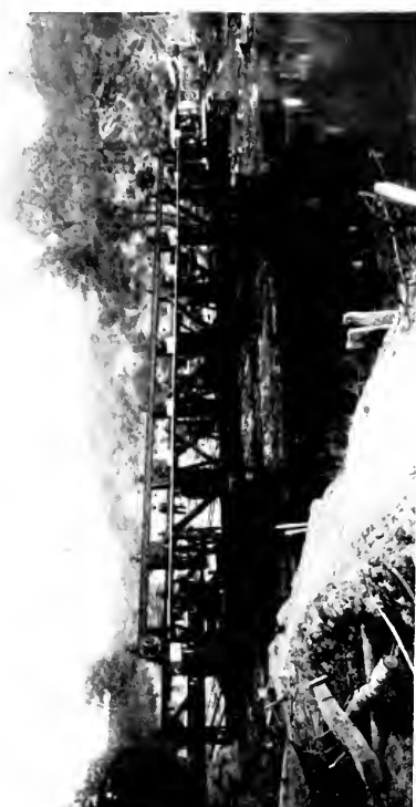
Fig. 6. Boat Carriage going up the Incline on the River Side of the Levee
