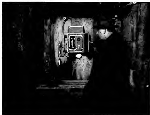
Fig. 26. Installation of Telephone
