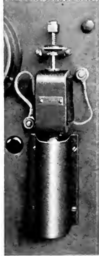
Fig. 11. Time-limit Shunt Relay
