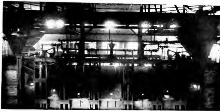
Fig. 6. A 50-ton Open-hearth Furnace Using Pulverized Coal. The Fuel Bins are shown at each end of the Furnace
