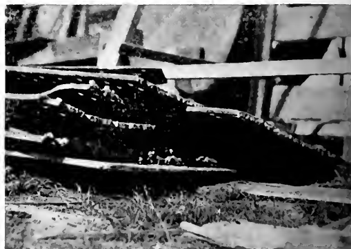
Pile of Scrap Plates Cut by Electric Arc
