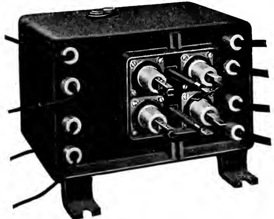
Fig. 10. Bottom Compartment of Oil Switch with Tank Removed to show Oil Circuit Breaker
