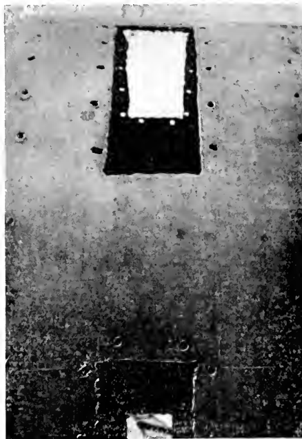
Details of Furnace Shell
