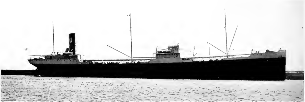
Oil Burning Tanker "La Brae." Driven by 2600-h.p. Curtis Turbine through Alquist Reduction Gear
