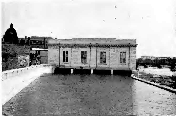
Fig. 2. Forebay Side of the Automatic Generating Station
