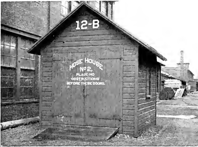
Typical Hose House
