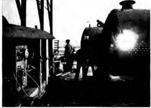
Fig. 12. Welding Oil Stills by Means of Electric Arc
