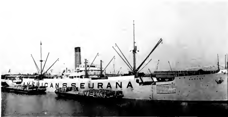
Fig. 1. S. S. Eurana, Equipped with Geared Turbine Propelling Machinery
