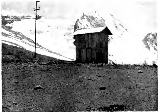
Fig. 7. Lightning Arrester Station at Antacona. Elevation 16,000 ft.
