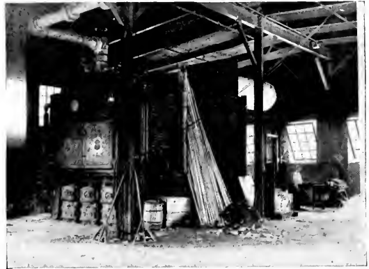
Interior of Destructor Plant Producing 53,000,000 lbs. of Steam a Year
