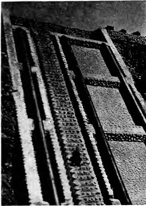
Fig. 11. Near View of Penstocks and Masonry
