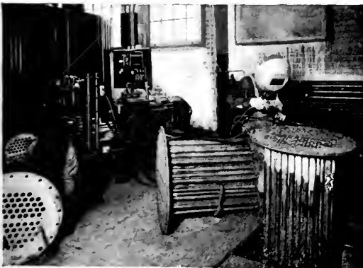
Fig. 13. Welding Air Compressor Intercoolers by Electric Arc Process
