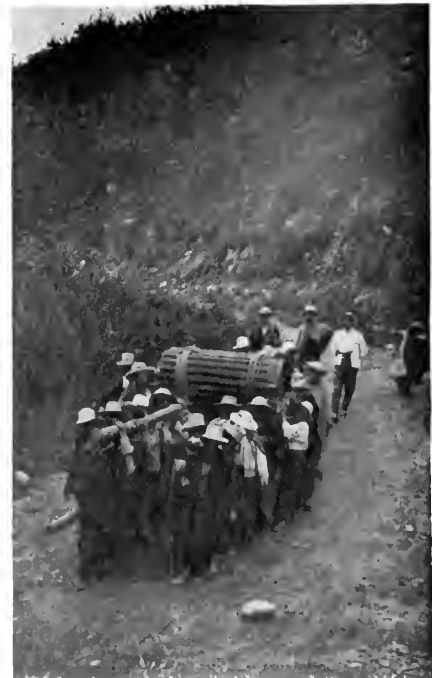
Fig. 2. Transformer Case Secured to Bamboo Poles which are Carried on the Natives' Shoulders. Packages weighing as much as 1000 pounds are carried in this way
