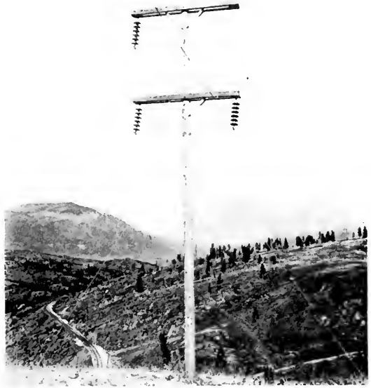
Fig. 4. Standard 100,000-Volt Wood Pole Transmission
