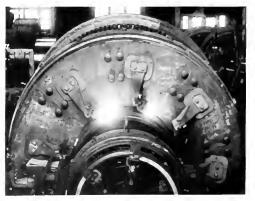
Fig 1. Flashing at Brushes on 1000 km. 1500 vol: Generativ Forming Part of 2000 km, 2000 volt Motor generator Set at Five Times Load, Showing Different Stages of Arc Formation.
