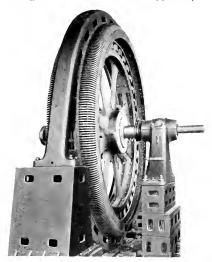
Fig. 4. 6250-kv-a., 6600-volt, 88-r.p.m. Generator for Gas Engine Drive
