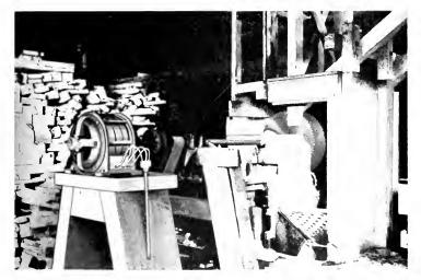
Wood Slasher, for Cutting Slabs into 16 in. Lengths, Driven by a 35-h.p., 1200-r.p.m., 550 volt Direct-connected Motor. Weyethaeuser Timber Company.
