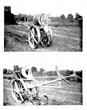
Figs. 2 and 3. Front and Rear Views of Electric Tractor, showing Cable Reel, Control Levers, etc.
