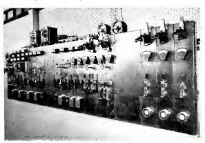
Fig. 34. Switchboard in Motor Room and Sub-station, for 36-inch Reversing Blooming Mill, Ashland Iron Mining Company, Ashland, Ky
