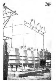
Fig. 8. Oxide-film Lightning Arrester for Outdoor Service Installed on a 33,000-volt Circuit
