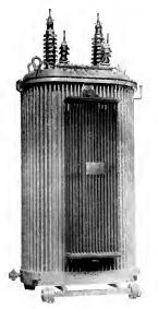
Fig. 54 Combination Radiator and Corrugated Type Tank
