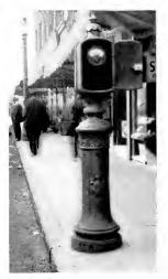
Fig. 7. Control Pedestal for 100 kv-a., 550-volt, 60-cycle, Three-phase Subway Static Condenser. Lynn Gas & Electric Company
