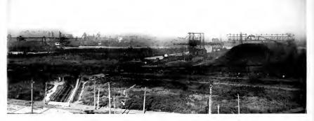
Fig. 5. View of Coal Storage Pile at South Chicago. Both steam and electrically operated unloaders and electrically operated stocking bridge are shown. There is sufficient storage area to care for 300,000 tons of coal
