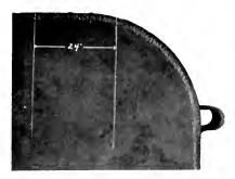
Fig. 5. Near View of Arc Weld in Base of Large Tank
