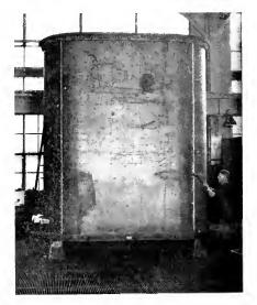
Fig. 14. Large Tank in Regular Test for Leaks. It is filled with water and allowed to stand for 48 hours. This tank with 90 ft. of welding did not develop a single teak. While filled with water the seams are given sharp blows throughout their length with a five-pound hammer
