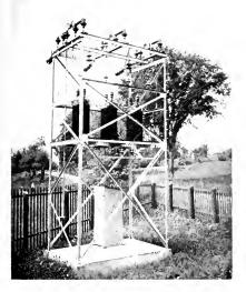
Standard Outdoor Substation, steel structure mounted, three-phase, 60 cycles, 33,000 volts high tension, 2300 volts low tension, 150 kv-a.
