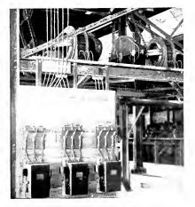
25-h.p. Back-geared Motors Driving Main Bagasse Conveyors, Central Delicias. The motors are mounted directly under the conveyor while the starters are on the operating floor below
