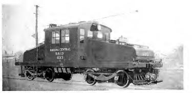
60-ton Trolley Type Electric Locomotive for Bringing in Cane Trains from the Fields
