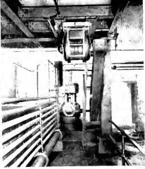
25 h.p. Motor Driving Refrigerating Machine 5 - Keep Down Reaction Temperatures at National Applies & Chemical Company, Buffalo, N.Y.
