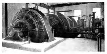
Fig. 20. 1800-h.p. Hoist Motor Driving First Motion Double-cylindrical Hoist, Elm Orlu Mining Company, Butte, Mont.
