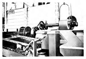
Lath Bolter Driven by a 50-h p., 1800-r.p.m, 500 volt Direct connected Motor Weyerhaeuser Timber Company
