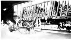
Motor operated Side Tilting Car Platform, Central Ulacia, Cuba. The control is located on the opposite side with the operator
