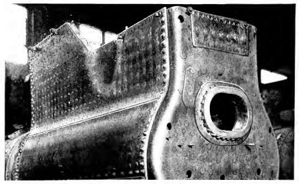
Fig. 7. Loconotive Boiler Being Changed to Stationary Type, New Half Side Sheets and Patch in Door Sheet; Work Done by Electric Arc Welding
