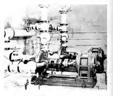
35-h.p. Induction Motors Driving Supply Water Pumps in the Pump House at Central Chaparra
