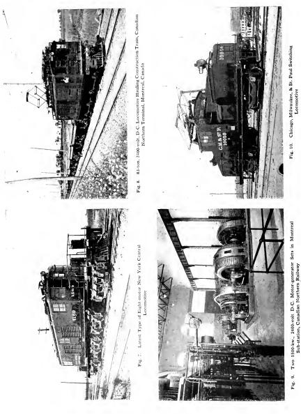
The substation, located at the portal of the 3-mile tunnel under Mt. Royal, was entirely completed, and contains two 3-unit, 2400volt motor-generator sets with a capacity of 1500 kw. each (Fig. 9). Energy is purchased from the Montreal Light, Heat, and Power Company at 11,000 volts, 60 cycles, 3 phase, and transformed by these units to 2400 volts d.e. for the electric zone.
