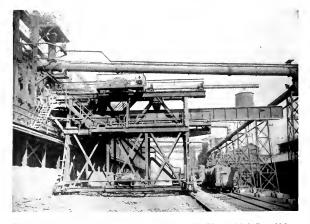
Fig. 8. A Coke Pusher. This plant is located on the Ohio River and is built on high foundations to avoid damage from floods. This accounts for the height of the structural supports under the real operative part of the pusher
