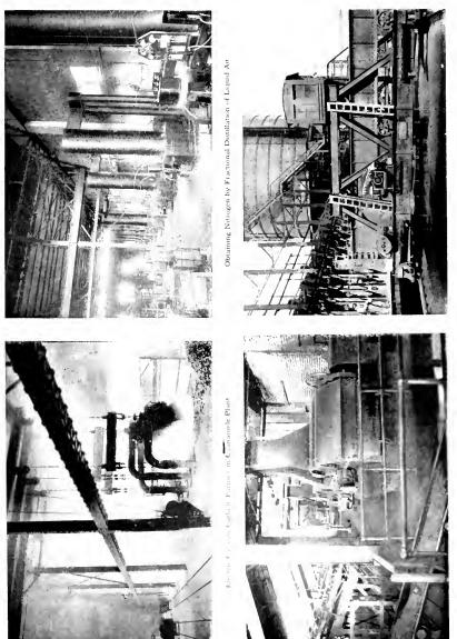
Motor operated Traveling Coke Pusher at Indi ina Steel Compuny. Gary, Ind which discharges coke from ovens into a quenching car
