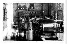
Two 500-kw., 480-volt, Alternating-current Curtis Steam Turbine Generators. Central Agramonte, Cuba
