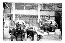
Power Plant, Central Lequeitio, Cuba. Two 300-kw., 480-volt, Alternating-current Curtis Steam Turbines with Qil Engine and Electric Motor-driven Exciters. The Qil Engine Driven Exciter is Used for Lighting in the Dead Season
