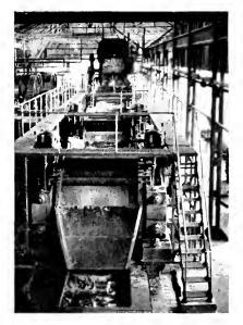
Fig. 35. Typical Cane Crushing Rolls in Sugar Mill
