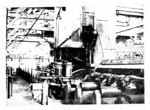
7-ft. Vertical Resaw Driven by a 75-h.p., 550-volt Slip-ring Induction Motor. Weyerhaeuser Timber Company
