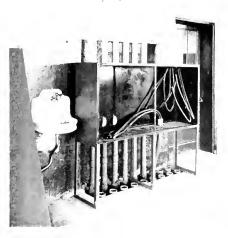
Fig. 9. Typical Floor Power Riser Junction
