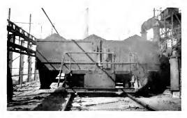
Fig. 7. A Charging Car in Position for Discharging its Load of Coal Into an Oven
