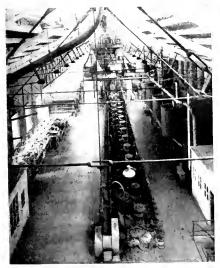
Fig. 7. Cell Floor showing Diffusion Cells and Cossette Conveyor in the Center with Heaters, Filter Presses, and Carbonation Tanks at the side. American Beet Sugar Company, Chino, Cal
