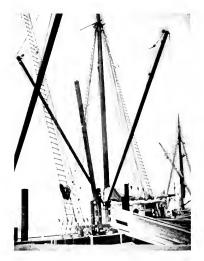
Fig. 9. Long Timber Suspended in Position Preparatory to Lowering
