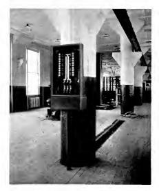
Fig. 24. Standard Lighting Panel Board
