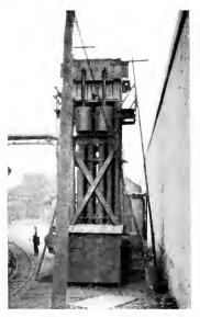
Fig. 44. Experimental Precipitator Used in Electric Precipitation of Coal Smoke-Voltage On
