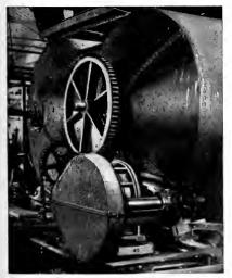
35:h.p., 600-r.p.m. Back-geared Motor Driving Open Crystallizers, 1150 Cu. Ft. Bach, a Magma Conveyor and First and Second Magma Pumps. Central Santa Rosa. The motor is mounted out of the way on a platform of the closed crystallizers shown
