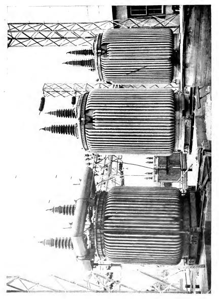
Before the changes were made the frame and base of the constant current transformer were made up of castings held together by steel rods and nuts, and the form-wound coils were heavily insulated. The initial improvement, which occurred in 1916, eliminated the castings by the substitution of angle iron for frame and base, effecting a reduction of about 20 per cent in weight. A protective casing of extruded metal or wire net was also made part of the regular equipment.
