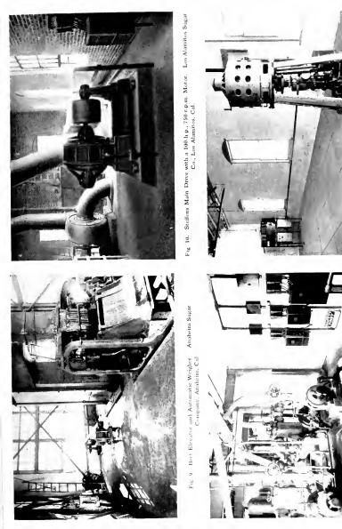
Fig. 12. 150-h.p., 750-r p.m. Squirrel-cage Vertucal Motor Direct-coupled to a Deep Well Water Supply Pump. Anaheim Sugar Company, Anaheim, Cal.
