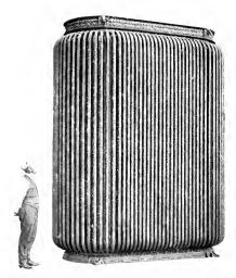
Fig. 13. Finished Tubular Tank with Base, Seams, and Tubes Welded
