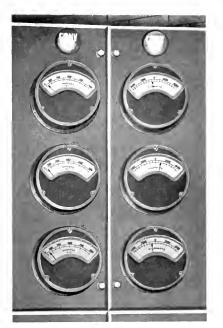
Fig. 11. Indicating Meters Connected in Balancer Circuit. Converter Set Balancing to Extent of 1000 kw.
