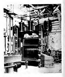
12-in. by 42-in. Gang Saw Driven by a 10-h.p., 550-volt, Slip-ring Induction Motor, Weyerhaeuser Timber Company
