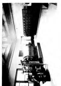
Fig. 2. Power Plant Consisting of One 750-kv a., 3000-f p.m., 480-volt Alternator with Direct connected Exciter, Divien by a Non condensang Curis Steam Turbine. Switchboard consists of one generator and exciter panel, six feeder curcut panels and two lighting panels. Anaheim Sugar Company, Anaheim, Cal.
