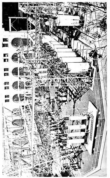
Partial view of a typical large size outdoor substation (60,000 volts high tension, 2400 volts low tension) including outdoor power transformers, oil circuit breakers, lightning arresters, disconnecting devices, and bus structure. Outdoor substations are equipped with apparatus successfully operative under any climatic conditions and can be built in any capacity. (See page 640.)
