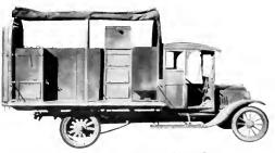
Fig. 1. Automobile Electric Kitchen showing Chycking Compartments and Water Tank, at rear, M united on Truck Platform
