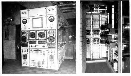
Fig. 7 Voltage and Phase-balancer Regulator Switchboard
