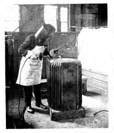
Fig 19. Use of Carbon Electrode with Metal Filler when Welding <sup>1</sup><sub>1</sub>, in Steel Bases to the Edges of Crushed Corrugations
