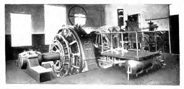
Fig. 22 1400 h.p. Motor driving First Motion Heist at Mine No. 80, Consolidation Coal Company, Fairmont, West Virginia Dupheate Equipment at Mine No. 87
