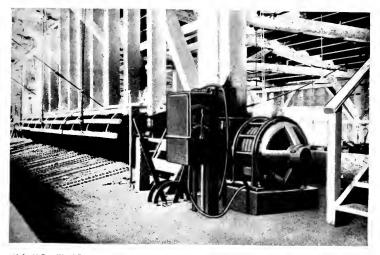
42-ft. 10-Saw Wood Slasher for Cutting Slabs into 4-foot Lengths for Fuel. It is Driven by a 75-h.p., 550-volt Direct-connected Motor. Weyerhaeuser Timber Company, Everett, Wash.
