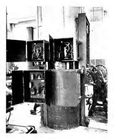
Fig. 18 Controllers on Columns
