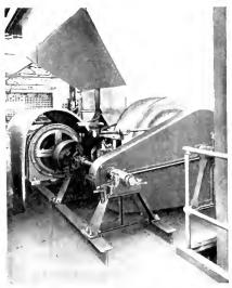
Fig. 6. Beet Sheers Driven by One 60 h p. 750 r p.m. Squirrelcage Motor through Friction Clutches and Chain Drive Anaheim Sugar Company, Anaheim, Cal
