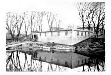
Fig. 5. The Concrete Boathouse on the Banks of the Mohawk River in the Rear of Edison Club and Hall. A double track is provided for running the 200 cances in and out of the fireproof boathouse
