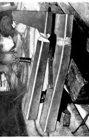
Fig. 9. Two Steel Stem Forgungs, One of Which Has Been Electrically Welded and the Other is Ready for Welding
