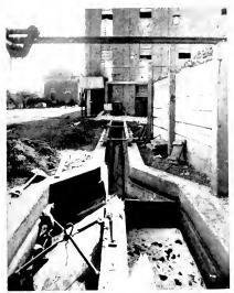
Fig. 5. Beet Flume showing a Dalton Weed Separator at the Entrance to the Building. A Motor Operated Hoist Removes the Crib with the Weeds and Trash. Anaheim Sugar Company, Anaheim. Cal
