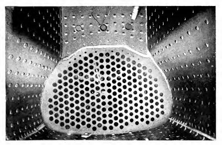
Fig. 6 Interior of Locomotive Fire Box, Back Tube Sheet Welded by Arc Process
