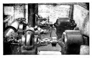
Two 100-h.p., 1200-r.p.m. Motors Driving 4500-gal.-per-min. Injection Water Pumps. Central Santa Rosa
