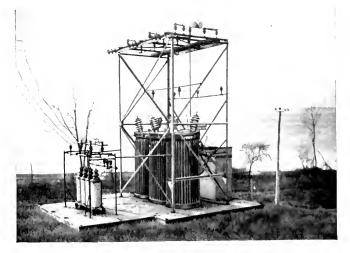
Standard Outdoor Substation, steel structure mounted, three phase, 60 cycles, 22,000 volts high tension, 440 volts low tension, 750 kv a
