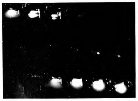
Fig. 32 High spot Photograph of Short Circuit on 500 km, 600 volt, 60 cycle Synchronous Converter Protected by Flash Barriers and Standard Circuit Ercakei after Arrangement of Brush Rigging has been Changed – Uniform distribution of flashing PROTECTION FROM FLASHING FOR DIRECT-CURRENT APPAPATU - - -
