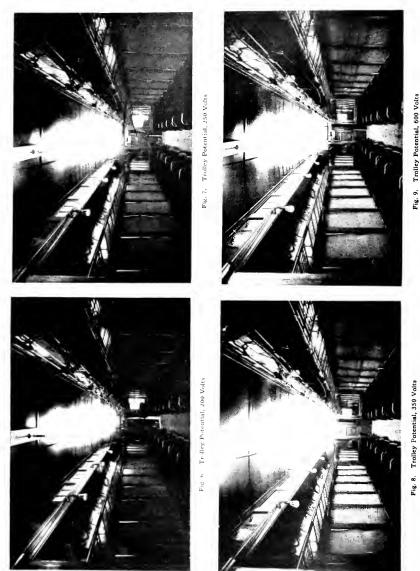
Photographs showing Maintenance of Satisfactory Lighting by Motor-generator Set, with Varistion in Trolley Potential from 200 to 600 Volts
