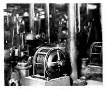
15-h.p., 600-r.p.m. Motors Geared to Triplex Plunger Molasses Pumps. Central Mercedes
