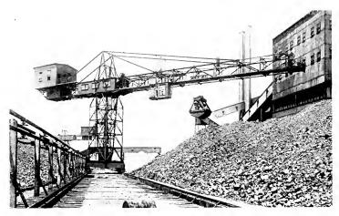
Fig. 27. High Speed A-C. Hammer Head Coal Handling Gantry Cranes
