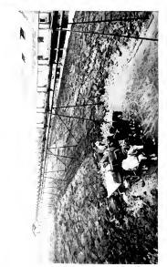
Fig. 15. Pulp Silo showing the Outgoing Pulp Line, the Strainer Tower and the Return Water Pipe. Los Alamitos Sugar Company, Los Alamitos, Cal.
