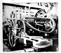
15-h.p. Back-geared Induction Motor Driving a Cane Crushing Roll for Turning Off the Surface Central Mercedes
