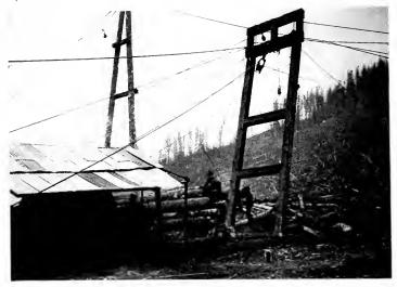
Electric Logging Engine, showing Main Supporting Tower for Sky Line and Loading Boom, operated by 150-h.p., 550-volt Siip-ring Induction Motor. Potlatch Lumber Company, Elk River, Idaho (A Sky Line is an overhead tramway for getting loga across a canyon)
