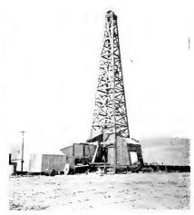
One of the Heaviest Derricks in the World, in the Fig. 2. Coalinga Field, California. Height 106 ft. Depth of well 4200 ft.
