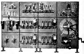
Main Control Panel for 200-h.p. Variable Speed Induction Motor for Driving Cane Crushing Rolls
