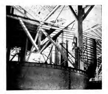
Open Wiring in an Existing Mill Horizontal lines are carried on insulators and anchored by turn-buckles. Vertical connections are made through iron conduit to the control apparatus
