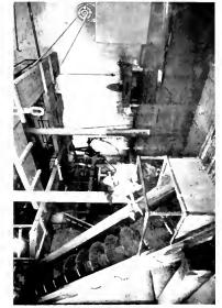
Eq. 4 Beet Serew for Elevating the Beets from the Flume to the Washer the top American Beet Sugar Company, China, Cal.
