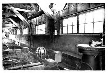
10-h p., 1200 r.p.m., 440-volt Motor Driving the Set Works on the Log Carriage. The Sliding Cable to the Motor is shown along the Right Wall Booth Kelly Lumber Company
