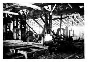
50-h.p. Motor Driving a Rip Saw and a 25 h.p. Motor Driving a Planer and Woodworking Tools in the Carpenter Shop. Central Delicias
