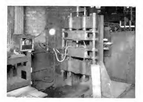
Fig. 1. Electric Welding Machine of 36 Tons Pressure Capacity and 100,000 Ampere Current Capacity, Built to Determine the Pratticability of Spotwelding Heavy Plates. The transformer (at the right) furnishes the welding current, and the meters in the box (at the left) were used while making the initial welds to record the values of current, pressure, and time
