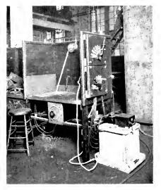
Fig. 2. Alternating-current Welding Transformer
