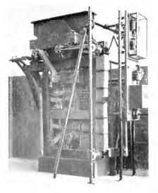
Fig. 4. High-speed Circuit Breaker Installed in Substation
