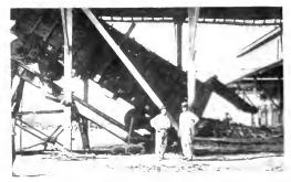
Hydraulie Car Unloader. Central Mercedes - A metor driven centrifugapump replaced the steam pump for supplying the water
