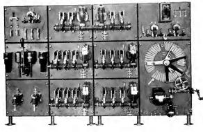
Fig. 36. Main Control Panel for 200-h.p., 440-volt, Three-phase, 45–65-cycle Variable Speed Induction Motor for Driving Cane Crushing Rolls
