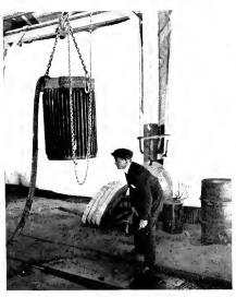
Fig 21. Tanks are Given a Static Water Test for 36 Hours and Then Carefully Inspected for Leaky Joints
