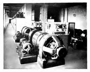
Fig. 9. Boosters and Exciters of Regulator System
