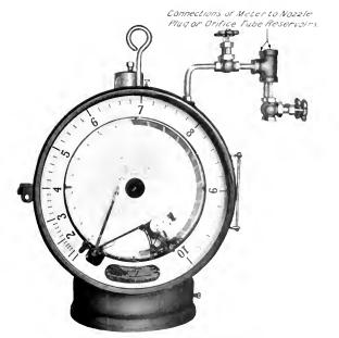
Fig. 6. Indicating Recording Integrating Flow Meter
