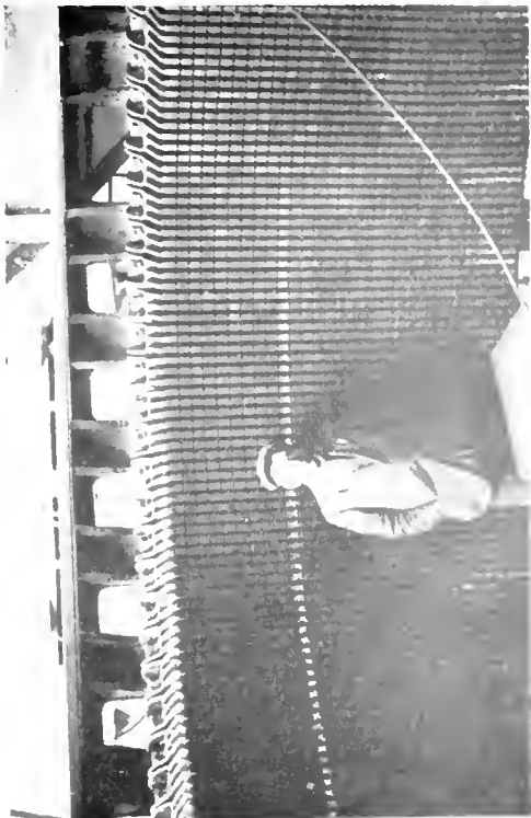
Fig. 32. Rotor of 32,500 kv. a. Waterwheel Generator Being Erected in Power Station
