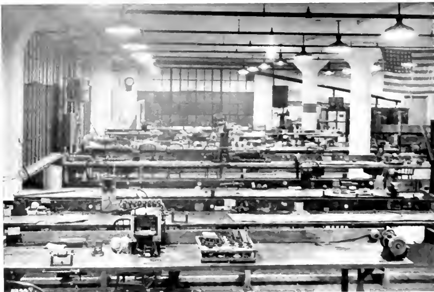
Fig. 6. A Modern Lighting Installation in an Armature-winding Room. RLM Standard Dome Reflectors and 300-watt Bowl-enameled Lamps. Spaced 10 by 12½ feet. Mounted 11 feet above floor. Average illumination obtained, 17 Foot candles.
