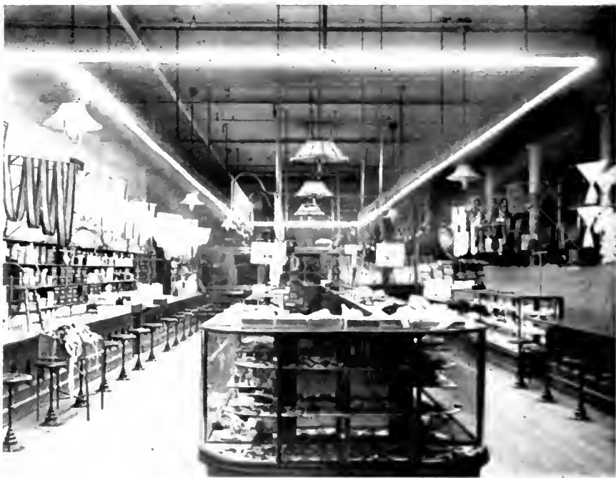
Fig 9 Installation of Low voltage "Long tube" Nitrogen Conductor Lamps
