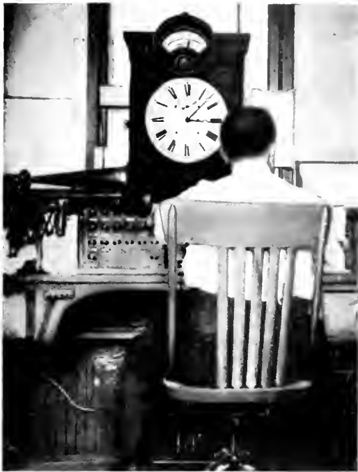
Fig. 9. Photograph Showing Indicating Kilowatt Totalizer in the Trick Dispatcher's Office
