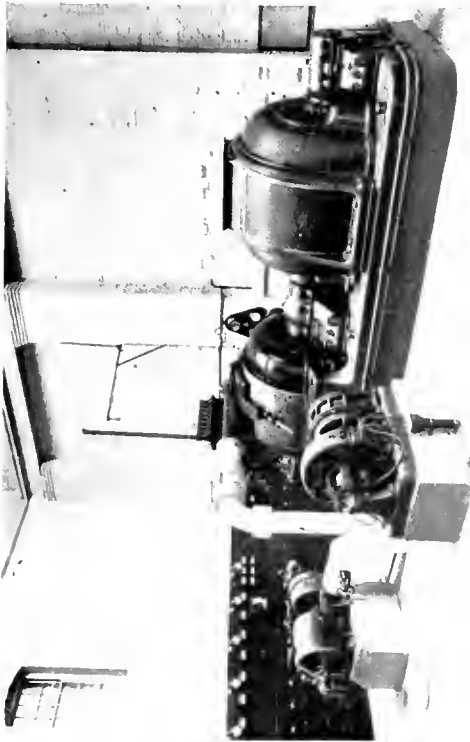
Fig. 1. Motor-driven and Turbine-driven Exciter Sets, together with a 3000-kw. Curtis Steam Turbine Generator
