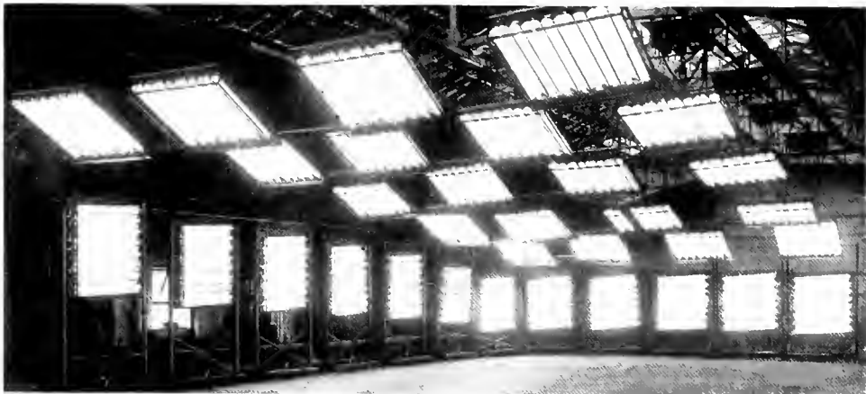
Fig. 17. Banks of the Cooper Hewitt Lamp on the Metro Motion Picture Stage
