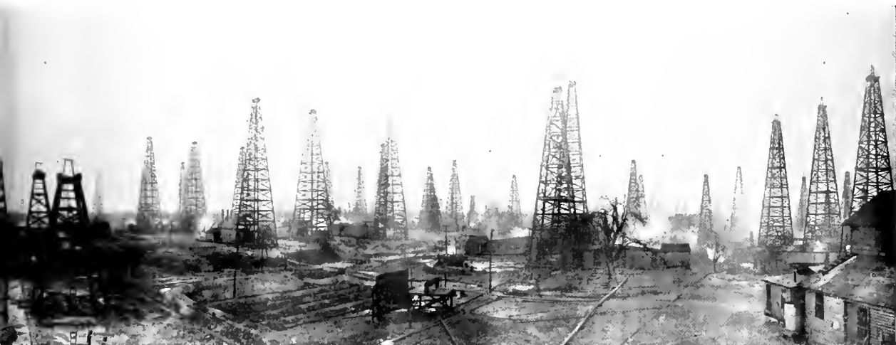
Wells are Now Pumped by Two-speed Oil Well Motors
