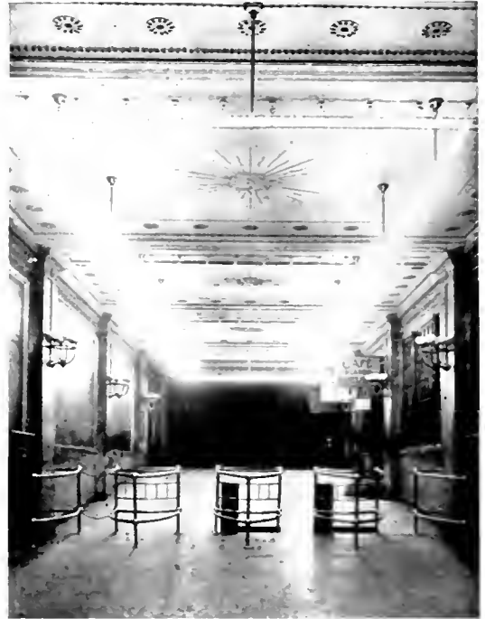
Fig. 10. Lobby of Madison Square Garden Illuminated with Low-voltage "Long-tube" Lamps
