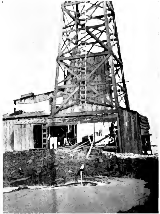
Fig. 12. Pumping 450 Barrels of Oil a Day From a Depth of 1900 ft. with a Two-speed Oil Well Motor in the California Midway Field
