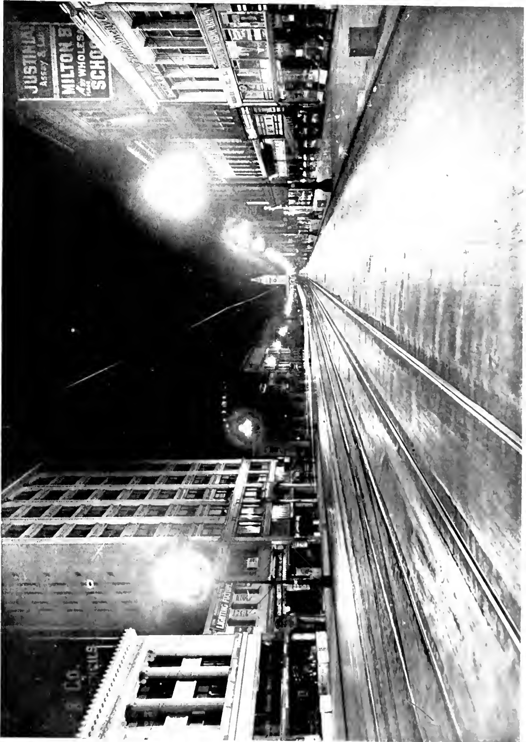
Fig. 3 - Market Street, Looking Toward Ferry Building, San Francisco, Cal., Intensively Lighted by 6.6 amp Ornamental Luminous Arc Lamps
