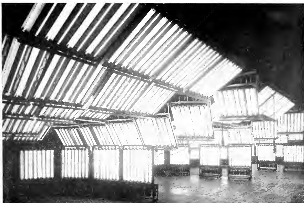
Fig. 11. Installation of Cooper Hewitt Lamps in a Motion Picture Studio
