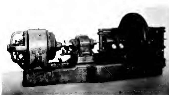
Fig. 1. 50 kw. High Frequency Alternator Installed at the New Brunswick Radio Station
