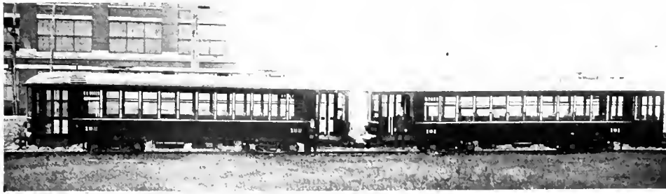
Fig. 2. Two-car Train, Low-wheel, Light-weight Cars, Buffalo and Lake Erie Traction Company
