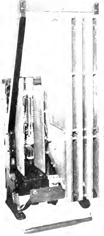
Fig. 6. Disconnecting Switch and Line Contactors. The knife blade switch makes it possible to test the control apparatus without applying power to the motors. The magnetically operated line contactors break the motor circuit both when the master controller is turned off and when an overload occurs
