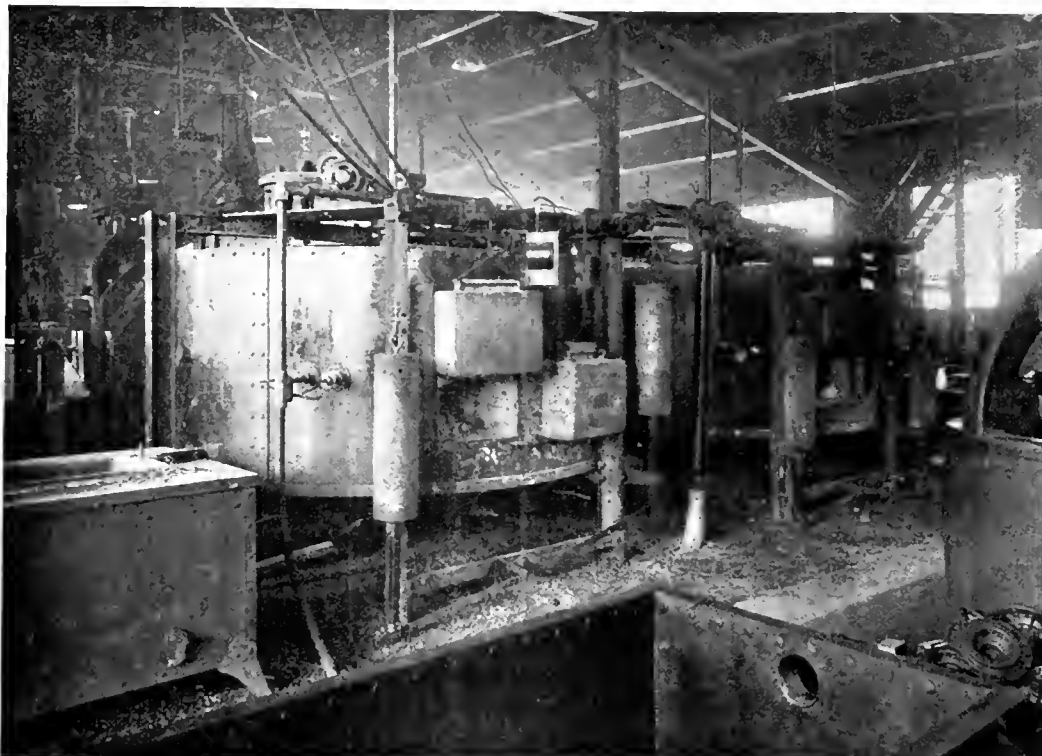
Fig. 11. Rotary Annular Ring Furnaces for Treating Gears and Similar Parts
