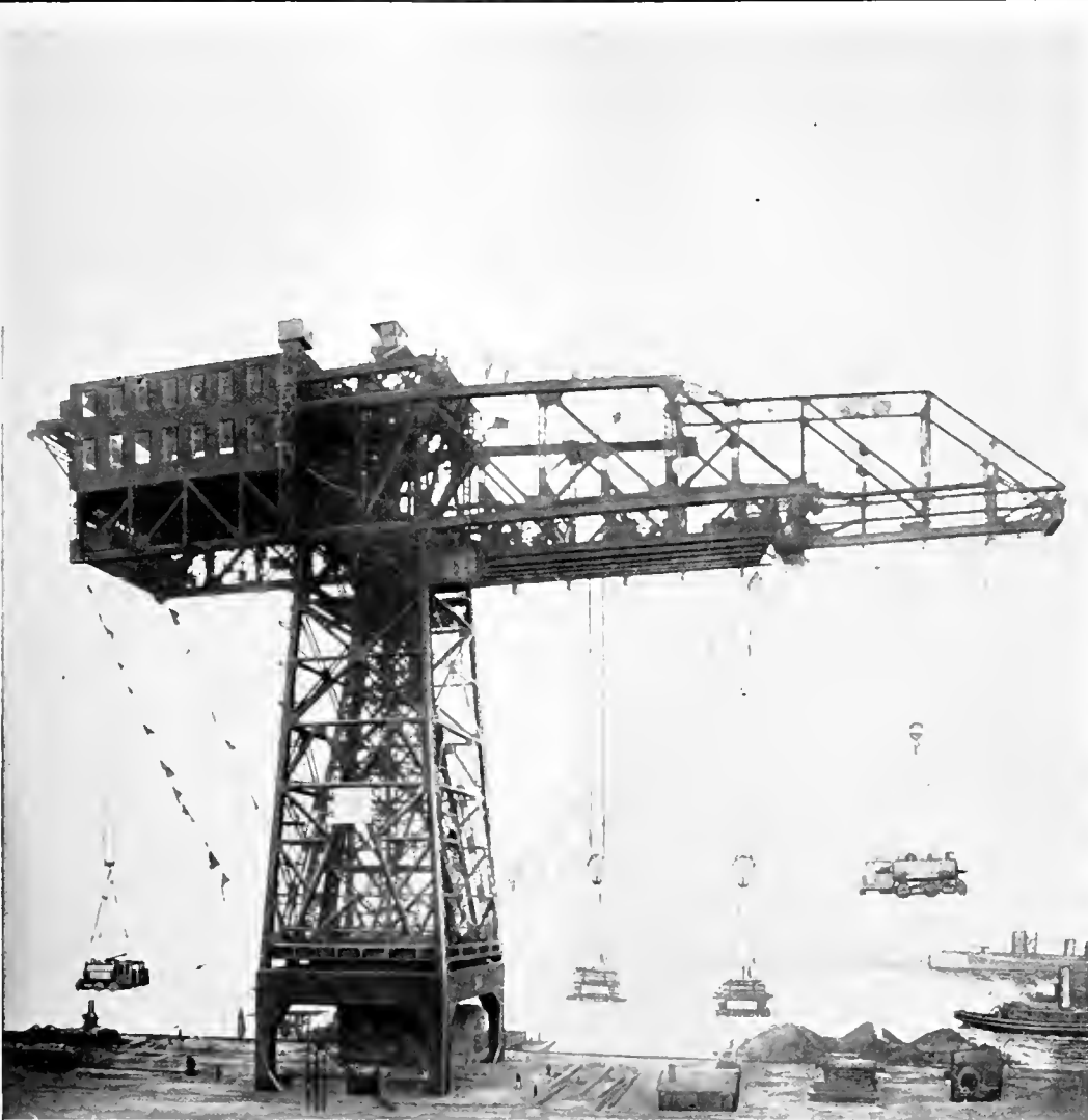
The Largest Hammer Head Crane in the World, Located at League Island Navy Yard, Philadelphia, Lifting a Load of 1,010,000 Lb. From left to right the loads are, respectively: Switching Locomotive, 78,000 Lb.; Two Loads of Steel Shapes, 416,000 Lb. each; Locomotive, 100,000 Lb. Total horse power of motors, 530
