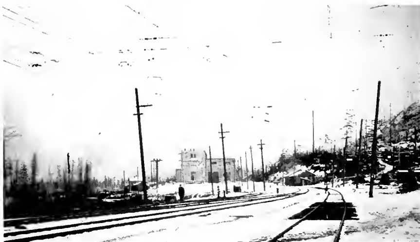
Fig. 14. Overhead Construction Looking East Toward Cedar Falls Substation
