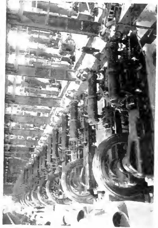
Fig. 15. Synchronous Motors Driving Air Compressors, U. S. Air Nitrates Corp., Muscle Shoals, Ala.
