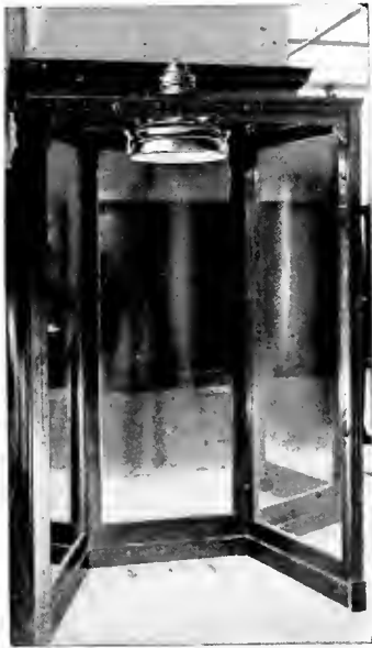
Fig. 5. A Color Identification Unit Placed Above the Triplicate Mirror in a Clothing Establishment. Confidence in purchasing garments is much greater when artificial daylight is available
