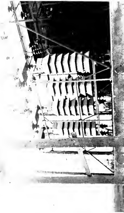
Fig. 4. A Close-up View of the Oxide-film Lightning Arrester, Located on the Concrete Platform as Shown in Fig. 2
