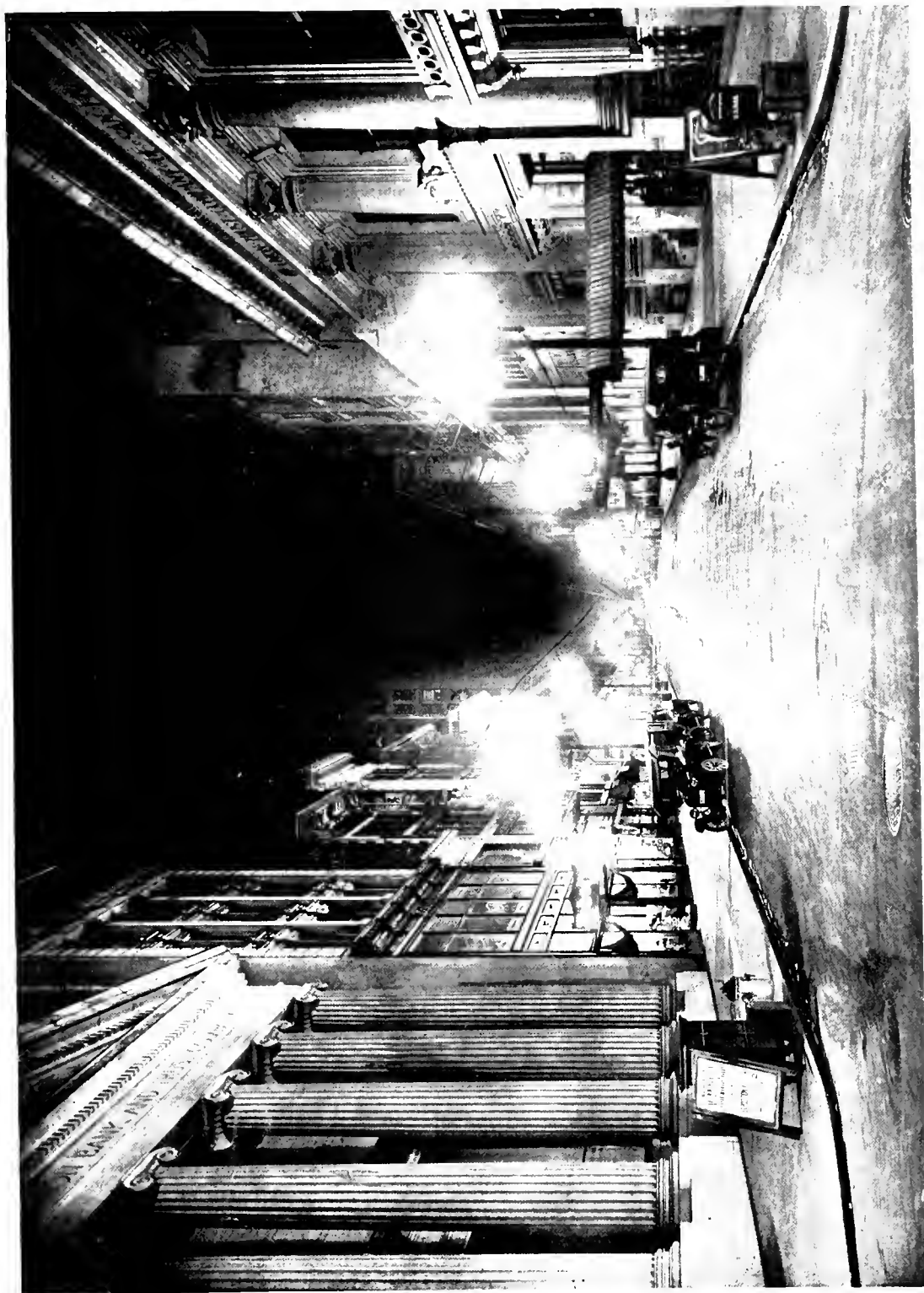
Fig. 7. Grant Avenue, Looking North, San Francisco, Cal., Intensively Lighted by 6.6-amp Ornamental Luminous Arc Lamps
