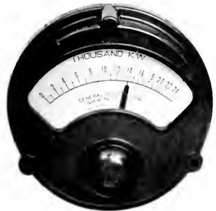
Fig. 4. Indicating Kilowatt Totalizer. Dispatcher's Office
