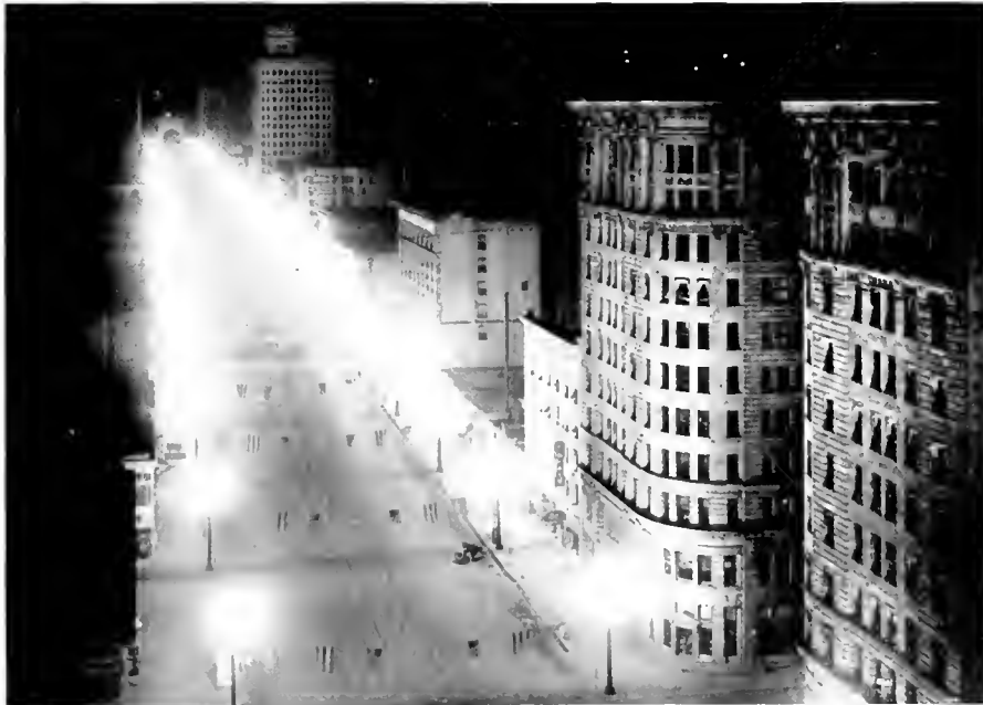
Fig. 12. Main Street, Salt Lake City, Utah, Intensively Lighted by Ornamental Luminous Arc Lamps
