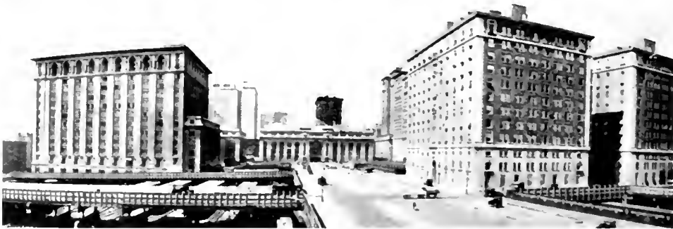
Fig. 5. General Views of Grand Central Terminal Area from 50th Street Before and After Electrification
