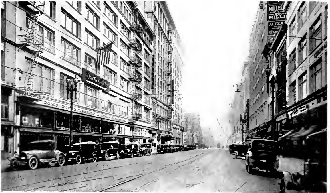
Fig. 8 Day View of Broadway, Los Angeles, Cal., showing 6.6 amp Ornamental Luminous Arc Lamps. The lamp units on the trolley suspensions were used for temporary lighting during the installation of the arc lamps. A night view is shown in the Frontispiece.
