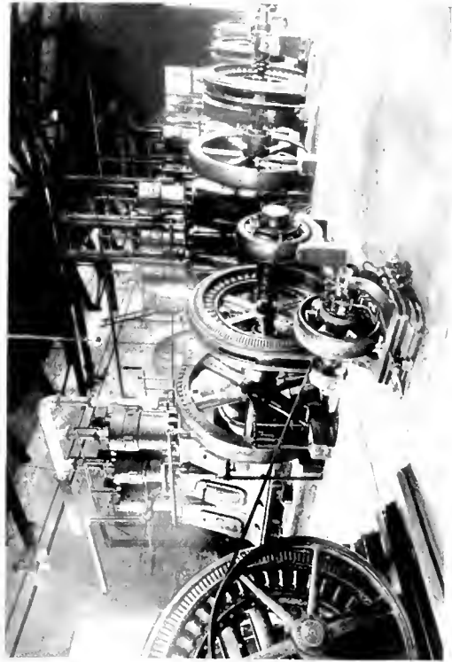
Fig. 2. Exciter Direct-connected to a 1250-kw., 3600-r.p.m., 2300-volt Curtis Steam Turbine Generator
