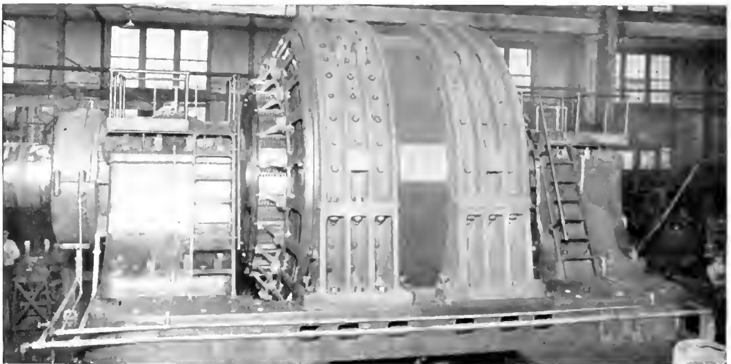
6300-h.p., 80 r.p.m., Direct-current Reversing Motor for Steel Mill Drive; 22,000-h.p. Momentary
