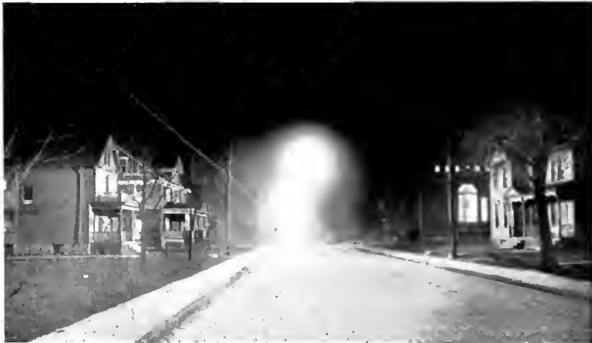
Fig. 12 Night View Showing Street Illuminated with Pendent Type Novalux Units Equipped with Refractors
