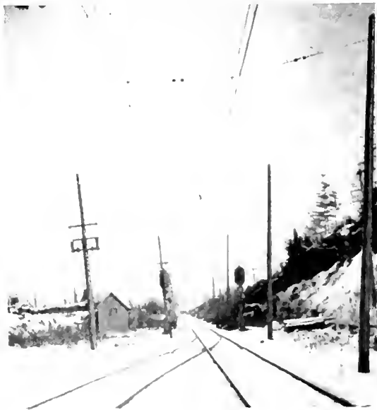
Fig. 13. Main Line, showing Overhead Construction Looking East from Cedar Falls Substation
