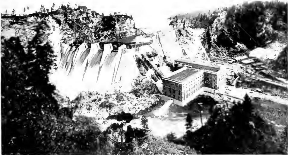
The Long Lake Station of the Washington Water Power Company located on the Spokane River, Washington. This system is interconnected with that of the Puget Sound Traction, Light & Power Company and furnishes energy to the Cascade Division of the C., M. & St. P. Rwy.
