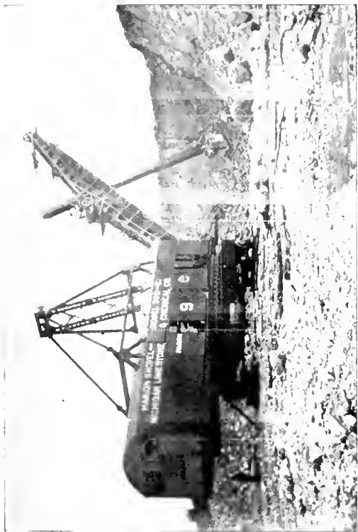
Fig. 2. Taking a 6 Cu. Yard Mouthful of Limestone
