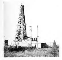
Fig. 4. This Well is being drilled by the Roxana Petroleum Co. with motor-operated cable tools, power being received from Gutbrie, Okla, over a 0<sup>3</sup>4-mile, 6600-volt transmission line which the Company built and operates to save the expense of hauling fuel for steam drilling
