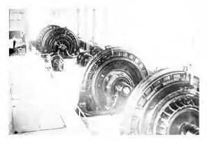
Fig. 2. In this Substation are four General Electric Synchronous Converters, each supplying 13,000 amperes at 525 volts for the electrolytic production of aluminum. A fifth unit has later been added, making the total expacity of this station 65,000 amperes
