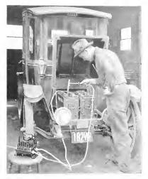
Fig. 4. Application of Pyrotip to the Repair of Vehicle Battery. The portability and general convenience of this device are valuable features for service of this sort
