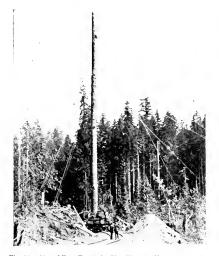
Fig. 34. Use of Tree Trunk for Handling the Yarder and Hoisting Cables for Hauling in Logs and Loading Them on Railroad Cars
