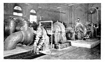
Fig 1. 1275-h.p. Curtis Turbine Direct-connected to Pumps for Municipal Water Supply
