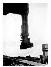
Fig. 38. Coal Trimmer at Bottom of Telescopic Chute, Showing Location of Operator's Cage
