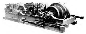
Four-drum Duplex Loading Machine for Logging Operations Snoqualmie Falls Lumber Company
