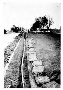
Fig. 8. Band Steel Armored Cable is generally recommended in places where no conduit exists as it can easily be laid in the ground without conduit as shown in this illustration
