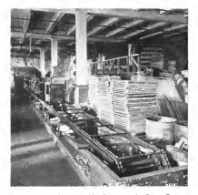
Fig. 1. Progressive Assembly Conveyors in Stove Factory. The stoves are handled entirely by conveyors during operations of assembly, enamelling, drying, crating and shipping to platform.
