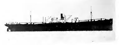
Fig. 4. S. S. Eclipse, the First Electrically Propelled Cargo Ship
