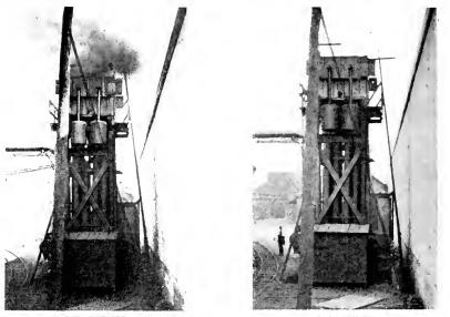
CURRENT OFF CURRENT ON Figs. 1 and 2. Comparison Showing the Effectiveness of an Electrical Percipitator in Eliminating Coal Smoke
