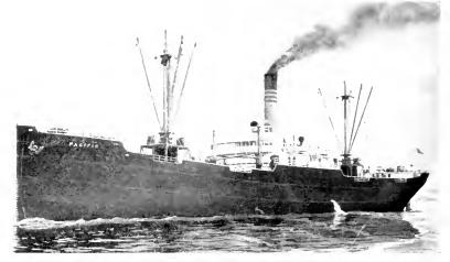
The Pacific is the first metchant ship in the world to be equipped with a high-speed turbine, double-reduction gear drive. The turbine is of the Curtis impulse type and the gears of the two-plane type. Up to October 1, 1920, this vessel has steamed over 230,000 miles
