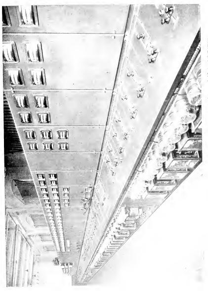
The 3-phase to 2-phase transformer circuits have time-limit overload relays, and also instantaneous differential protection across the transformers.
