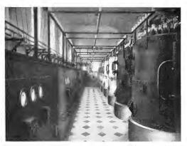
Fig. 3. A Battery of 2000-kw. Steam Boilers in Which the Water Itself Comprises the Heat Generating Resistance
