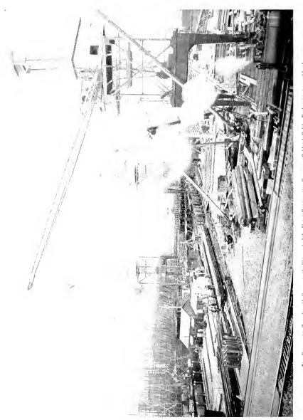
Five Four-motor Traveling.jib Cranes in the Shipyard of the Union Construction Company, Oakland, Calif. Each crane is capable of lifting 5200 fb. at a speed of 150 ft. par min. at a radius of 76 ft. or 15,000 fb. at a speed of 50 ft. par min. at a radius of 35 ft.
