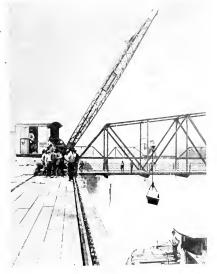
Fig. 4. Electric Locomotive Crane Handling Cargo at a River Terminal
