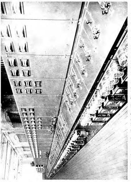
An Elaborate Instrument and Control Board for Cape Town, Africa Thit switchboard is more than 100 ft. long, and while it controls at present only 20,000 kw. provision is made to handle several times this capacity. It was completed late in 1920, and will be described in an early issue of the General Electric Retree
