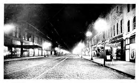
Fig. . State Store L. Joing South, Chicago, Id. Lighted by Novalax Stippled Glass Clubs Units Containing 1000 watt Multiple Mazda C Lamps
