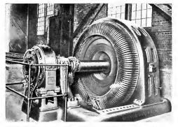
Fig. 5. 5000-kv-a., 600-r.p.m., 2300-volt Synchronous Condenser with Direct-connected Exciter, Trumbull Steel Co., Warren, Ohio
