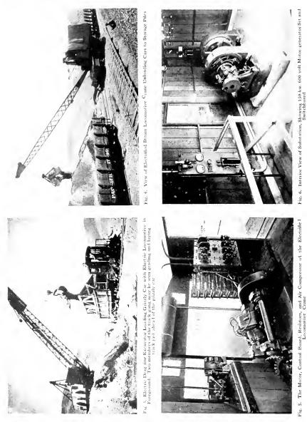
60-cycle 440-volt variable-speed type. This equipment has been in almost continuous service for seven years. Its radius of operation, and its flexibility in handling and loading material is very much greater than is possible with a shovel-type excavator.
