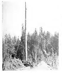
Use of Tree Trunk for Handling the Yarder and Hoisting Cables for Hauling in Logs and Loading Them on Railroad Cars
