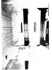
Fig. 5. A Typical Stateroom Lightung Installation Cne central ceiling fixture employing a round bib all-fixted. March B lamp and an adjustable reading lamp by the side of the berth. Enclosing glassware or fabric shades would have remarkably improved the installation.
