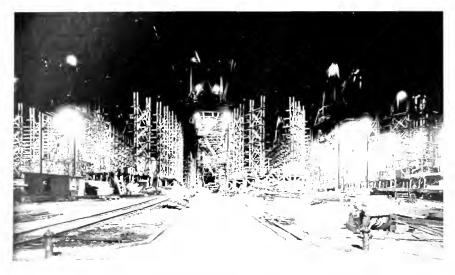
Fig. 11. Shipways Illuminated by Floodhghting Projectors and Novalux Units Hog Island Shipyard, Philadelphia Pa.
