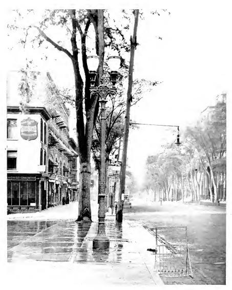
On Brochway South a Springs, Filtern 600 c p. Pen lant Type Fixtures Were Replaced by 70 Ornamental Standards, Each Having Two 1000 c p. Units – At the same time all ove lead wiling and unsightly poles were removed from the street
