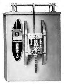
Fig. 73. Arrangement of Oil Circuit Breaker Mounted in Solid Concrete Cell
