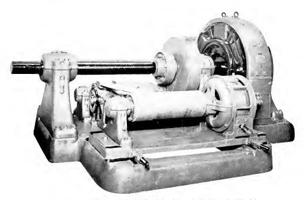
Fig. 4. One of the Motor Units for Sectionalized Drive of Newsprint Machine at the Mills of the Crown-Willamette Paper Company, West Linn, Oregon. Nine of these units are employed to drive the various sections of the paper machine
