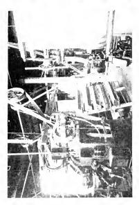
Fig. 22. BTS 55:b p. 1:90+r.pm. 550-volt Varging Speed Bruchshifting Motor isemi-automatic control) Drving a fix color Rice. Barton and False Cloth Printing Machine Imperial Printing and Finishing Co., Providence, R 1
