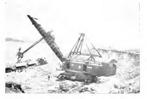
Fig. 1. 300-ton Electrically operated Shovel Loading Cars
