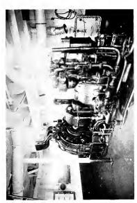
Fig. 6. The Dynamo Room on One of the United States Battleships. It is interesting to note the excellent diffusion produced by the white walls, ceiling and piping. Contrasty to what might be termed "standard practice" reflectors are employed in addition to the vapor proof enclosing globe.
