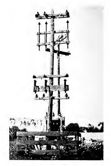
Fig. 9. Transformer, Lightning Arresters, etc., for 13,200 220-volt, 3-phase, 60-cycle Line
