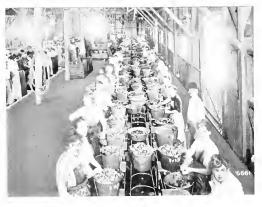
Fig. 4. Continuous Moving Conveyor in Canning Factory
