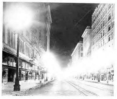
Fig. 1. Broadway, Los Angeles, Cal., Intensively Lighted by 6.6-amp. Luminous Arc Lamps
