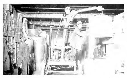
Battery Truck Crane Employed in Tiering Cases in the Plant of the Eastern Manufacturing Company, South Brewster Me
