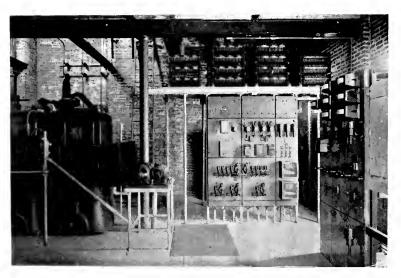
Interior of the Warrenville Automatic Substation of the A. E. & C. R. R., Showing Automatic Control Equipment
