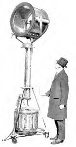
Fig. 5. High intensity Studio Light for one form of "hard" lighting
