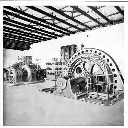
STEEL MILL INDUCTION MOTOR INSTALLATION WITH SCHERBIUS SYSTEM OF SPEED CONTROL. REGULATING SET ON LEFT; MAIN MOTOR ON RIGHT
