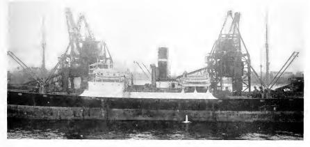
Fig. 5. General View Showing a Vessel with Two Mechanical Trimmers in Operation
