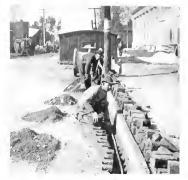
Fig. 3. Installation of Armored Cable in Brick Paved Street
