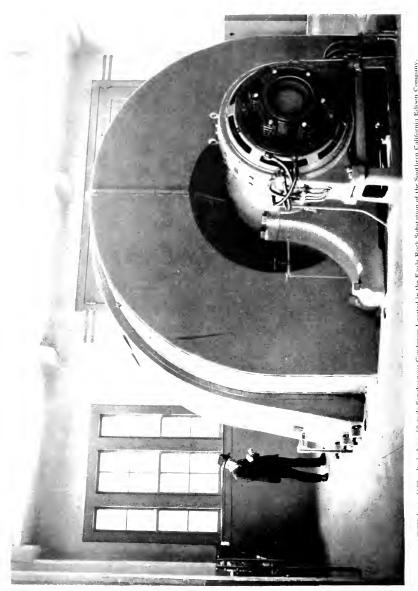
30.000 kv.a., 6000 volt, 3 plase, 50 cycle Synchronous Condenser Located in the Eagle Rock Substation of the Southern California Ediven Company. Two articles relative to the future operation of the transmission lines of this company at 220,000 volts uppear on pages 397 and 390 of this issue
