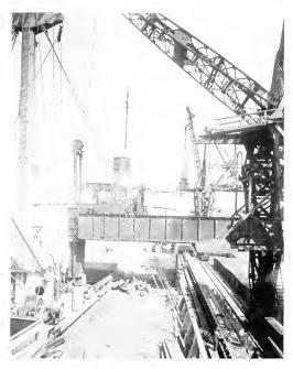
Fig. 1. Conveyor Tower and Ram with Coal Trimmer in Position to Operate
