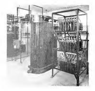
Fig. 4. 180-kv-a., 3-phase, 60-cycle, 6600-volt Static Condenser Equipment, Public Lighting Dept., Detroit, Mich.
