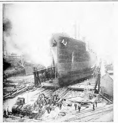
A Marine Railway Capable of Dry Docking a Vessel 500 Ft. Long, 76 Ft. Wide and 7500 Tons Actual Weight (13,000 Deadweight Tonnage) in Forty Minutes. (See article on page 240.) Nnety per cent of the vessels built under our emergency fleet wardine program come within the capacity of this dry dock
