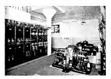
Fig. 1. Three 300-kw., 1200-r.p.m., 250-volt Synchronous Converters and Direct-current Switchboard, Bullard Engineering Works, Bridgeport, Conn.
