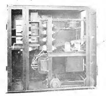
Fig. 67. Removable Truck Type Panel, 4600 Volts 400 Amperes, Showing Truck Partly Withdrawn
