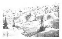
Fig. 1. Oil Wells Pumped by Electric Power in the Midway Oil Field, Calif.
