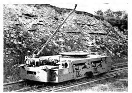
Fig. 1° New Type of Gathering Locomotive Showing Arrangement of Controller and the Use of Journal Leaf Springs
