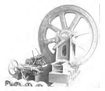
Fig. 6. Welding End Ring of Rotor, 36-pole, 1400-h.p. Induction Motor
