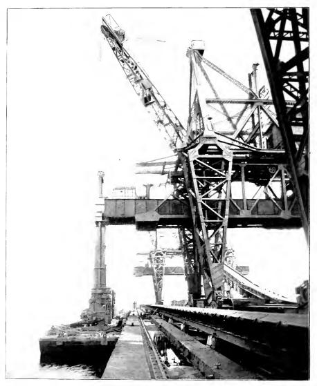
TRIMMING MACHINE LOCATED ON END OF COAL DELIVERING RAM OF BALTIMORE & OHIO COAL LOADING PIER. CURTIS BAY, M D See page 22
