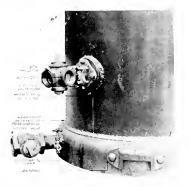
Fig 48. Standard Transformer Tank Showing Arrangement of Jack Boss and Drain Valves
