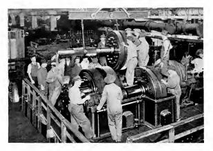
Fig 1. Class of Chief and First Assistant Marine Engineers at the General Electric Company's School Engaged in Assembling and Adjusting a 2500-h.p. Marine-geared Turbine
