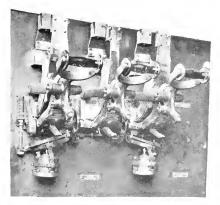
Fig. 69. Inverse Time Limit Overload Air Circuit Breaker, Shock-proof Type
