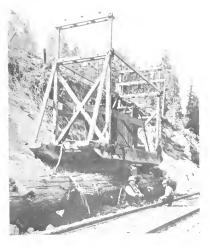
Arrangement of Outdoor Transfo:mer Equipment Showing Method of Mounting on Sled and Location Near Railroad Tracks
