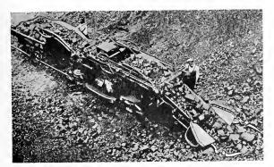
Fig. 37. Coal Loading Machine Showing Installation of Motor in Center and Complete Travel of Coal from Face to Mine Car
