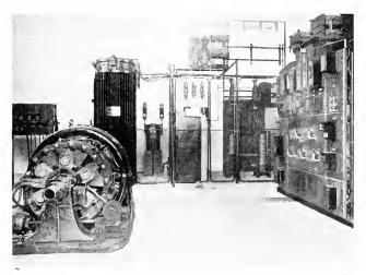
Fig. 4. 300-kw. Synchronous Converter Transformer and Control Gear, Cashmere Hills Substation
