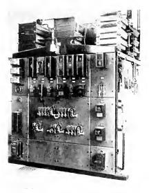
Fig. 2. Automatic Control Panel with Current Limiting Resistors on Top. (Time switch on righthand bottom sub-base panel)
