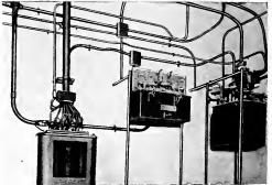
Fig. 6. Oil Immersed Line and Y-delta Contactors and Rotor Transformer for 150-h.p., 720-r.p.m., 2200-volt Brush-shifting Motor
