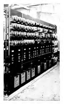
Fig. 6. Electrically Operated Switchboard for Controlling the Incoming Alternating-current Power
