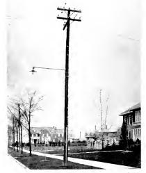
Fig. 1. Aerial Line Construction Showing Series Lamp Bracket Suspension
