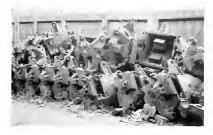
Fig. 4. Scrapped Cast Iron Motor Cases Being Reclaimed by General Electric Constant Energy Welding Machine
