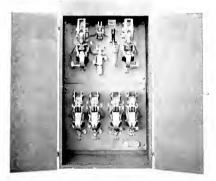
Fig. 5. Non-watertight Magnetic Controller, for Engine-room Auxiliaties, and Typical of Construction of Panels for Magnetic Control of Deck Machinery
