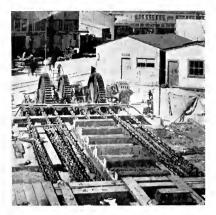
Fig. 5. A View Toward Shore from End of the Cradle, Showing the Electric Hoist and Chain Arrangement. The motor is of the slip-ring type and rated at 500 h.p. The liquid rheostat is covered by the canvas in the foreground
