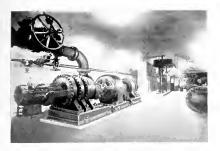
Fig. 5. 1050-h.p., 1200-r.p.m., 2200-volt Induction Motors Installed in a Pumping Station of an Iron Mine
