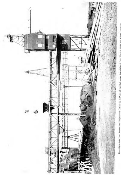
Mead Marrison Coal Tower and Lidgerwood Cableway at Plant of the Baltunore Consolidated Gas, Electric Light and Power Company. General Electric Alternating current Motors and Control Used. Bucket in Closed Position. Capacity, 350 Tons Per Hour
