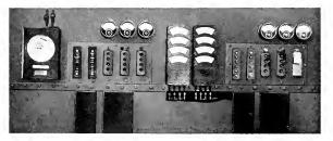
Fig. 10. Boiler Room Group Center Control of Auxiliaries for Two Boilers
