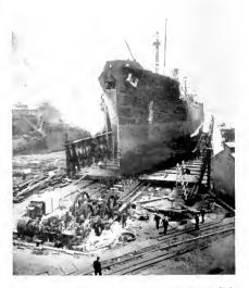
Fig 6. A View of the Orani, Showing Especially Well the Hoist and Chain Arrangement, as Well as the Cradle, Tracks, and Roller Trains The view was taken before the construction of the hoist house
