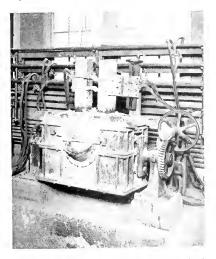
Fig. 4. Experimental Steel Furnace Built About 1907 by the Research Laboratory from Odd Parts. This furnace had a capacity of 600 lb, steel. Two 8 in square carbon electrodes were used, and power input amounted to as much as 200 kw with todia.cs up to 99 as higher cost, but the superiority of the automatic control is graphically illustrated by Fig. 2, which shows a wattmeter record
