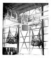
Fig 2 Monoral on Adjustable Loop Tracks Handling Miscellaneous Freight on Steamship Pier
