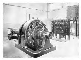
Fig 80. Automatic Railway Substation Equipped with Synchronous Converter and Automatic Control Equipment
