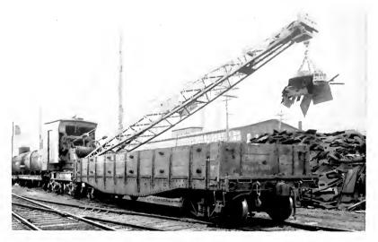
An Electro-magnetic Crane is Beyond Compare for Handling Scrap Boiler Plate and Structural Shapes Around Industrial Plants and Shipping Yards
