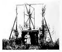
Fig. 4. Direction Finding Radio Station with Camouflage Protection as Employed for Military Purposes in France
