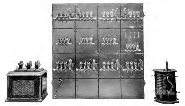
Fig. 6. Speed Control Equipment for Scherbius System
