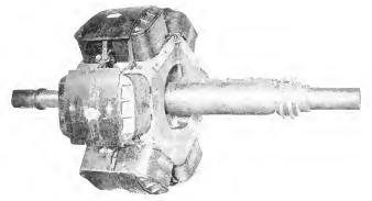
Fig. 7. Rotor of a 6-pole, 3530-kv-a., 500-r.p.m, Waterwheel Driven Alternator
