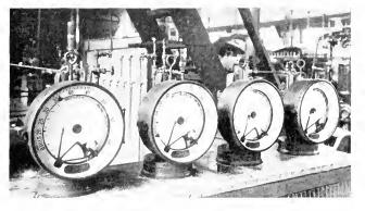
Fig. 4. General Electric Steam Flow Meters Installed in a Paper Mill
