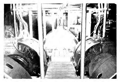
Fig. 3 Forward End of Engine Room looking forward , Showing Main Generators and Propeller Motor with Master Controlle: at Right
