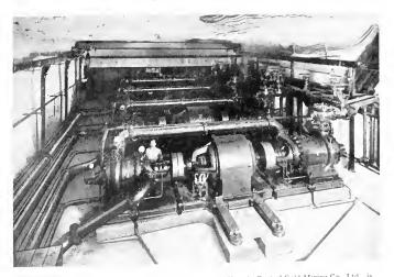
Fig. 1. The New Centralized Pumping Station of the Randfontein Central Gold Mining Co., Ltd. is Located in an Underground Chamber Cut in Solid Rock and Consists of Four Pumping Units Each Comprised of a Motor and Two Direct connected Pumps in Series
