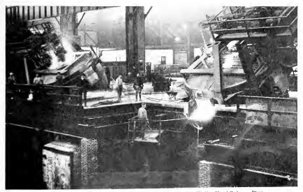
Fig. 1. The Two 40-ton F croult Electric Furnaces at the Charletton, W. Va., Naval Ordnance Plant. Furnaces are thown in tilted position immediately after pouring
