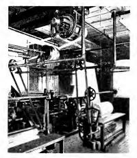
Fig. 19. BTS 10-h.p., 1200-r.p.m., 550-volt Brush Shifting Control, Varying Speed Motor Belted to Tenter Frame, Windsor Print Works, North Adams, Mass.
