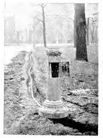
Fig. 4. Installation of Armored Cable for Park Lighting
