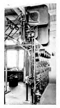
Fig. 7. 3000-volt, Direct-current Switchboard with Main Circuit Breakers Above
