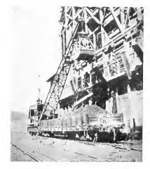
Fig. 8. Electric Locomotive Crane Moving Cars for Loading in Front of Washing Plant Chutes
