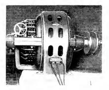
Fig. 17. BTS 100-h.p., 375-r.p.m., Three-phase, 440-volt Brush-shifting Motor Driving 100,000 Cu. Ft. Robinson Mine Fan at Aultman, Pa. This motor was installed in 1913
