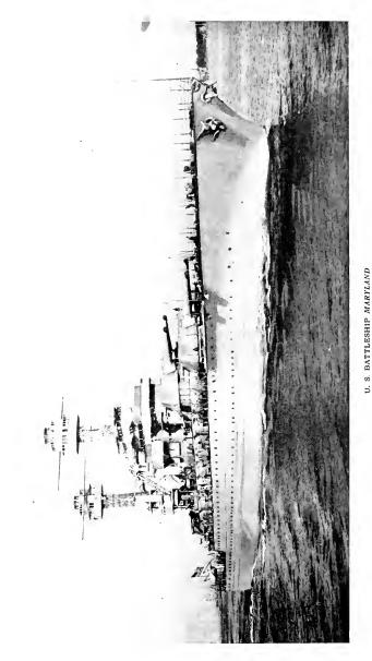
Main battery, eight 16-inch guns; displacement, 33,000 tons; speed, 21 knots; length, 624 ft.; beum, 971/2 ft. The Third "All-electric" Dreadnaught Completed for the U. S. Navy
