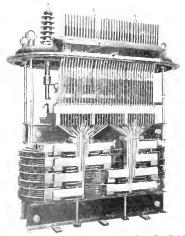
Fig. 10. High Capacity Transformer of the Type Supplied for the 40 ton Electric Furnace. Note the coil and core construction and the general sturdiness
