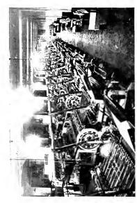
Fig. 88. Localized General High Intensity Lighting as Applied to a Modern Printing Plant. The white enamel finish of the machinery is worthy of special comment, introducing an element of diffusion in the illumination and eliminating sharp photos:
