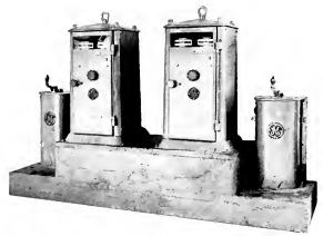
Fig. 3. Reel and Calendar Protective Panels and Controllers
