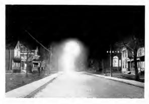
Fig. 8. A Street Intermediate Between a Business District and Highway Lighted by Novalux Mazda Lamp Units Equipped with Refractors
