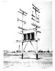
Fig. 3 A Typical Transformer Installation Made by the Empire Gas and Fuel Co. for O<sup>31</sup> Well Pumping in the El Dorado Field, Kansas The bank consists of three 25-kv-a, units, stepping the voltage down from 12,000 to 440.
