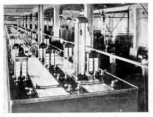
Fig. 3. Lock Control Board of the Panama Canal
