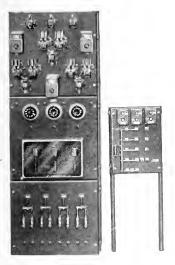
Fig. 9., General Electric Automatic Control Panel for Electric Furnace Electrodes. Operator's panel on right
