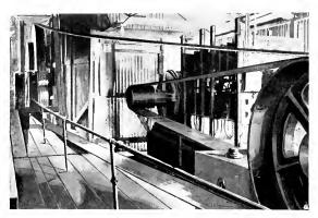
Fig. 29. 75-h.p., 720-r.p.m., 440-volt Induction Motor Operating Oil Well Drilling Equipment
