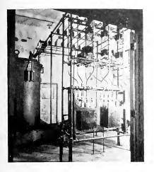
Fig. 8. One of the Transformers, with Its High-tension Switching Equipment, for the Forty-ton Steel Furnace
