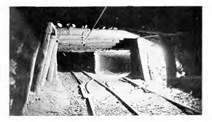
Fig. 90. The Switchpoint in a Coal Mine, with Suitable General Illumination. It is very interesting to contrast this picture with conditions as usually encountered in the mine. It is no wonder that the accident rate is relatively high considering the dangerous operating conditions and the total innadequacies of the lighting as ordinarily supplied
