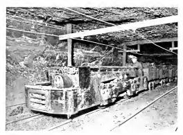
Fig. 18. 13-ton Haulage Locomotive of 1920 Type in Operation in Coal Mine
