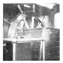
Fig. 6. Arrangement of Wheel and Master Controller in Pilot House
