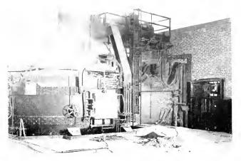
Fig. 3. Another View of 40-ton Furnace, Showing Control Panels on Right and Electrode Motors on Platform Above
