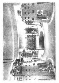
Fig. 20. Three BTS 180-bp - 380-rpm, and Three 100-bp - 400 rpm, 2200-volt Squarel Case Verical Motors with Push Button and Float Switch Control Severa Pumping Plant, Albany, N. Y.
