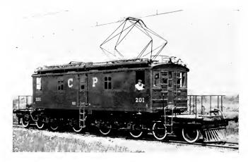
Fig. 3. One of the Four 120-ton Geared Passenger Locomotives
