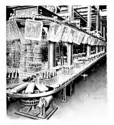
Fig. 1. Motor Driven Horizontal Staticnary Conveyors Lower conveyor of the slat type and upper of chain and hook type. Shows containers for adapting the product to conveyor handling. Empties returned on upper conveyor
