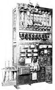
Fig 1. Typical Switchboard for the Control of the Apparatus and Circuits on an Electrically Propelled Vessel
