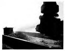
Fig. 39. Coal Trimmer Being Lowered Into Hold of Coal Boat, Showing Method of Depositing Coal from High-speed Belt Conveyor
