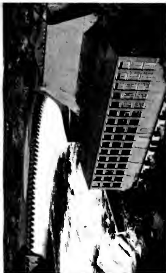
Fig. 5. Volta Plant of Great Falls Power Company, at Great Falls, 60,000 kw., 150-ft. head
