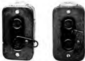
Fig. 6. Push-button Station for Starting and Stopping. The motors are equipped with remote control. A latch can be carried over the stop button and this latch held in place with a padlock. When this lock is in place the feed circuit is open and the equipment cannot be operated from this or any other station
