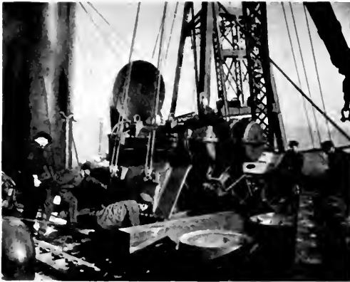
Fig. 9 Replacing a Set of One-plane Reduction Gears by the Two-plane Type in the Record Time of Ten Days
