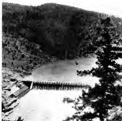
Fig. 1. Hauser Lake Development of the Montana Power Company, on Missouri River, 18,000 kw., 65-ft. head
