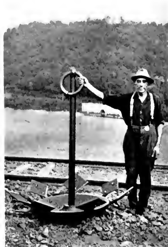
Fig. 6. A Modified Anchor for Holding Floating Equipment on Flashboard Work
