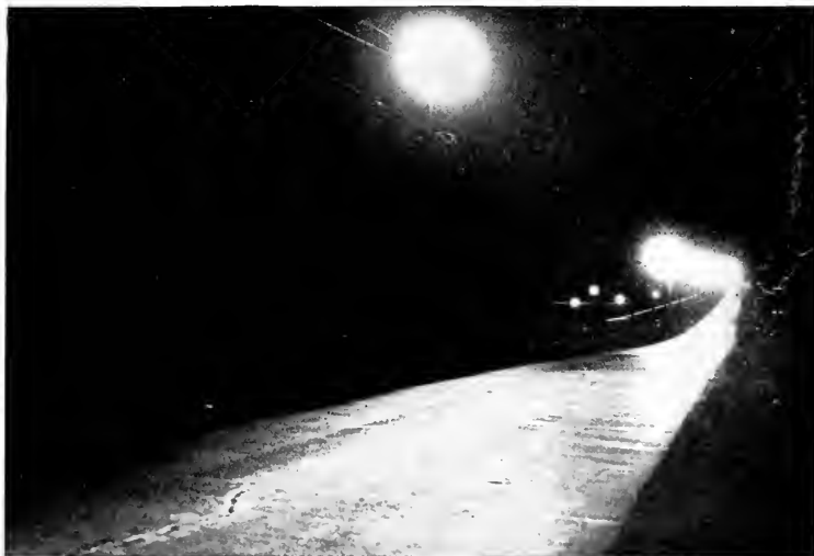
Fig. 82. A Typical Installation of Highway Lighting Units
