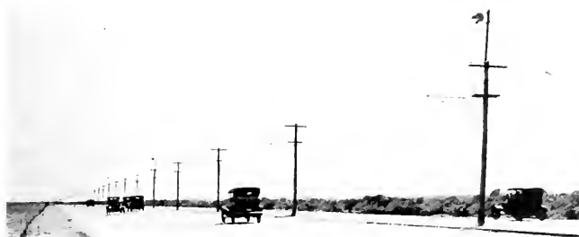
Fig. 5. Day View of Highway Lighting Installation, Miami Beach, Florida
