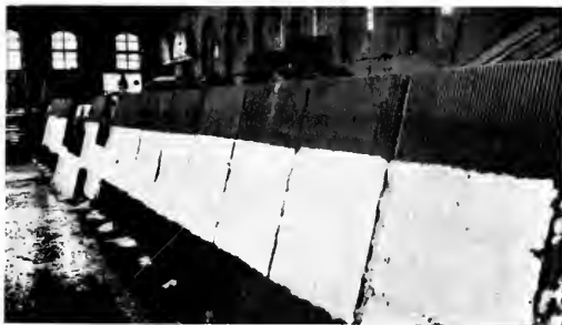
Fig. 6. Ten Years Ago This Plant Was Shut Down by Frazil Ice Obstructing the Screens and the Turbines. Today improved operating methods prevent any interference with consumers' service
