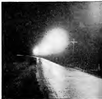
Fig. 7. Night View of Paradise Road, Swampscott, Mass., Illuminated by Novalux Highway Units Equipped with 2500-Lumen (250-c-p.) 6.6-amp. Mazda C Series Lamps
