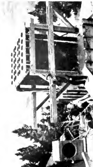
Fig. 7. Cottrell Precipitator Under Construction at a Commercial Size Copper Plant
