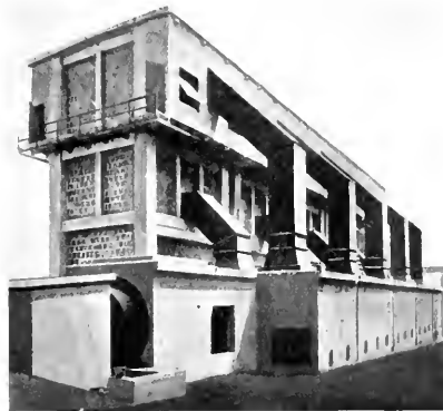
Fig. 1. Cottrell Precipitator Installation for Treating Cement Kiln Gas at the Dexter Portland Cement Company, Nazareth, Pa.
