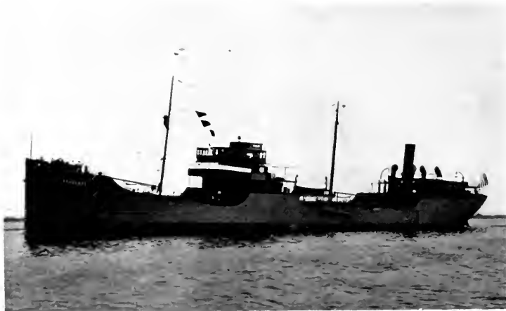
S. S. Bessemer, 7000-ton Tanker, Equipped with Electrically Driven Cargo Oil Pumps
