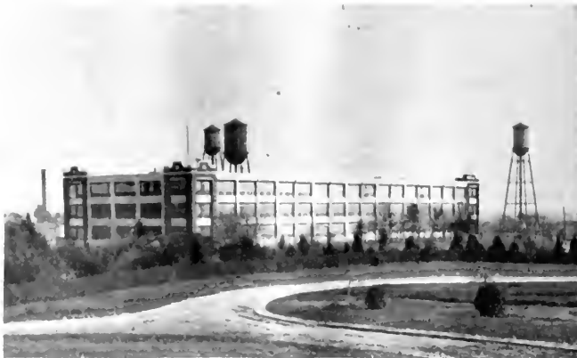
Fig. 1 Modern Cotton Mill Building. This mill, equipped with individual motor drives in picking, spinning and weaving departments, has been in operation since 1917
