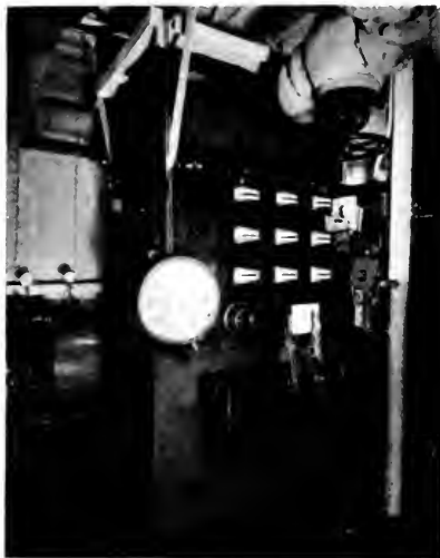
Fig. 2. The Maneuvering Platform of an Electrically Driven Vessel. The ship is held under perfect control by the two small levers near the bottom of the panel
