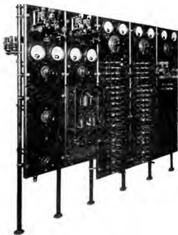
Fig. 9. Twenty-one-circuit Switchboard for Straight Constant-potential Charging
