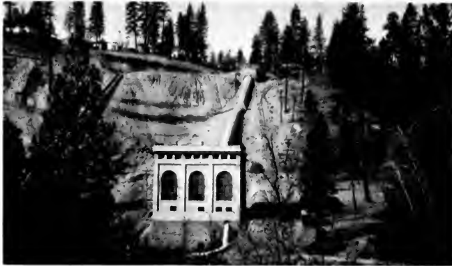
Fig. 1. Hat Creek Power Plant No. 2, Pacific Gas and Electric Company. This is a Stream Flow Plant, there being no dams or reservoirs in connection with the water supply. Installed capacity 12,500 kw-a.
