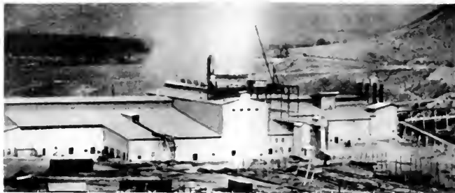
Fig. 2. Photograph Taken Before the Installation of Cottrell Precipitators at the Plant of the Riverside Portland Cement Company, California; compare with Fig. 3
