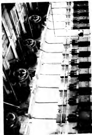
Fig. 3 Moderate Size Motors Connected to Shafts by Chain Drives. Each shaft drives 84 looms. There are 20 motors rated at 30 h.p. each in this row.
