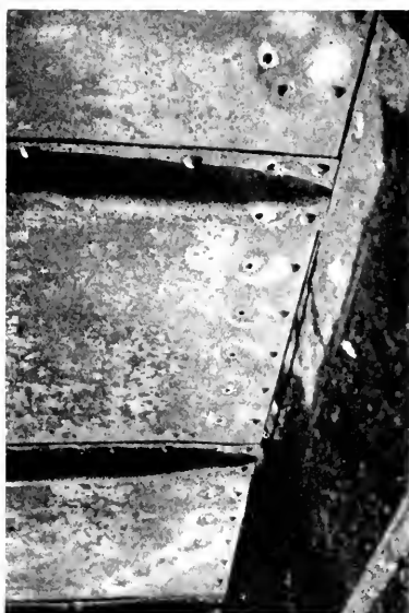
Fig. 4. After the Rivets are Backed. The rivet holes are not damaged by the arc
