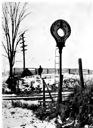
Fig. 78. Relay Operated Flashing Danger Signal at Railway Crossing
