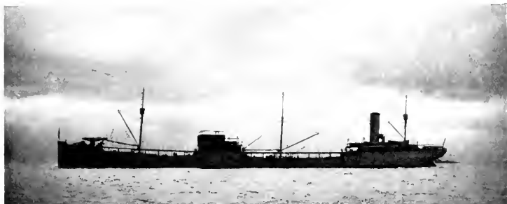
Fig. 4. Typical Tanker, Carrying Approximately 10,000 Tons of Oil. Twenty-four of these have been equipped with G-E Marine Geared Turbines
