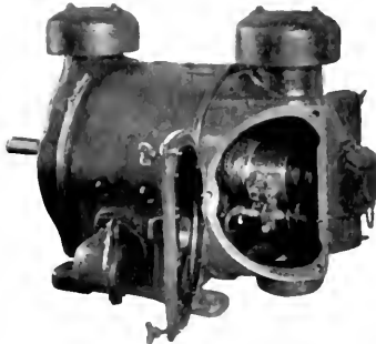
Fig. 6. 10-h.p., 1700-r.p.m. Enclosed Self-ventilated Marine Motor
