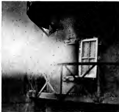
Fig. 5. Gas Issuing from Blast Furnace Precipitator When the Current is Off
