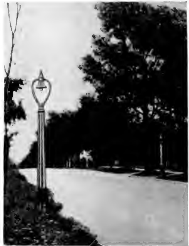
Fig. 81. Globeless Lighting Units Installed in Residential District of Rochester, N. Y.
