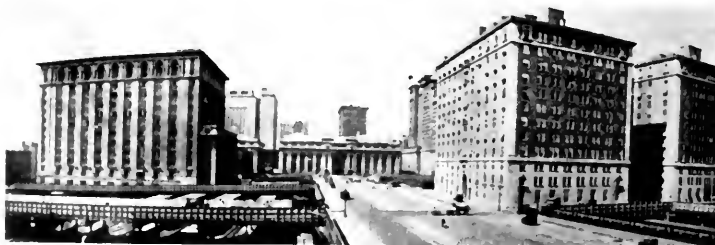
"General Views of Grand Central Terminal Area from 50th Street Before and After Electrification"
