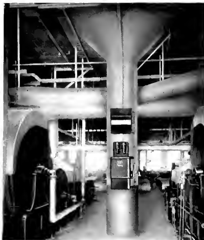
Fig. 11. Arrangement of Compensator with Relays for Slasher Group Drive Control
