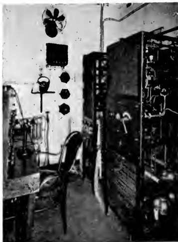
Fig. 3. Installation of Duplex Radio Apparatus on Board the S. S. America
