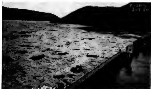
Fig. 4 Cake Ice Does Not Ordinarily Affect Hydro Plant Operation. This illustration shows how an arch wall prevents the ice from getting into the forebay.
