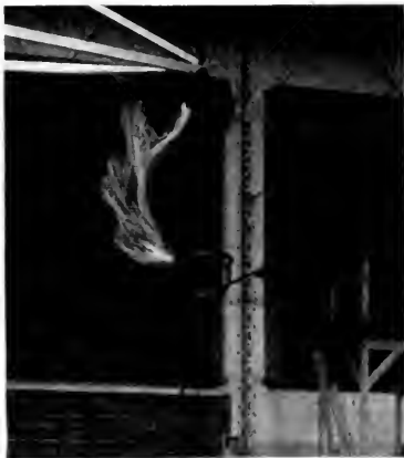
Fig. 37. Shield for Equalization of Voltage on Insulators Showing Dry 60-cycle Arc-over on a Shielded String
