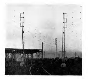
Fig. 2. Split Conductor Transmission Line, Victorian Railways. Each circuit is composed of six  $\frac{7}{16}$ -in. copper conductors
