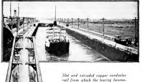
rail from which the lowing locamotices of the Panama Conal pick up electric current. Copper rails supplied by The American Brass Company.
