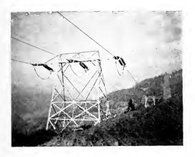
Fig. 9. Anchor Tower on 220,000-volt Big Creek Line of the Southern California Edison Company
