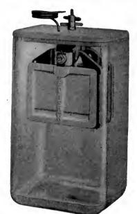
Fig. 9. Five-hundred Ampere-hour Edison Primary Battery
