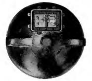
Fig. 6. 50-kv-a. Transformer Equipped with Network Protector View of Cover and Fuse Board
