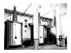
Fig. 4. Three 8333-ky-a. 220,000-volt Transformers Installed in Big Creek No. 8 Hydro-electric Station
