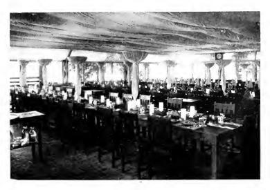
Fig. 80. Lighting pedestals which project slowly moving bands of blended color on the ceiling by means of a motor rheostat device
