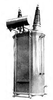
Fig. 13. Large Water-cooled Transformer with Conservator Tank
