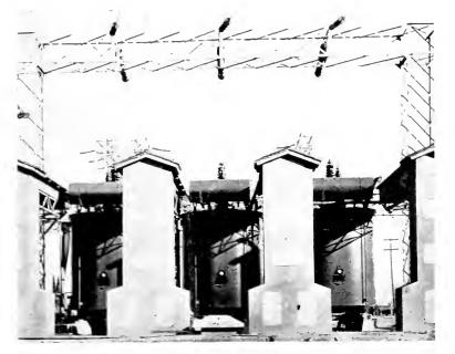
Fig. 3. Installation of Conservator-Type Transformers at the Vacaville Substation of the Pacific Gas & Electric Co. Single-phase Auto Transformers of 16,667-kv-a output to transform from 200,000 to 100,000 volts
