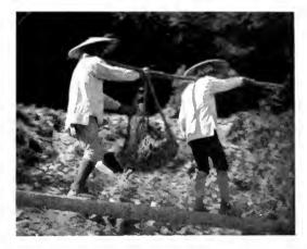
Fig. 5. Method of Excavating by Means of Rope Baskets
