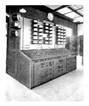
Fig. 11. Front View of Main Control Switchboard
