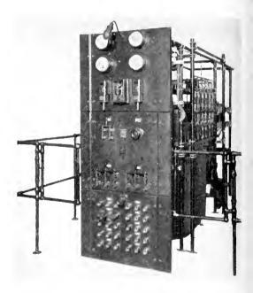
Fig. 2. Front View of the Rectifier showing Panel and Controls
