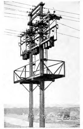
Fig. 41. Three Manually Operated Oil Circuit Breakers Installed on Transmission Line
