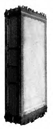
Fig. 1. A Cooler Section 9 Tubes Wide and 24 Tubes Deep. The more usual section will be 20 tubes wide and 12 to 18 tubes deep
