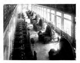
Fig. 1. Seven 3000-kw. Synchronous Converters in the Substation of the Electrolytic Zinc Company of Australasia
