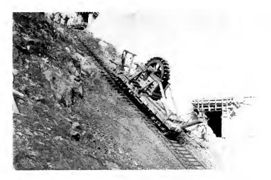
Fig. 3. Lowering 28-ton Generator Rotor to Power House, Jan. 8, 1923
