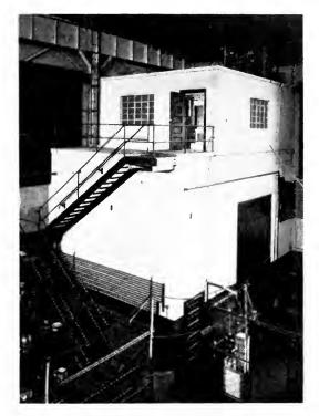
Fig. 5. Small Dark Room with Office Above. This dark room is equipped for tests up to 300 ky, to ground
