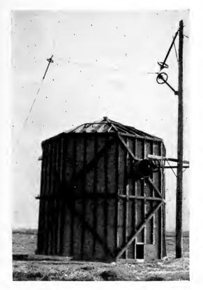
Fig. 4. Coil Similar to That of Fig. 3, but Housed in a Frame Structure Lined with Copper
