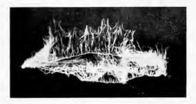
Fig. 21. Another 1,000,000-volt, 9-ft. Three-phase Arc showing Both Y and Delta Formations
