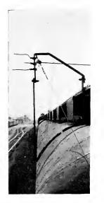
Fig. 48. Antenna Construction on Pullman train for radio reception en route
