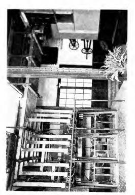
Fig. 3. Arrangement of Main Busbars between Generator and Switchboard
