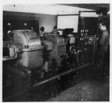
BEARING RESEARCH—speeds to 30,000 rpm and loads to 65 tons are studied
