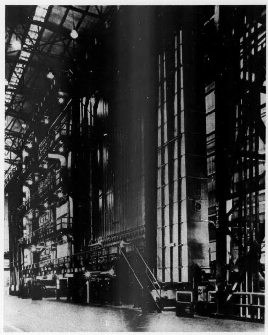
WORLD'S LARGEST annealing furnace continuously anneals tinplate at a maximum strip speed of 1000 feet per minute
