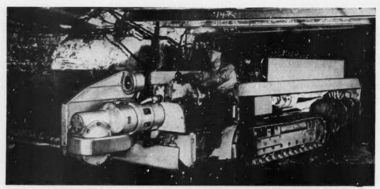
MINE SHUTTLE CAR carries coal from the working face to the main haulage way. It has a capacity of 190 cubic feet
