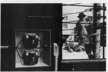
inate the problem of oil contamination that is always present with oil interrupters. The solenoid operating mechanism included in the new design fulfills the demand for a breaker with long mechanical life under the stress of continuous repetitive service.
