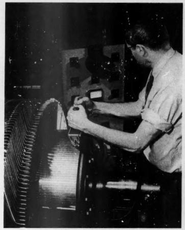
INSULATION of large rotor is checked with this winding-insulation tester
