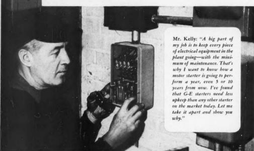
Martin Kelly, Plant Electrician for John R. Evans & Co., changes an overload relay on G-E combination starter quickly and easily,
