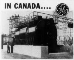
One of two Synchronous Condensers, Outdoor type hydragen-cooled, ruled 48,000 kvs, 13,800 volts, 720 rpm, built at Peterborough Works, of Canadian General Electric Co Ltd and instelled at a large transformer station of the H. E. P. C. of Onterlo.
