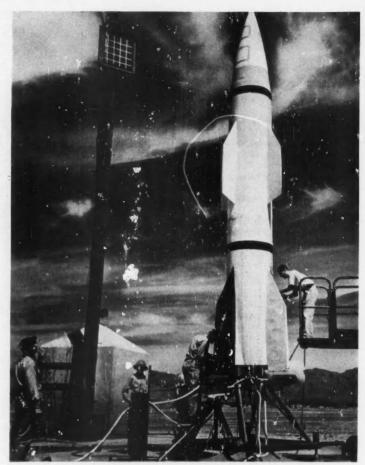
HERMES A-1 MISSILE on the firing stand at the White Sands Proving Ground. This rocket was one of a series launched to gain valuable data for future designs
