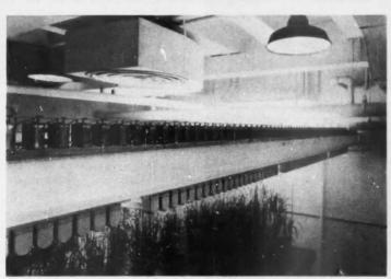
UNDERGROUND GREENHOUSE of the U.S. Department of Agriculture's greenhouse at Beltsville, Md., where the fluorescent lighting system operates on 360 cycles
