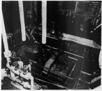
SINGLE-CYLINDER geared-turbine propulsion unit on the Great Lakes ore carrier Homer D. Williams replaced a reciprocating steam engine, thereby increasing its speed
