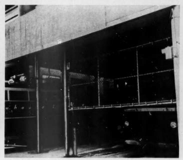
BUS-GATE SPOTLIGHTS in Detroit concentrate powerful 100,000-candlepower beam on electric eye that controls the opening and closing of two gates
