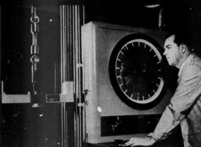
TENSILE TEST puts sample of new silicone adhesive under 900 pounds pull. Under greater tension, the rubber breaks before the bond that links it to the steel caps
