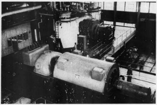
MERCURY-STEAM CYCLE proved its high thermal efficiency at the Schiller Station of the Public Service Co. of New Hampshire
