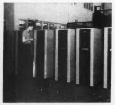
INDUCTROLS ARE AVAILABLE for both manual and automatic operation, and both single- and three-phase circuits. Singlephase units are being prepared here for final twit prior to shipment. Standard automatic regulators range in size from 3 kva, 120 volts up to 500 kva, 600 volts.
