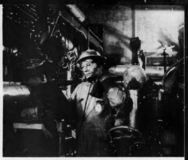
CLOSE-UP OF EXPERIMENTAL liquid-sodium heat-transfer apparatus being used in the development of a submarine intermediate reactor.
