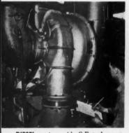
**DIESEL** engine, with G-E turbosupercharger, weighs 18 lbs per horsepower as agains 35 lbs without. On railroad locomotives, this diesel supercharger also improves operation at high altitudes.
