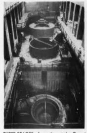
THREE STAGES of erection at the Grand Coulee pumping plant. From front to back can be seen a scroll case before motor foundation has been poured; a motor stator frame; a completed motor
