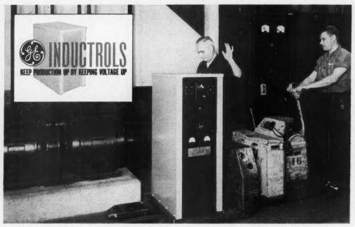
GENERAL ELECTRIC INDUCTROLS maintain correct voltage on electrical equipment, guard against the bad effects of poor voltage. Here a new threephase inductrol is being installed in a large industrial plant.
