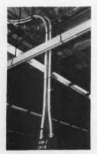
NO THREADING, NO PRE-BENDING on this run of two 500 MCM cables. Threadless fittings terminate cable at panel box. Two right-angle bends made with no fitting, no bending equipment.
