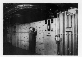
**FROM WAREHOUSE TO TANK PLANT** in less than a year. That's the latest record of this midwest tank plant. This 53-acre tank plant increased power distribution with two 7500-kva transformers and eighteen 1500 kva load centers. For fast installation G-E interlocked armor cable was the choice.
