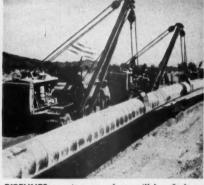
**PIPELINES** carrying natural gas will benefit from hooster pumps driven by General Electric gas turbines which burn gas "bled" directly off the main line. Because it needs no water, the G-E gas turbine is well suited for operation throughout desert areas.
