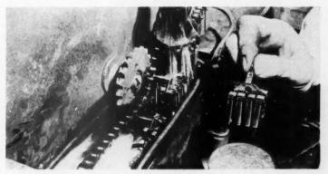
SPECIALIZED DEVICE for cleaning operation (shown in the accompanying diagram) includes handling equipment for the shaver heads and the means of providing freshly distilled cleaning solution
