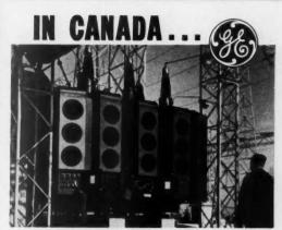
Canada's largest — a 120,000 Kva autotransformar installed in Southern Ontoria one of ten built by Canadian General Electric at its Davenpert Works, Teronto.
