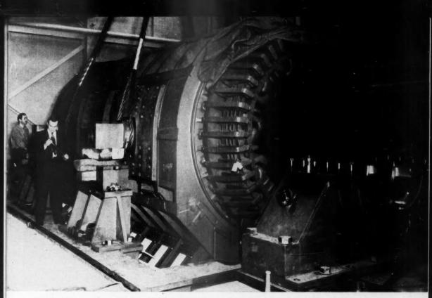
REINFORCED END WINDINGS AND UNIQUE SUPPORTING STRUCTURE CHARACTERIZE THE WORLD'S LARGEST SHORT-CIRCUIT GENERATORS
