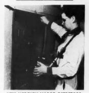
NEW MERCURY VAPOR DETECTORS Users of mercury compounds can now determine harmful concentrations of mercury vapor with the new, completely redesigned G-E Mercury Vapor Detectors. Electronic and chemical detectors provide either instantaneous or continuous indication. Electronic detector pictured being used to check curing oven in laboratory of silicone rubber plant. See bulletin GEC-312\*.
