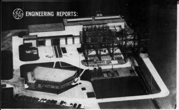
NEW ENGINEERING LABORATORY—making possible comprehensive tests on a scale never before possible—enables G-E engineers to make faster, more searching studies, clip months off major switchgear developments. Designed to keep pace with industry's increasing use of electric power, it has ten times the capacity of America's first such installation, built by G.E. in 1921.
