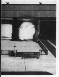
**FLASH** in one of five test cells results from deliberately testing a circuit breaker to destruction. Board at right indicates conditions of the test.
