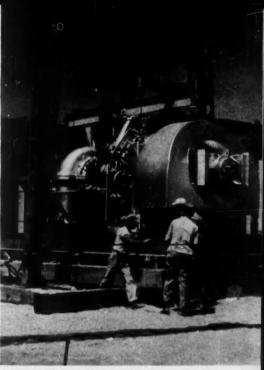
SUPERVISION OF INSTALLATION by G-E service engineers assures proper start-up of this gas turbine—one of 28 units for gas-pipeline pumping in the Southwest.
