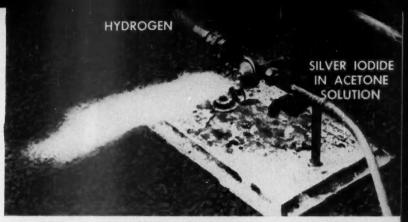
SILVER-IODIDE SMOKE GENERATOR DEVELOPED BY VONNEGUT FOR USE ON THE GROUND
