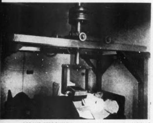
**REGAUD-FERROUX** This early French design used a thick lead container to shield a radium source of four grams
