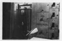
LOAD-CENTER UNITS are installed in secondaryselective system for greatest reliability.
