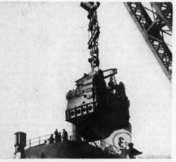
**KEEP 'EM SAILING** service cuts idle port time with day-and-night work on emergency repairs. Ships keep closer schedules, boost earnings. Here, a propulsion gear is being installed in a modern tanker.
