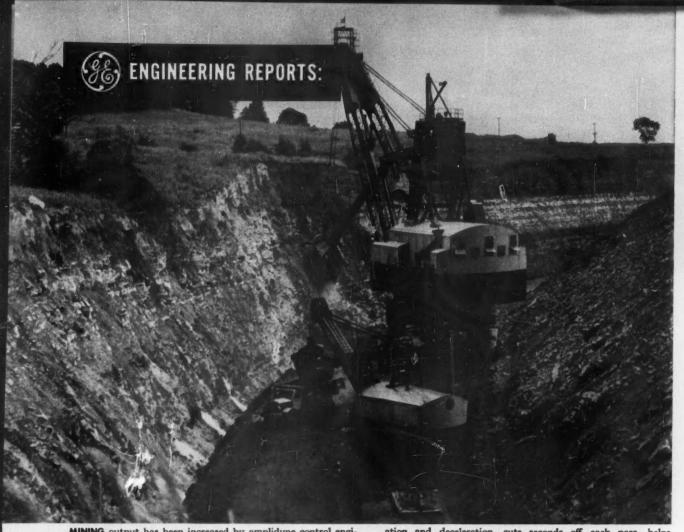
MINING output has been increased by amplidyne control engineered into electric shovels and mine hoists, including giant strippers like this. Instant shovel response, plus faster acceleration and deceleration, cuts seconds off each pass, helps increase the daily yardage handled. At all speeds, electrical and mechanical components of your equipment are better protected.
