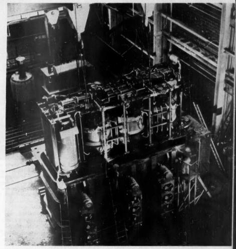
TANKING CORE AND COILS of largest autotransformer built by General Electric. It has a rated output of 156,000 kva and transforms voltages from 230 to 138 kv
