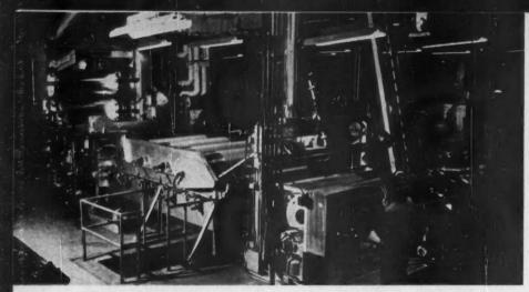
PLASTIC FILM calender train is driven by several d-c motors. Speed of the motors can be adjusted within wide limits, but once adjusted, motors remain in step
