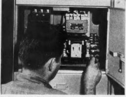
**EASY TO WIRE.** Four-inch wiring trough; components accessible from all sides; front-connected starters; doors swing more than 90°.
