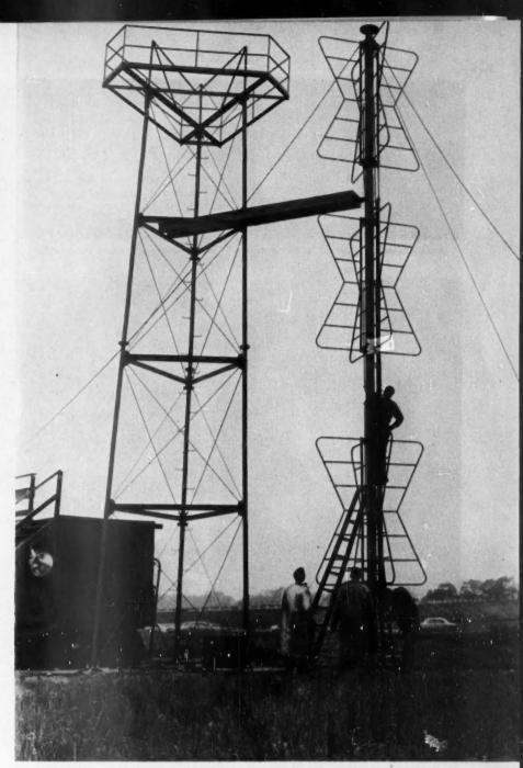
THREE-BAY TV ANTENNA FOR STATION KPIX UNDERGOES A FIELD-TEST OPERATION
