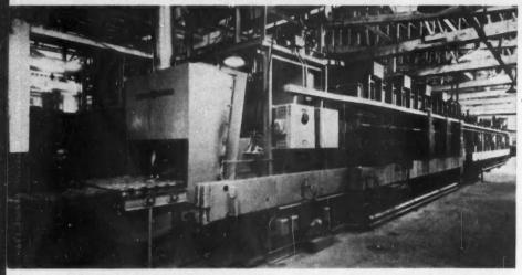
**ELECTRICALLY HEATED** roller-hearth furnaces are designed to anneal from 5500 to 13,750 pounds of steel cartridge cases per hour at 1250 F
