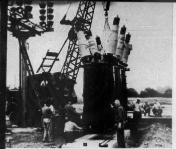
BASE-MOUNTED outdoor power circuit breaker is conveniently transported to its site and installed as a complete unit
