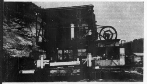
**REMOTE-CONTROLLED** coal digger developed for Carbide and Carbon Chemicals Company bores 700 feet into coal seam with 30-foot conveyor belt sections
