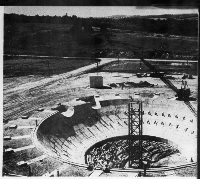
CONCRETE SAUCER IS THE FOUNDATION FOR A 225-FOOT STEEL SPHERE, LARGEST EVER CONSTRUCTED, THAT WILL HOUSE AN ATOMIC POWER
