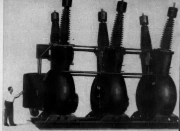
STEEL-CLAD impulse-type circuit breaker rated 10,000 mva contain only about half the oil of similar round tank breakers
