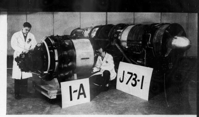
TEN-YEAR SPREAD-LATEST J-73 TURBOJET DELIVERS MANY TIMES THE THRUST OF THE I-A BUILT BY GENERAL ELECTRIC IN 1942
