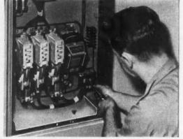
**EASY TO SERVICE.** Units are easily disconnected from bus and locked in test position (above). Barriers between units are easily removed to facilitate wiring (below).
