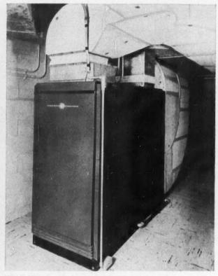
**HEAT PUMP** advantages for the home include fully automatic heating and cooling in one package, no fuel or chimney requirements, and uniform year-round temperature
