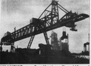
**ORE-HANDLING**, as well as blooming, rolling, pickling and other steel-mill operations, uses the G-E amplidyne. Ore bridge drives provide more accurate bucket control, fast trolley travel.
