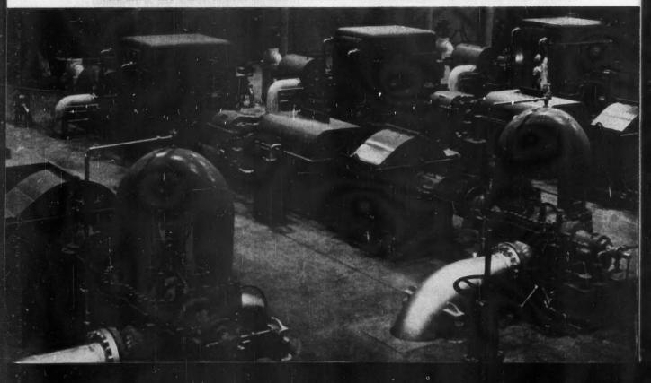
PURE HIGH-PRESSURE REACTOR COOLING WATER IS PROVIDED BY THIS PUMPING EQUIPMENT AT THE HANFORD WORKS
