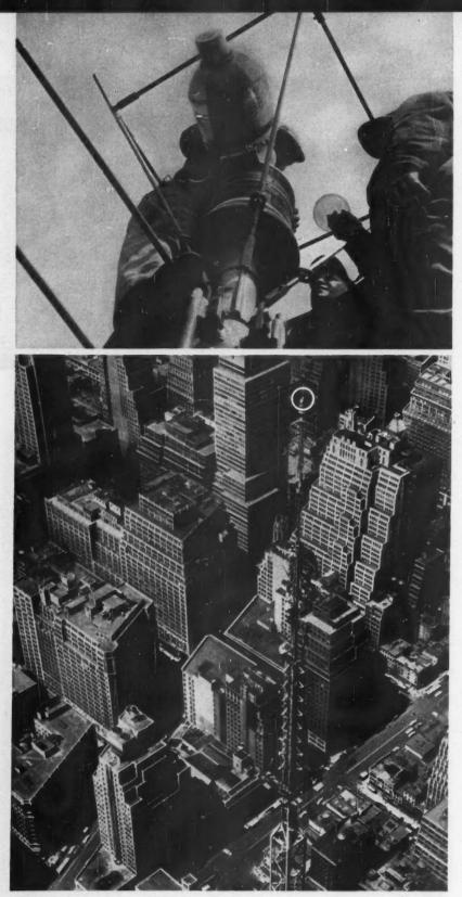
HARD GLASS LAMPS installed in red beacon unit atop Empire State Building's TV antenna (top) are heat and shock resistant. Aviation beacon (circled) must withstand bad weather. Ordinary lamps were replaced after hard storms
