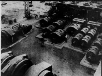
WORLD'S FASTEST cold-strip mill has five tandem stands and a winding reel (not shown) individually driven by d-c motors
