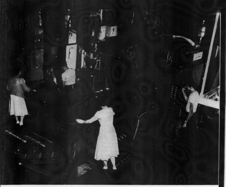
EIGHT-HOUR PRODUCTION OF WIRE REFRIGERATOR CONDENSERS BY THIS AUTOMATIC MACHINE REQUIRES NEARLY 150 MILES OF WIRE
