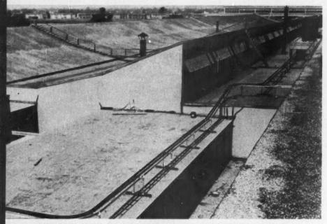
INTERLOCKED ARMOR CABLE IS CARRIED OVER ROOF ON LIGHTWEIGHT CABLE RACKS
