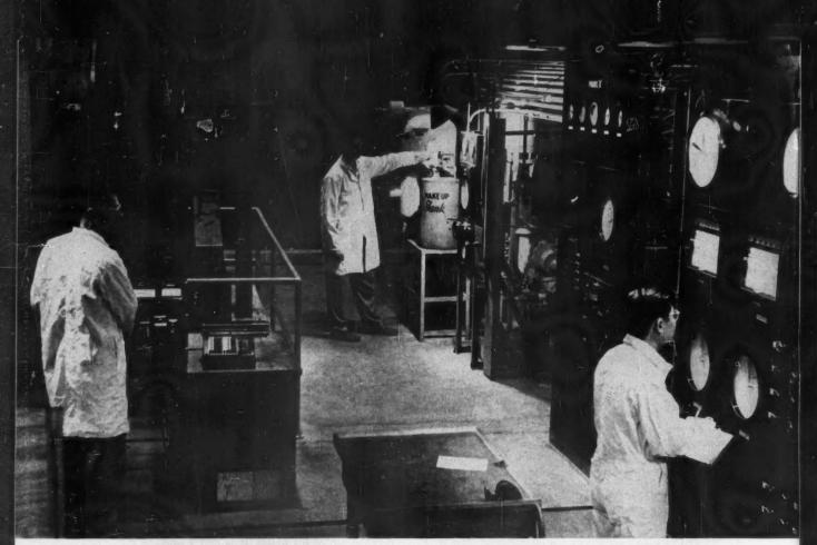
HEAT COMPARABLE TO THAT ENCOUNTERED IN A NUCLEAR REACTOR IS PRODUCED AND DISSIPATED IN THIS INSTALLATION
