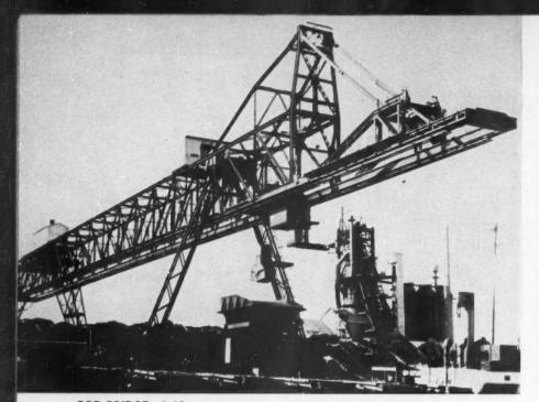
ORE BRIDGE of 12-ton capacity is equipped with adjustable voltage d-c drives and is supplied with a-c power. Ore from boat is being unloaded into hopper
