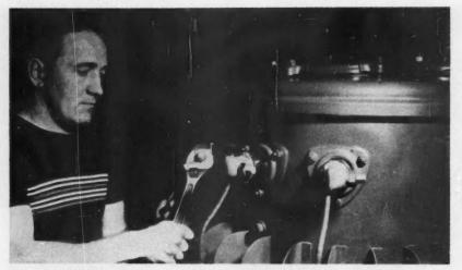
TERMINALS OF NEW ALLOY RESIST FAILURE IN CORROSIVE ATMOSPHERE
