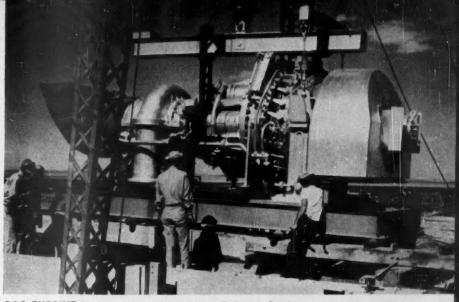
GAS TURBINE in the process of being installed in a Southwest compressor station will pump natural gas to industrial centers throughout the country
