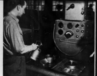
2 Operator sprays the propeller pattern with a special siliconeemulsion parting agent at the ejection station, after heating it to an operating temperature of 500 F. Transfer of pattern between oven—partially obscured at left—and ejection station is automatic. The purpose of this step is to facilitate later removal of the finished shell mold from the pattern. Next. . .
