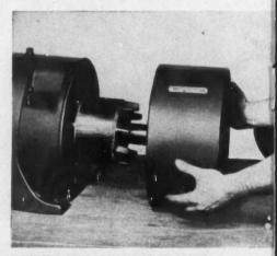
NOW THE STATOR MAY BE REMOVED. Entire job takes only minutes. This is only one of many features designed to cut "down time" up to 50 per cent.
