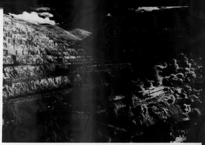
MOUNTAIN OF COPPER ORE, BINGHAM CANYON, UTAH-REMOVAL OF 135,000 TONS OF ROCK PRODUCES 92,000 TONS OF DRE DAILY.
