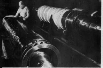
FIG. 10. PRECISION balanced generator rotor—after assembly in turbine-generator it is test-run to check for further unbalance.
