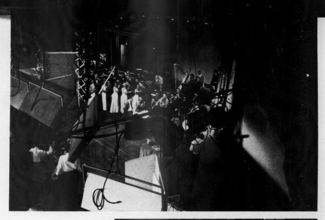
**MODERN TV LIGHTING** offers flexibility and efficiency. Contrast the highlights on hair and shoulders of performers in the Fred Waring program (*above*) with the lighting of an early installation at WRGB, Scheneetady (*right*). Overhead lighting with fluorescent lamp banks and Fresnel lens spotlights combine to effectively provide base, back, and key lighting, replacing water-cooled mercury lamps.
