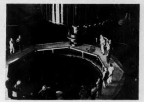
MORE AUTOMATIC VOLTAGE CONTROL. G-E engineers applied amplistats in the voltage regulator system for this giant alternator, being positioned at a hydro-electric installation.
