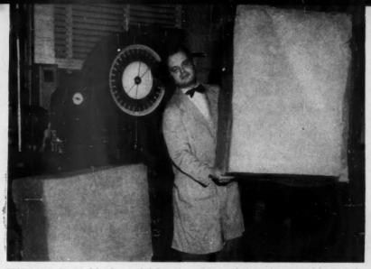
**TWO-FOOT THICK** slab of expanded foam is easily moved about the testing laboratory by author. Density of the slab, however, is what determines its mechanical properties.
