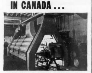
97.5 kw. infra-red oven drying finish coat on complete tractor assemblies,
