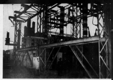
**INCOMING LINE SIDE** of 6.9-kv package substation that supplies power to large motors. Visible in upper foreground are incoming line terminations. Incoming line's circuit breakers and the substation building are in background. Note in one-line diagram (below) that the 66-kv circuit breakers feed stepdown transformers connected to the indoor switchgear.
