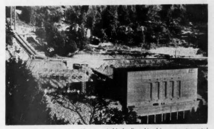
HYDROELECTRIC power station with two vertical hydraulic-turbine-driven generators rated 37,500 kva at 180 rpm. Here, engineers will concentrate on improvements in generator design.
