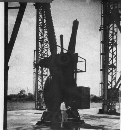
LARGEST circuit-breaker is rated 25-million kva. But will it be large by tomorrow's standards? Present concepts of circuit-breaker design are almost sure to be inadequate.
